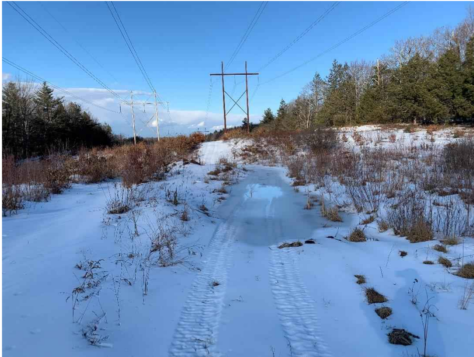
Photograph No. 4: Looking northerly at proposed access associated with Wetland CHW-14 towards 391 Structure 297 (right) and 373 Structure 300 (left). Timber matting will be used in the wetland portion of the access route.
