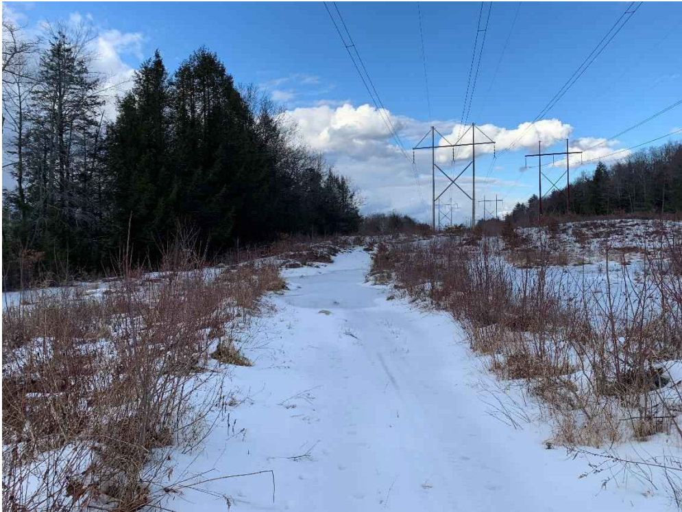
Photograph No. 6: Looking northerly at proposed access route associated with Wetland CHW-12 towards 373 Structure 299 to be replaced. Timber matting will be used in the wetland portion of the access route.
