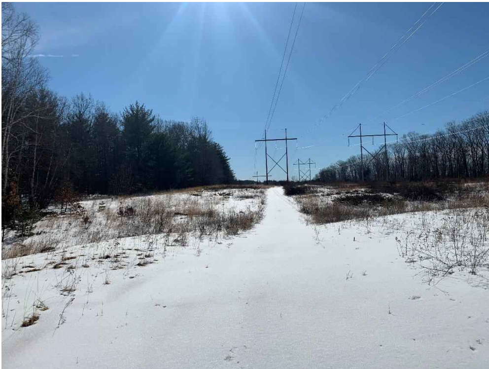
Photograph No. 12: Looking southerly at proposed access route towards 391 Structure 292 (left) and 373 Structure 295 (right) to be replaced.
