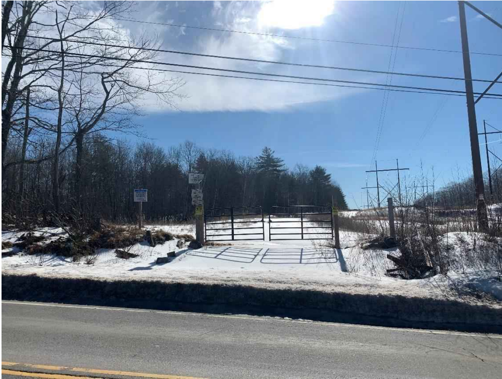
Photograph No. 13: Looking southerly at proposed access from Chester Street for 373 Structure 295 to be replaced.
