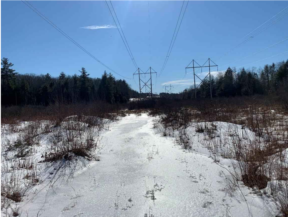
Photograph No. 9: Looking southerly at proposed access associated with Wetland CHW-10 towards 391 Structure 294 (left) and 373 Structure 297 (right) to be replaced. Timber matting will be used in the wetland portion of the access route.
