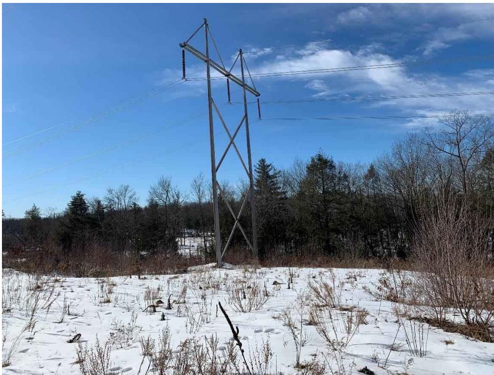
Photograph No. 8: Looking westerly at proposed access route towards 373 Structure 298 to be replaced.
