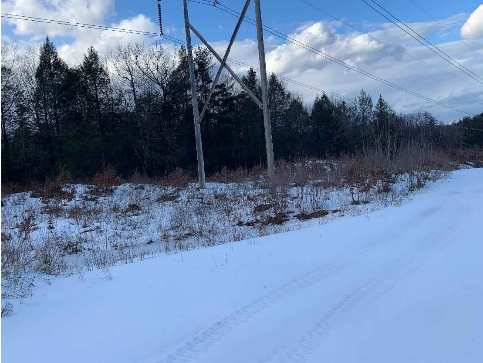
Photograph No. 5: Looking northwesterly at proposed access route associated with Wetland CHW-13 and 373 Structure 300. Timber matting will be used in the wetland portion of the access route.
