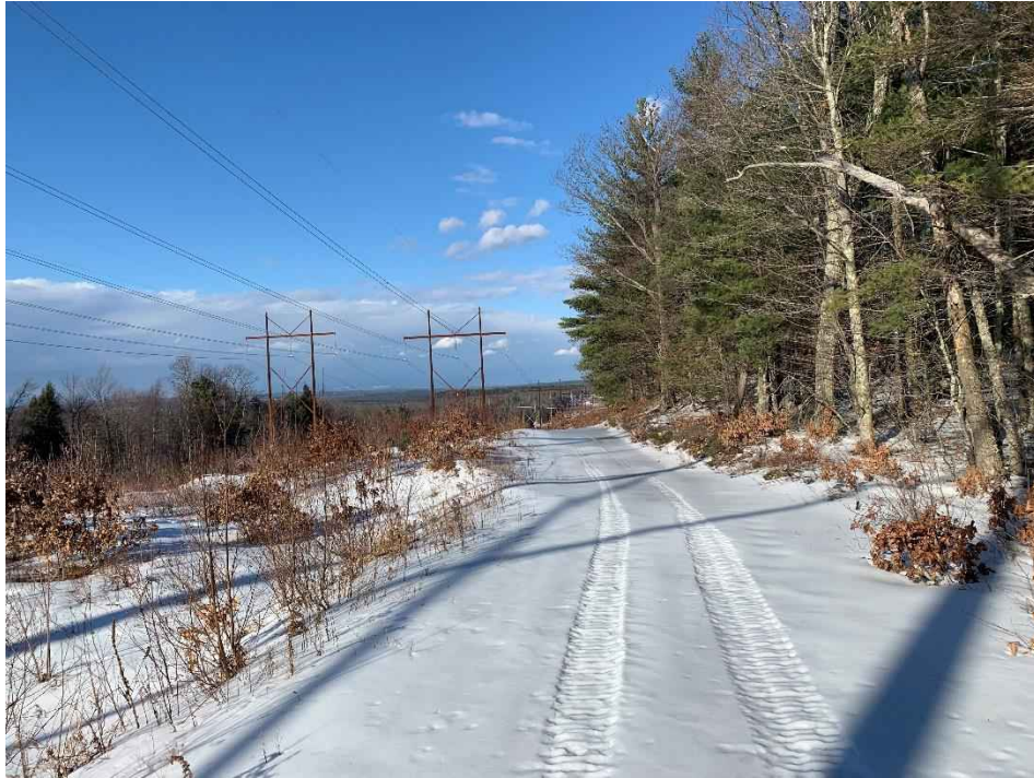
Photograph No. 3: Looking northerly at proposed access towards 391 Structure 299.
