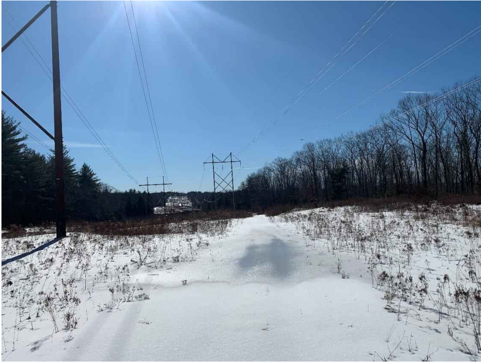
Photograph No. 11: Looking southerly at proposed access route for 373 Structure 296 to be replaced.
