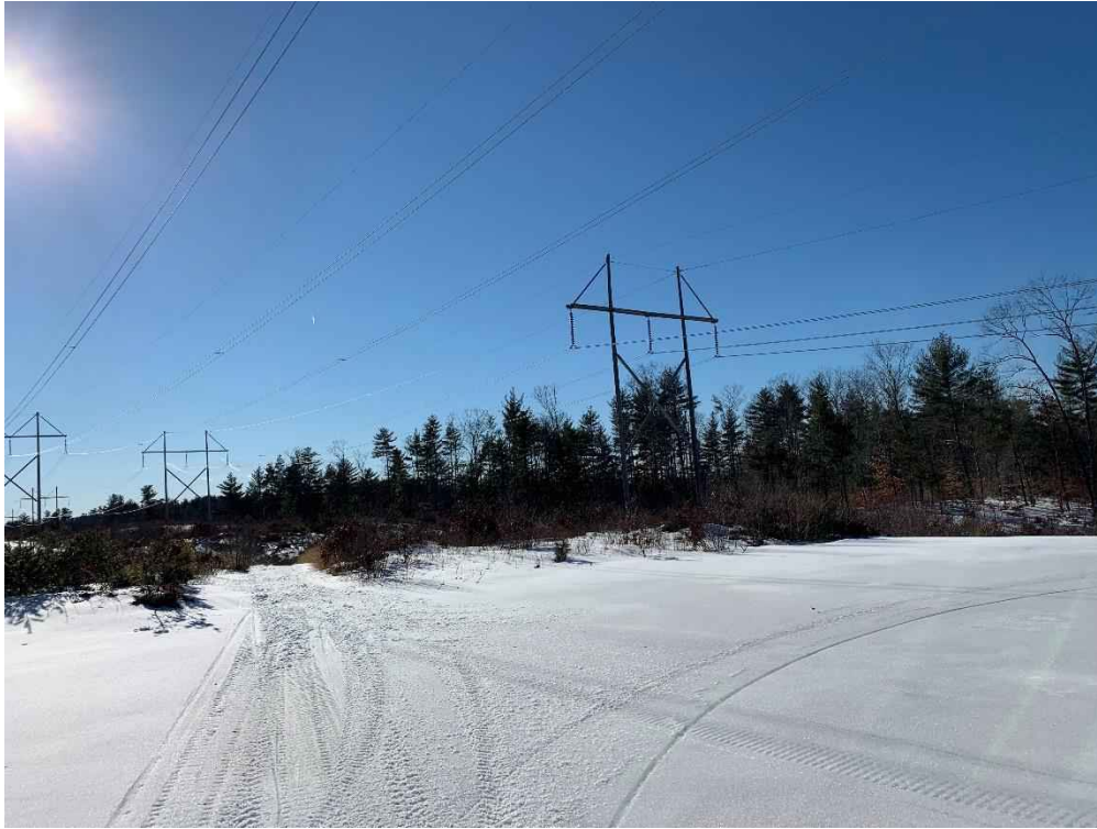
Photograph No. 17: Looking westerly at proposed access to 373 Structure 275 to be replaced.
