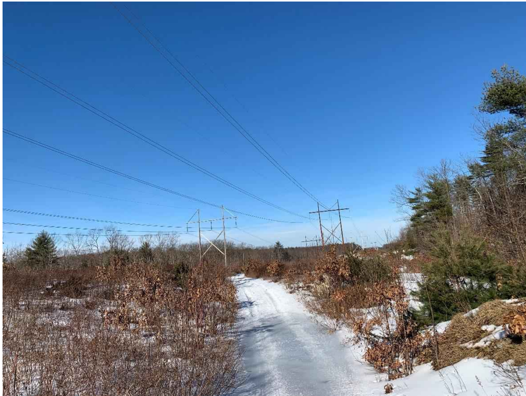
Photograph No. 20: Looking northerly at proposed access towards 391 Structure 273 (right) and 373 Structure 275 (left) to be replaced.
