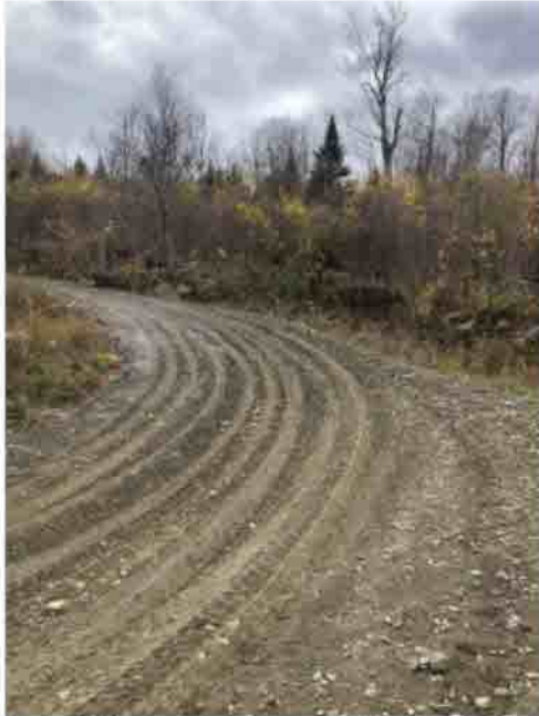
Figure 8- Shows berm on corner of trail
