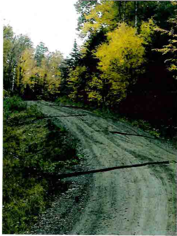
Figure 8 and 9- Picture on right shows the good exits of the newly installed culverts. Picture on left shows the rubber water diversion devices installed.
