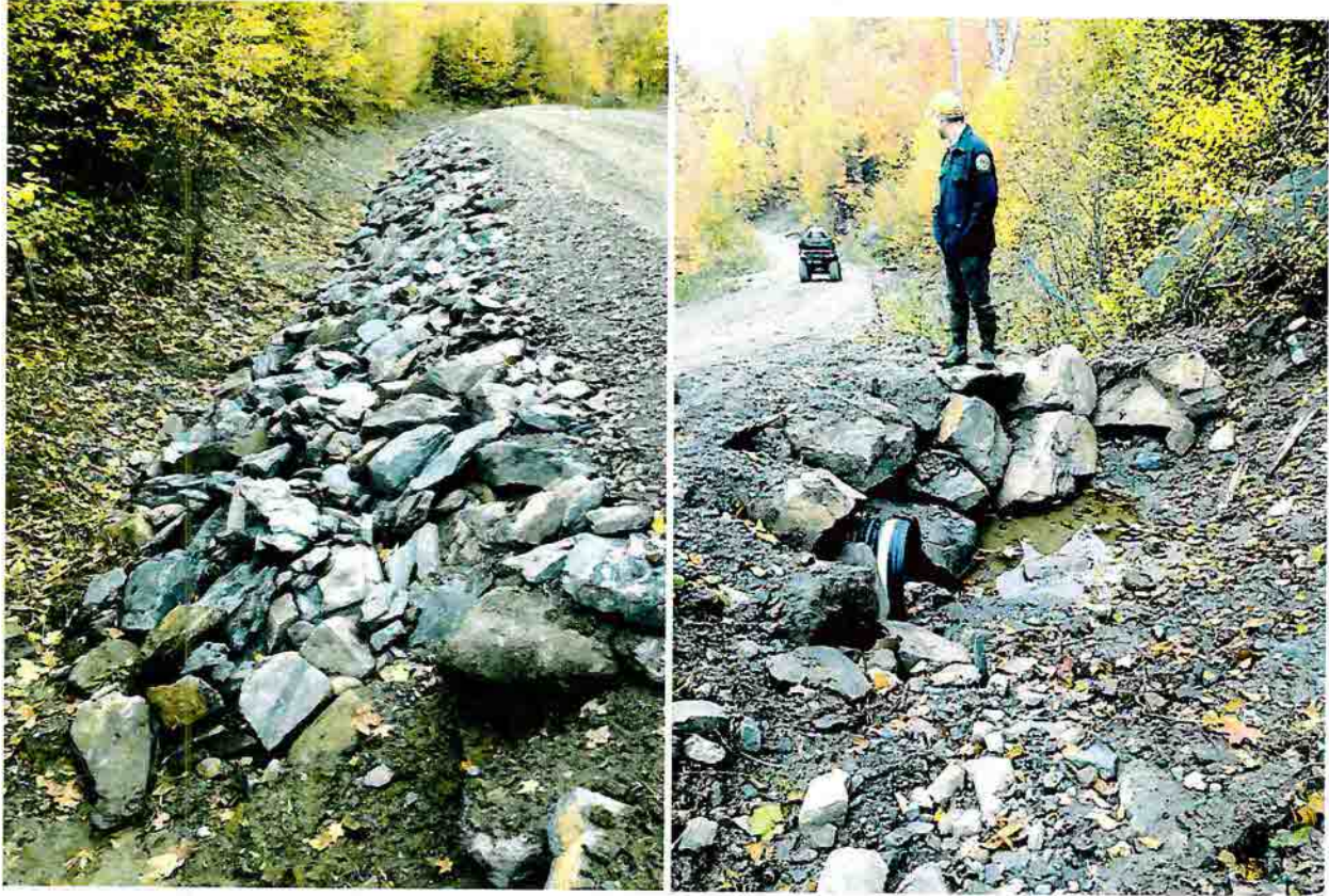
Figure 11 and 12- Depicts the newly fixed and armored ditch where the washout was previously. Also shows a newly installed culvert.
