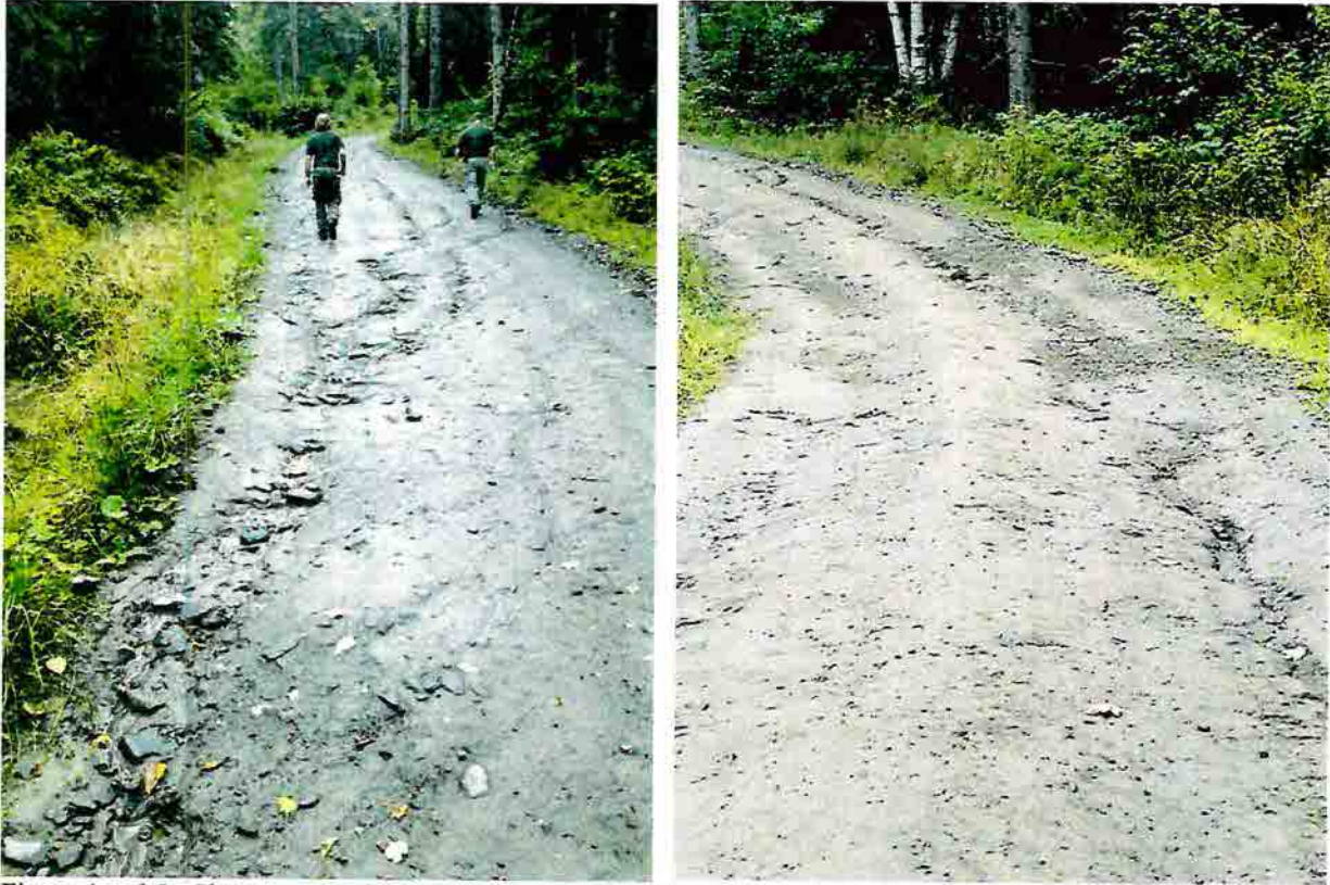
Figure 4 and 5- Shows some of the wear on the trail heading toward Colebrook.
