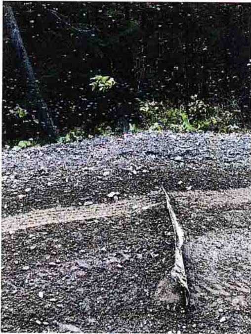
Figure 4- Showing the water diversion device
