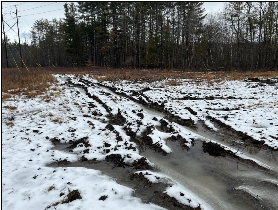
Photo 2: View looking northwest at proposed timber matting access location north of Structure 93 off Madbury Road in Madbury.
