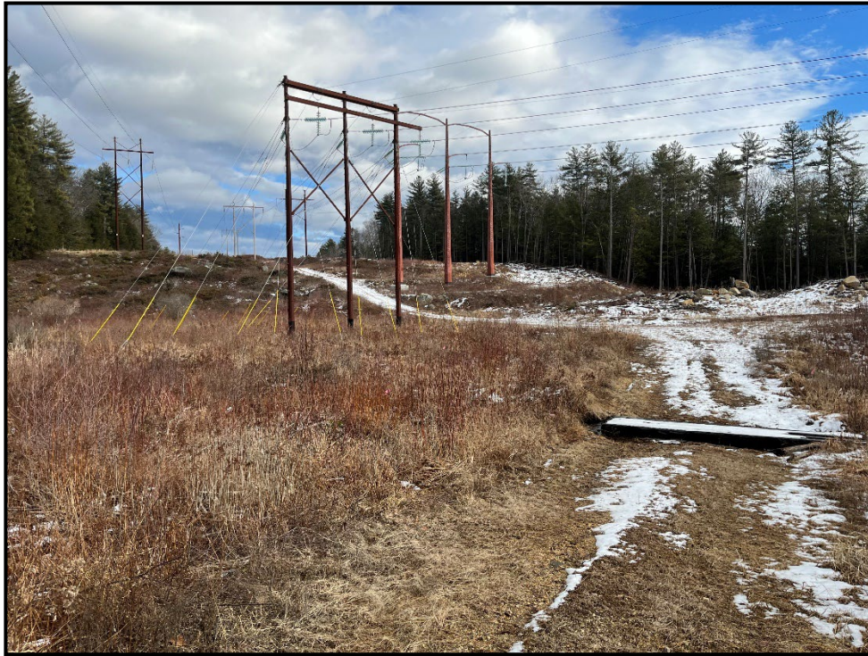
Photo 9: View of proposed timber matting location near Structure 187 off Cate Road in Deerfield.
