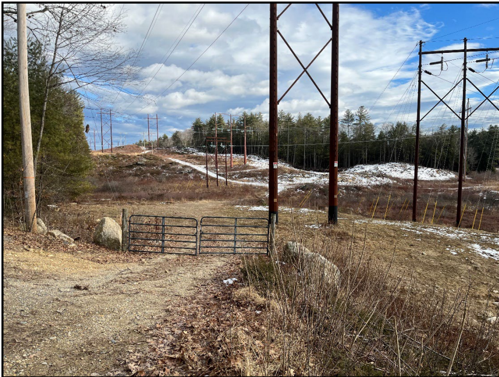
Photo 8: Existing access location near Structure 187 off Cate Road in Deerfield.
