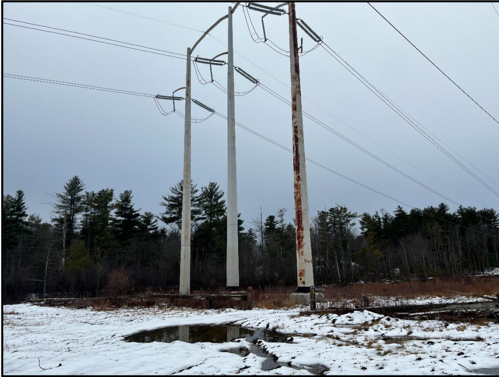
Photo 1: View southwest of proposed timber matting location at Structure 93 off Madbury Road in Madbury.
