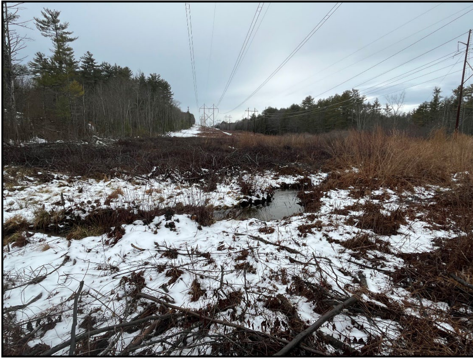
Photo 3: View looking west across Bears Creek through ROW toward Structure 94 off Madbury Road in Madbury.
