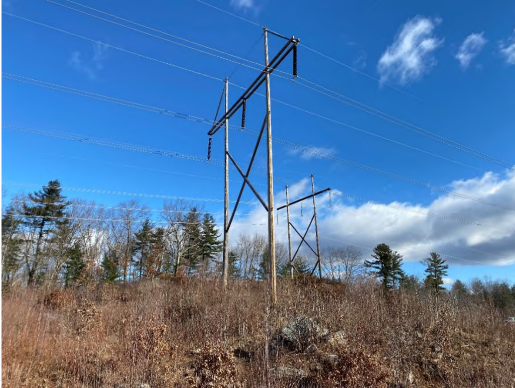
Photograph No. 41: Looking at proposed access and work pad location adjacent to Structure 7 of the 326 Line.
