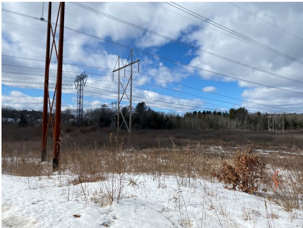
Photograph No. 10: Looking at proposed access and work pad location adjacent to Structure 69 of the 326 Line from Route 102.
