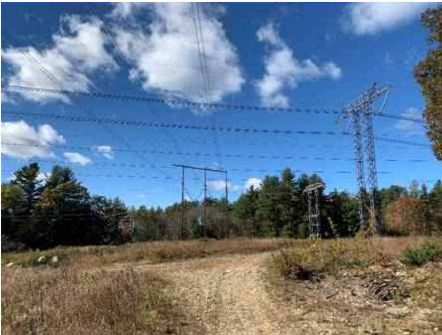
Photograph No. 4: Looking west at proposed trench location leading to Structure 380-58.
