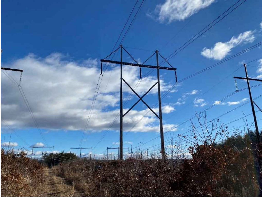
Photograph No. 37: Looking at proposed access and work pad location for Structure 11 of the 326 Line.
