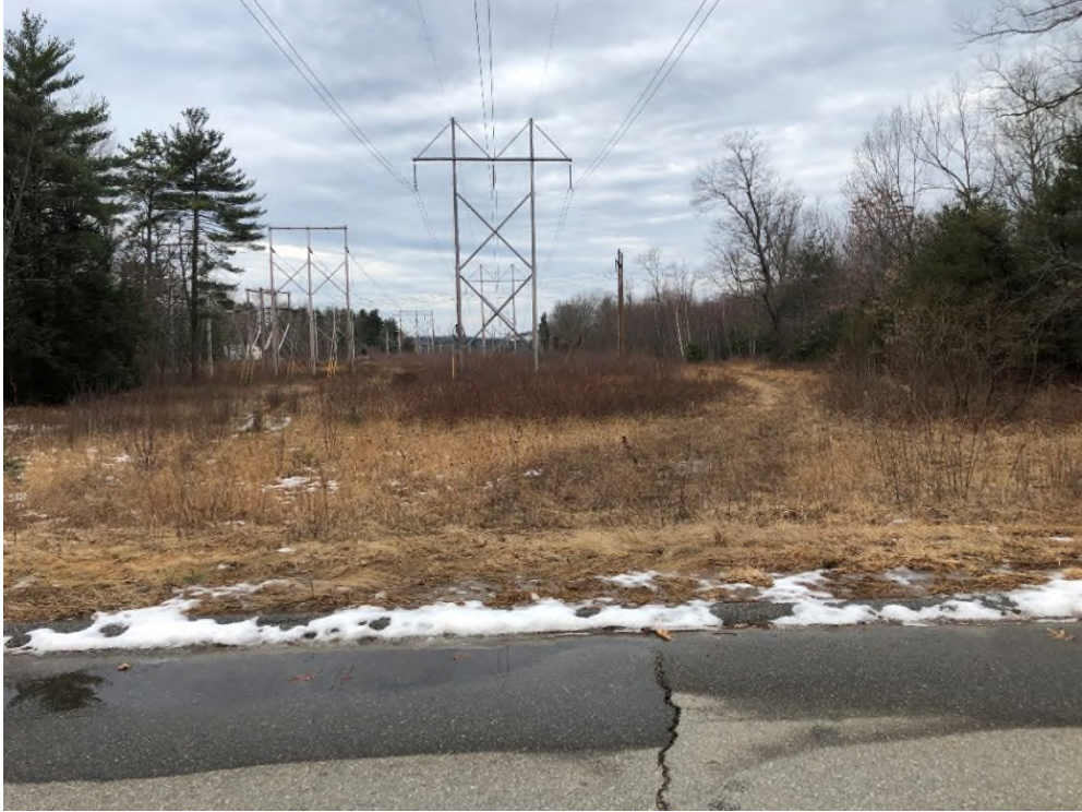
Photograph No. 1: Looking at proposed access and work pad location from Brick Yard Drive for Structure 85 of the 380 Line.
