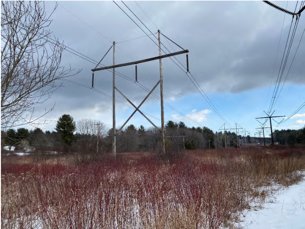
Photograph No. 21: Looking at proposed work pad location for Structure 153 of the 326 Line.
