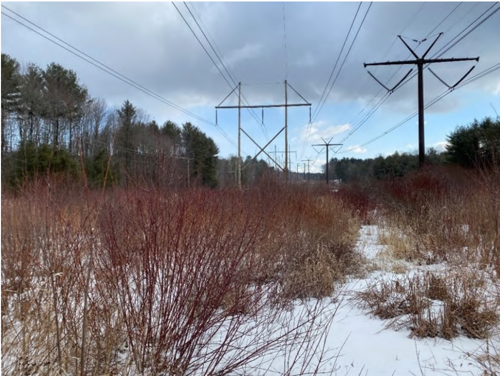
Photograph No. 20: Looking at proposed access and work pad location for Structure 152 of the 326 Line.
