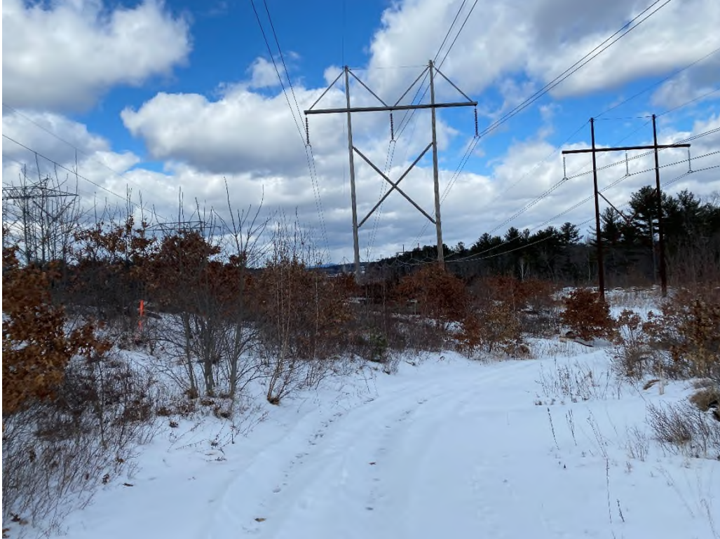
Photograph No. 15: Looking at proposed access and work pad location for Structure 78 of the 326 Line.
