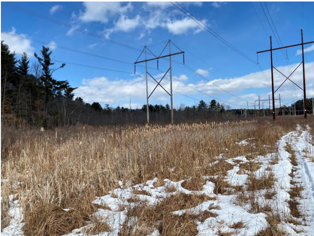
Photograph No. 28: Looking at proposed access and work pad location adjacent to Structure 28 of the 380 Line.
