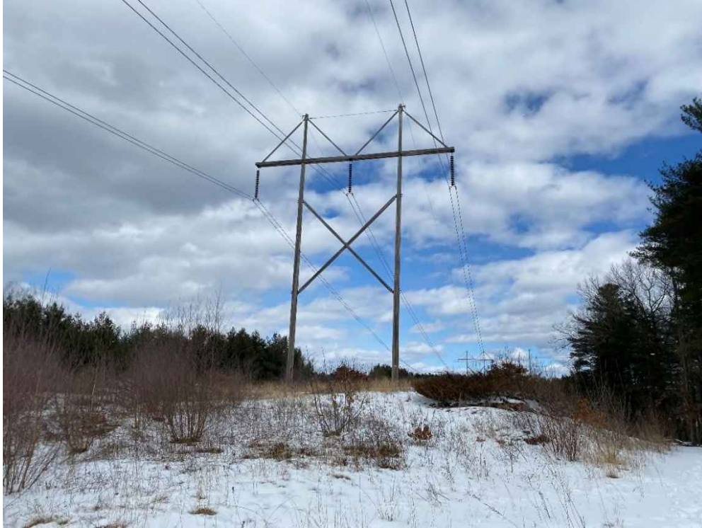
Photograph No. 5: Looking at proposed access and work pad location adjacent to Structure 62 of the 380 Line.
