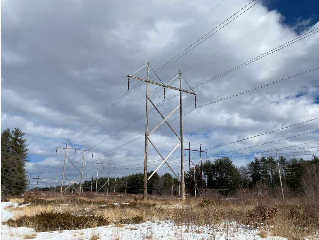
Photograph No. 7: Looking at proposed access and work pad location adjacent to Structure 56 of the 380 Line.
