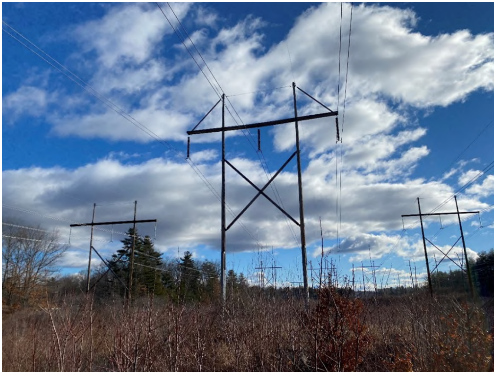
Photograph No. 40: Looking at proposed access and work pad location for Structure 8 of the 326 Line.
