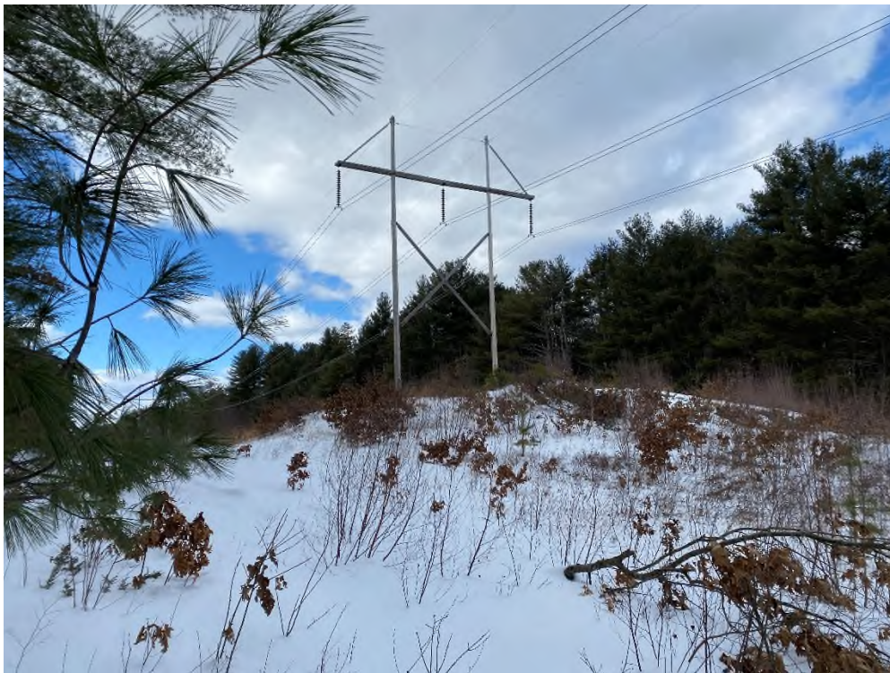
Photograph No. 4: Looking at proposed access and work pad location for Structure 65 of the 380 Line.
