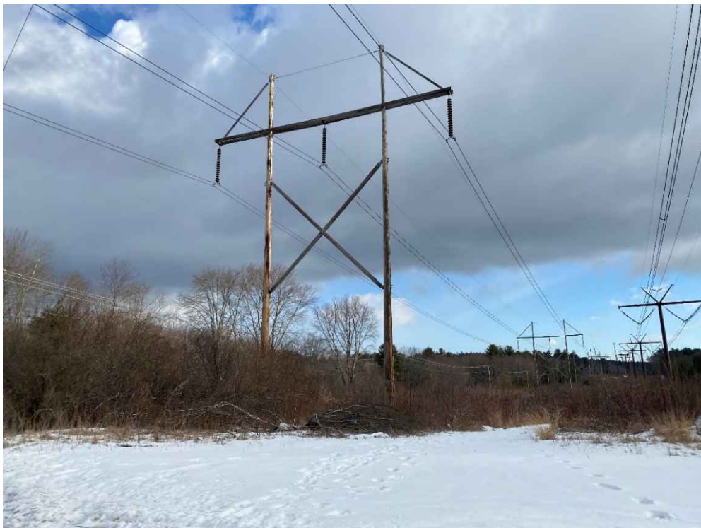
Photograph No. 22: Looking at proposed access and work pad location for Structure 154 of the 326 Line.
