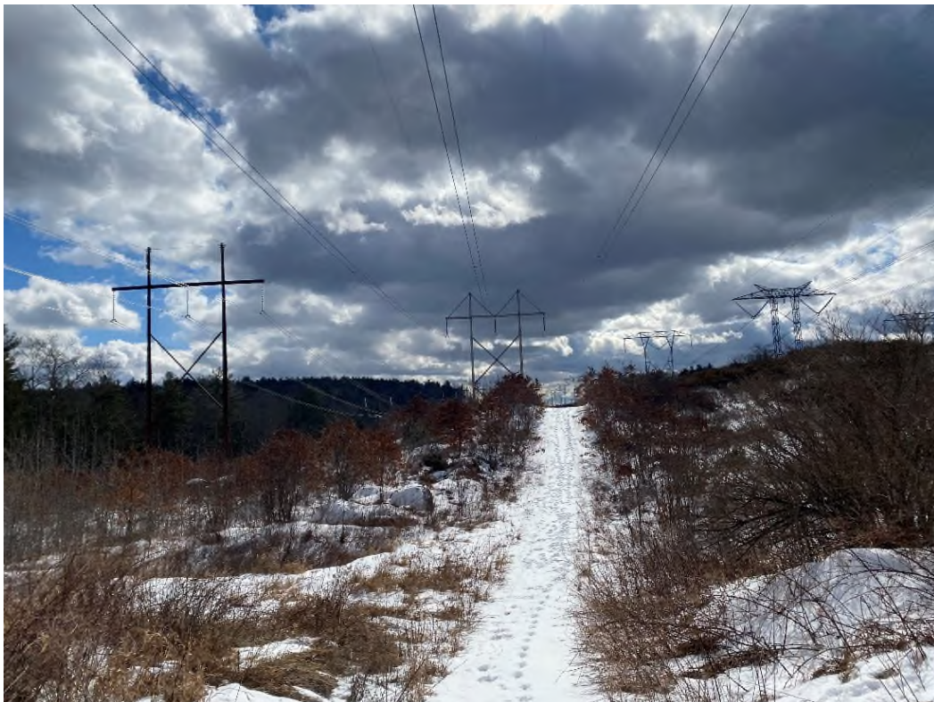
Photograph No. 16: Looking at proposed access and work pad location for Structure 79 of the 326 Line.
