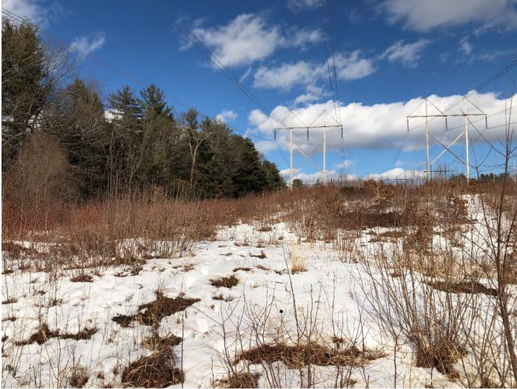
Photograph No. 31: Looking at proposed access and work pad location adjacent to Structure 23 of the 380 Line.
