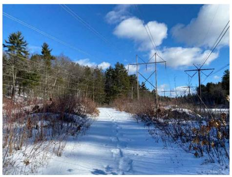
Photograph No. 2: Looking northeasterly at proposed access route to Structure 123 of the 326 Line to be replaced, associated with Wetland HW-45. Timber matting will be used in the wetland portion of the access route.
