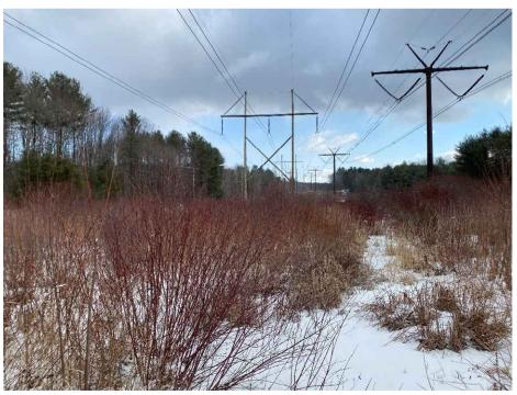
Photograph No. 6: Looking northeasterly at proposed access route and work pad associated with Wetland HW-81 towards Structure 152 of the 326 Line to be replaced. Timber matting will be used in the wetland portion of the access route and work pad.
