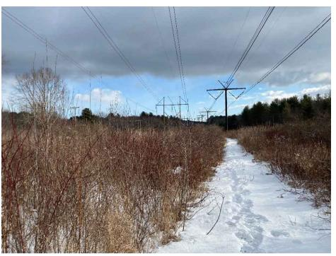
Photograph No. 3: Looking northeasterly at proposed access towards Structure 153 of the 326 Line to be replaced, across Wetland H-81. Timber matting will be used in the wetland portion of the access route.
