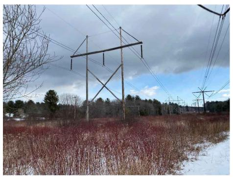
Photograph No. 4: Looking northeasterly at proposed access and work pad location for Structure 153 of the 326 Line to be replaced, associated with Wetland HW-81. Timber matting will be used in the wetland portion of the access route and work pad.
