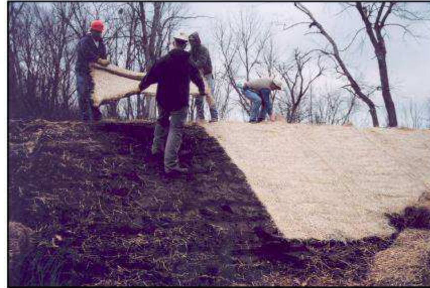
Best Management Practice 15: Erosion Control Blankets
