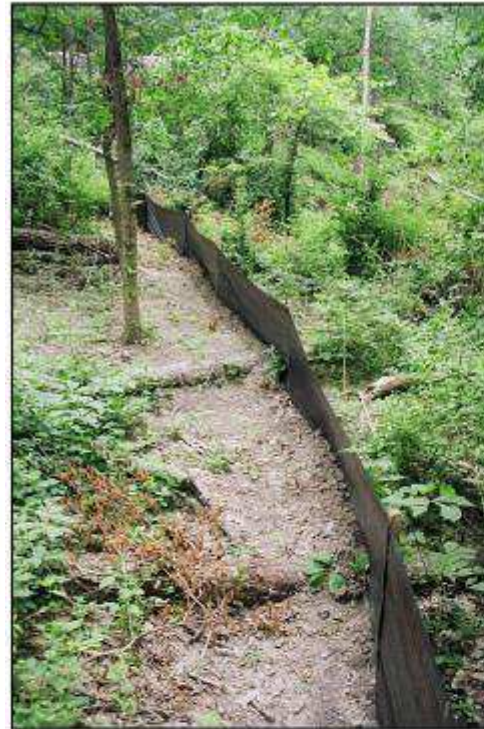
Best Management Practice 5: Silt Fence
