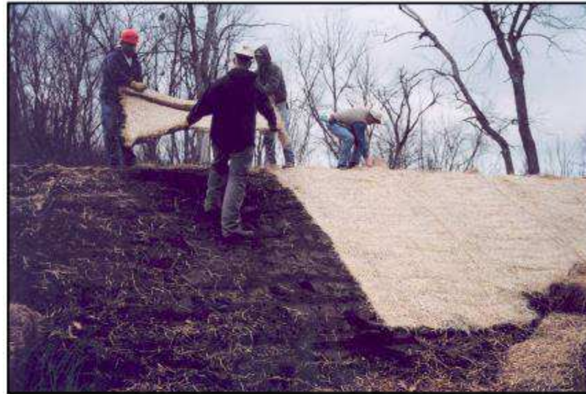
Best Management Practice 15: Erosion Control Blankets
