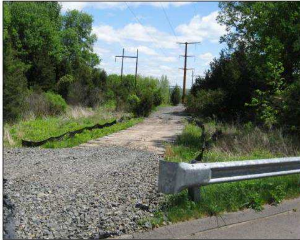
Best Management Practice 3: Temporary Construction Exit
