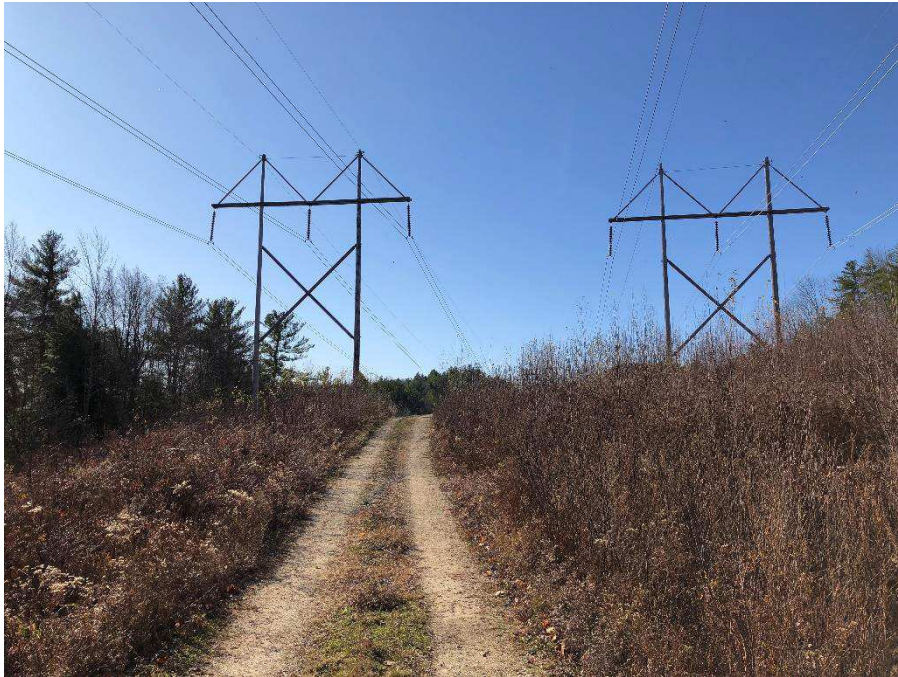
Photograph No. 35: Looking southwesterly at proposed existing access route between 391 structure 150 (right) and 385 structure 147 (Left) in Northwood.
