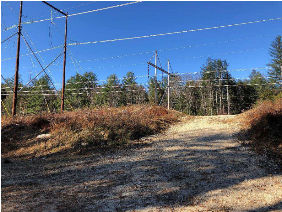
Photograph No. 32: Looking northwesterly at proposed existing access route in Northwood.
