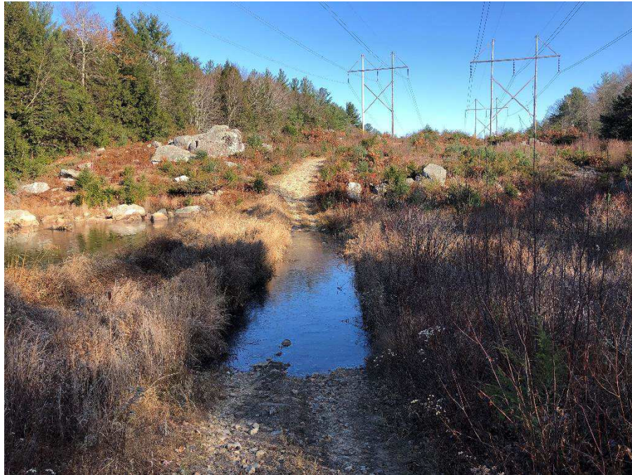
Photograph No. 13: Looking northerly at proposed access route between structures 156 and 155 in Deerfield.
