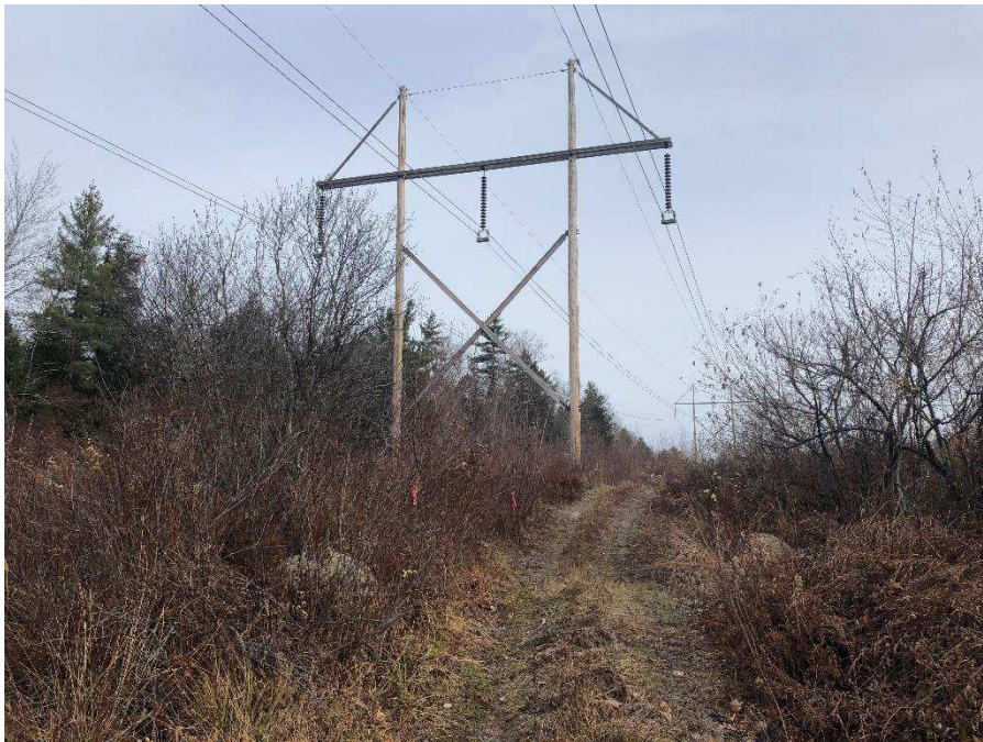
Photograph No. 40: Looking northeasterly at proposed access route and work pad location adjacent to 385 Line Structure 94 Strafford.
