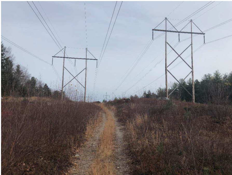
Photograph No. 42: Looking northeasterly at proposed access route lead to 391 Structures 98 and 385 Structure 93 in Strafford.
