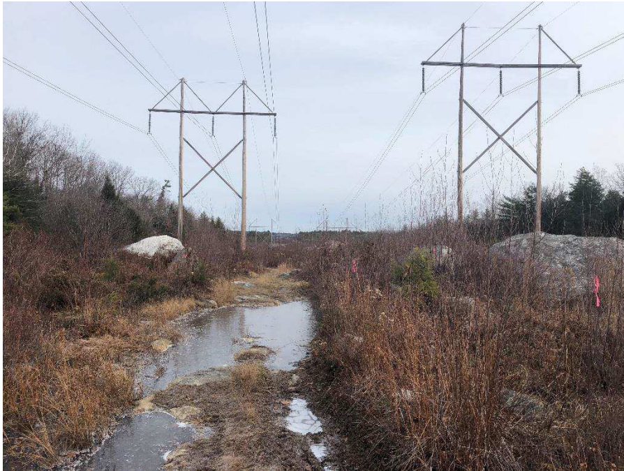
Photograph No. 45: Looking northeasterly at proposed access route lead to 391 Structures 97 and 385 Structure 92 in Strafford.
