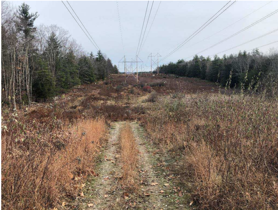
Photograph No. 39: Looking northeasterly at proposed access route between 391 Structures 99 and 385 Structure 94 in Strafford.
