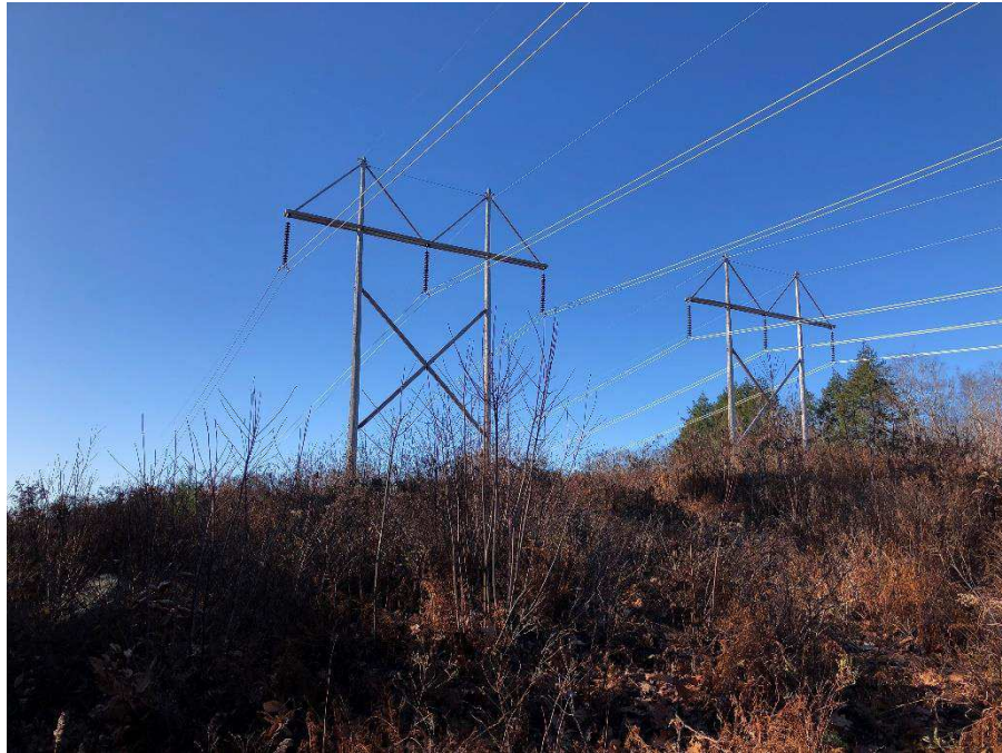
Photograph No. 25: Looking westerly at proposed structure replacement 391 structure 156 (left) and 385 structure 152 (right) in Deerfield.
