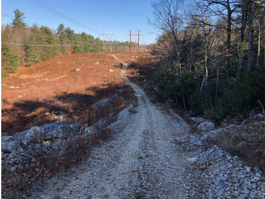
Photograph No. 29: Looking northeasterly at proposed existing access route between structures 154 & 153 on the 391 line in Northwood.
