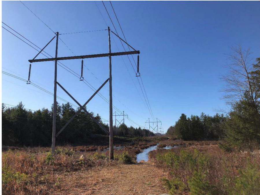
Photograph No. 5: Looking southwesterly at proposed structure replacement 385 Structure 158 in Deerfield.
