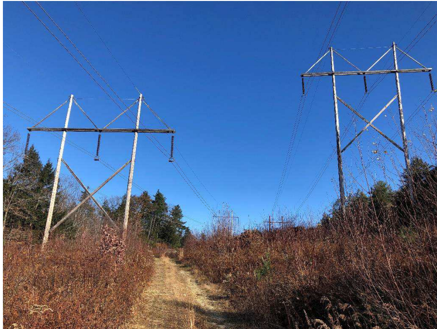
Photograph No. 27: Looking northeasterly at proposed structure replacement 385 structure 151 (left) and 391 structure 155 (right) with proposed access route between structures in Deerfield.
