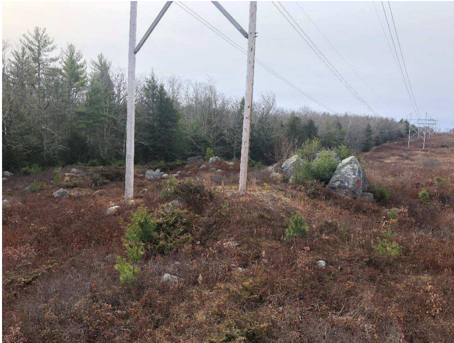
Photograph No. 53: Looking southerly at proposed work pad location adjacent to 391 Line Structure 93 Strafford.
