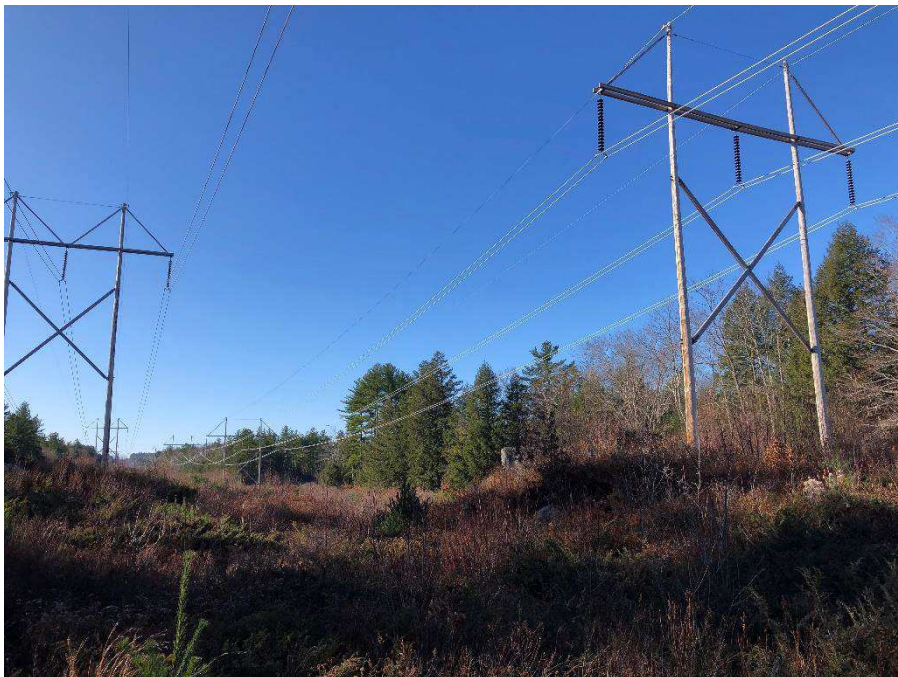
Photograph No. 8: Looking southwesteryly at proposed structure replacement 385 structure 157 on right in Deerfield.
