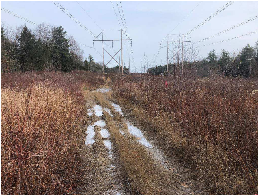
Photograph No. 52: Looking northeasterly at proposed access leading to 385 Structure 89 and 391 Structure 93.
