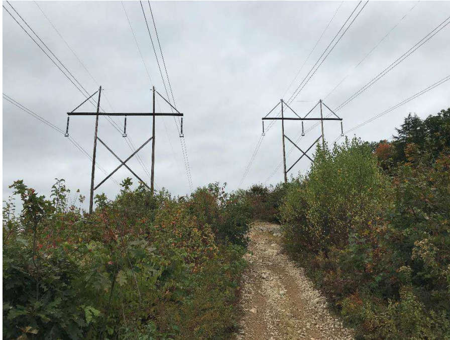
Photograph No. 3: Looking northerly at proposed access route toward 391 Structure 278 in Chester.
