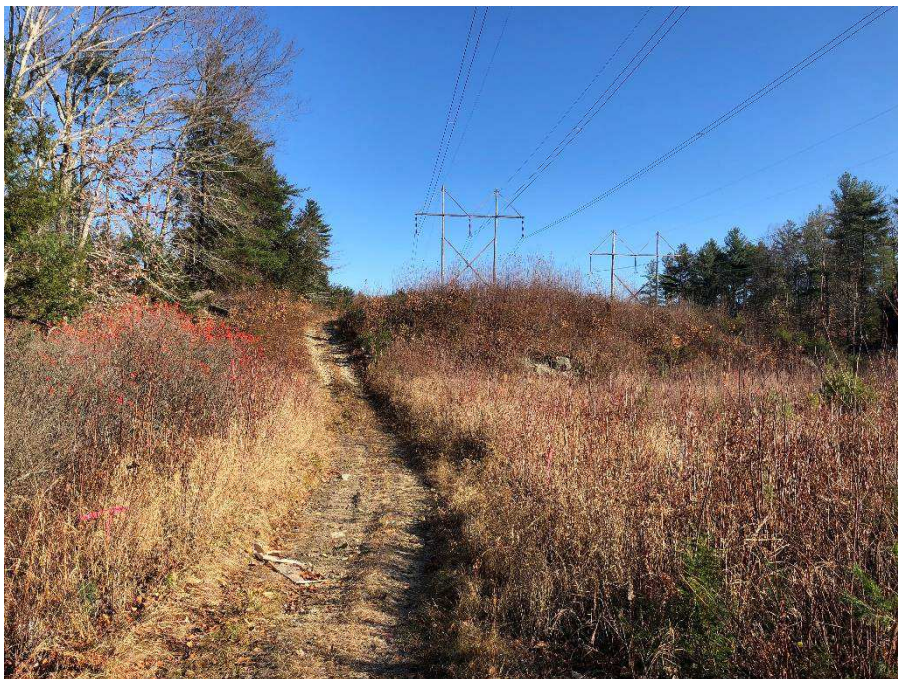
Photograph No. 10: Looking northeasterly at proposed access route between 385 structures 157 & 156 in Deerfield.
