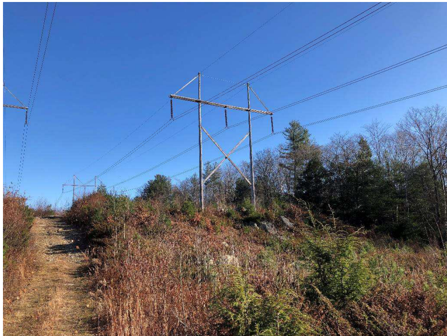
Photograph No. 14: Looking northeasterly at proposed structure replacement 385 structure 160 (right) with proposed access (left) in Deerfield.
