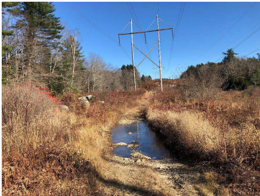
Photograph No. 22: Looking northeasterly at proposed access route and proposed structure replacement 385 structure 153 in Deerfield.
