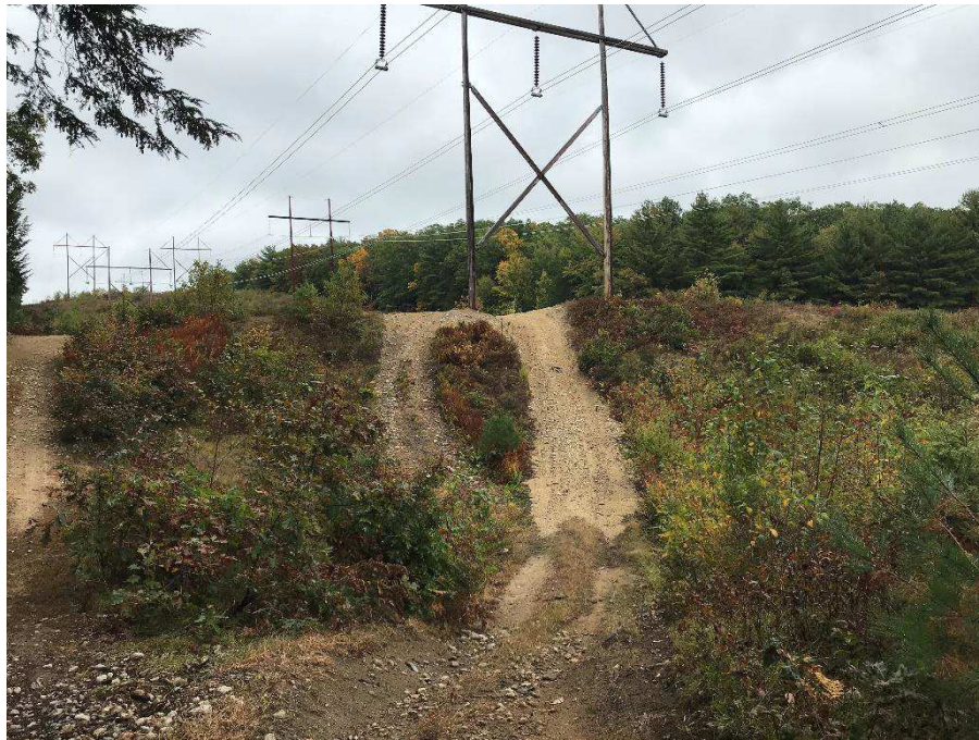
Photograph No. 2: Looking northwesterly at proposed structure replacement 391 Structure 286 in Chester.
