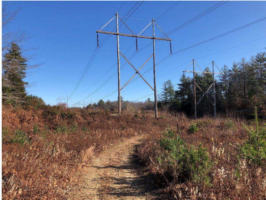
Photograph No. 11: Looking northeasterly at proposed structure replacement 385 structure 156 in Deerfield.
