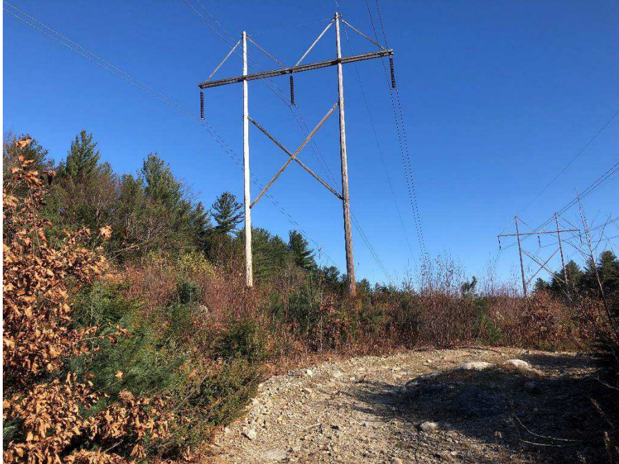
Photograph No. 15: Looking northerly at proposed structure replacement 385 structure 155 in Deerfield.
