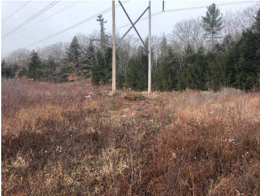
Photograph No. 49: Looking westerly at proposed work pad location adjacent to 385 Line Structure 91 Strafford.
