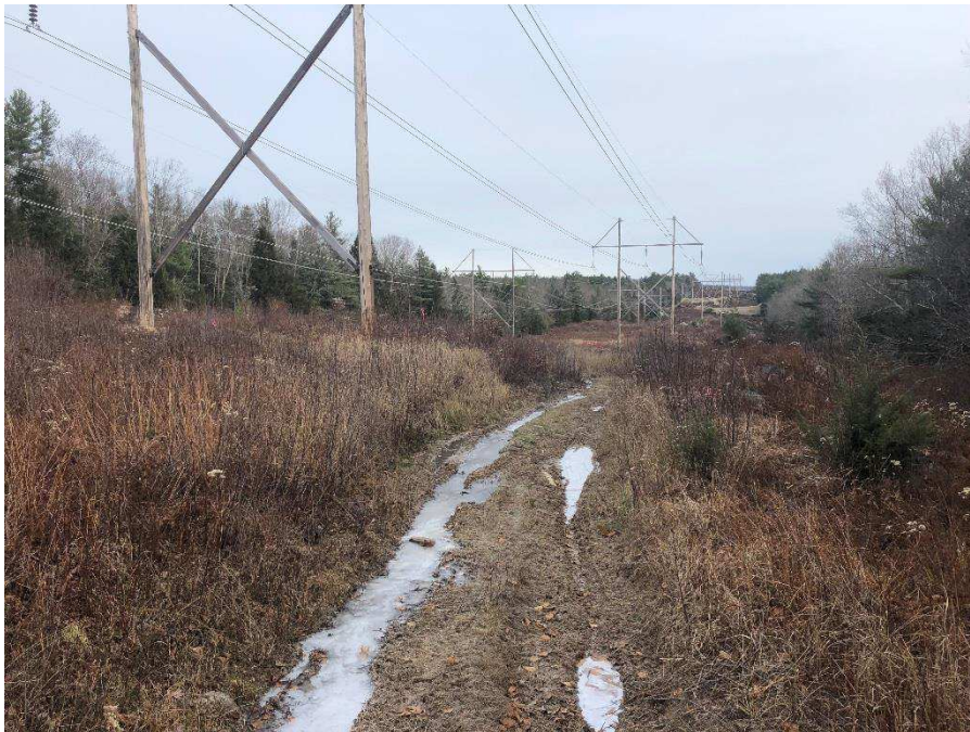
Photograph No. 48: Looking northerly at proposed work pad location adjacent to 391 Line Structure 95 Strafford.
