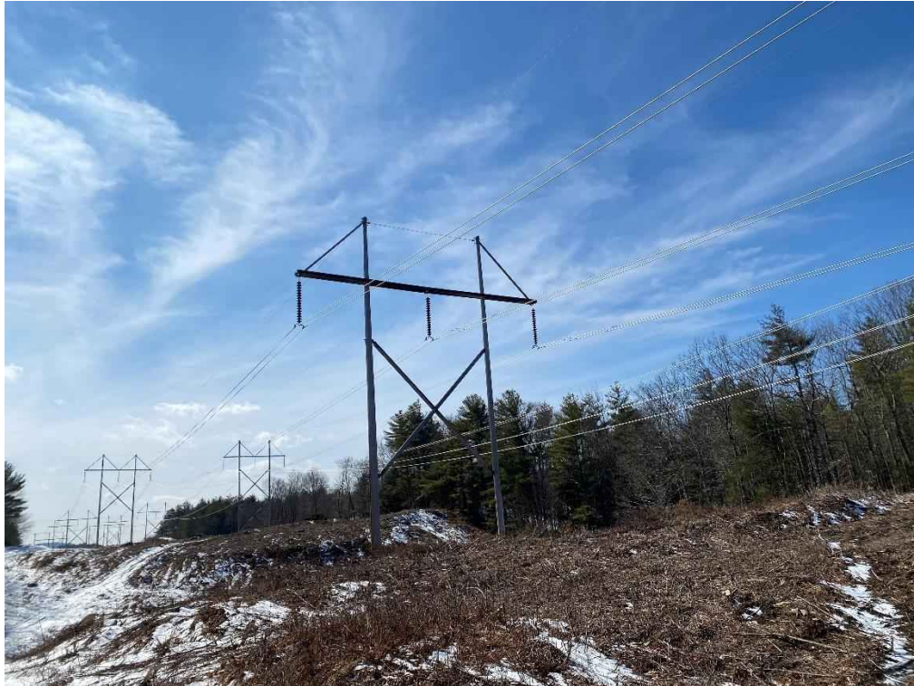
Photograph No. 33: View of proposed access to 373 Line Structure 145.
