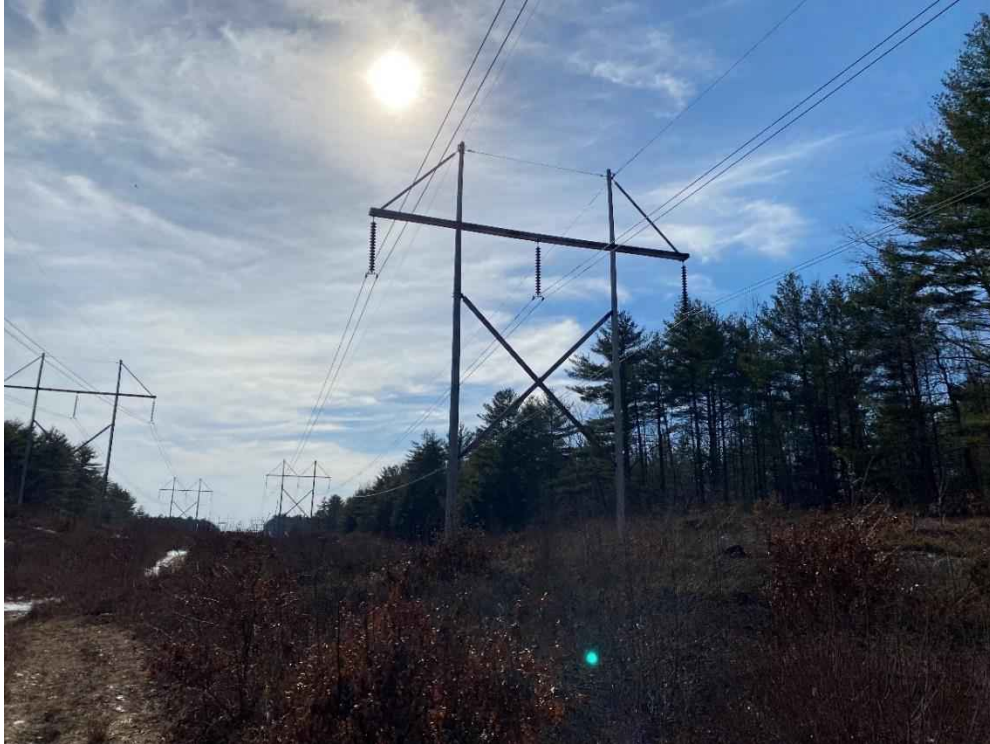
Photograph No. 19: View of proposed work pad location for 373 Line Structure 262.
