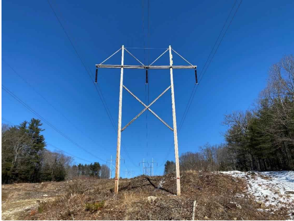
Photograph No. 37: View of proposed access and work pad location for 391 Line Structure 131.
