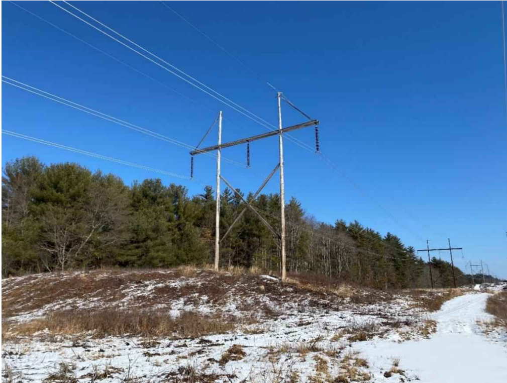
Photograph No. 43: View of proposed access and work pad location adjacent to 385 Line Structure 80.
