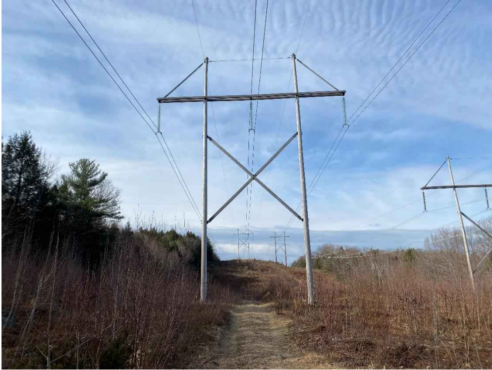
Photograph No. 25: View of proposed access and work pad location adjacent to 391 Line Structure 192.
