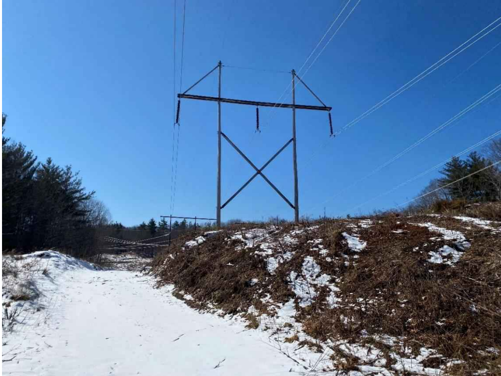
Photograph No. 41: View of proposed access to 391 Line Structure 121.
