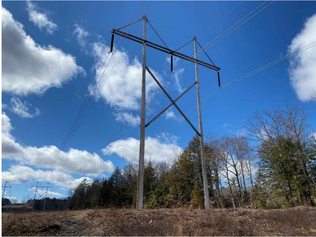
Photograph No. 63: View of proposed access and work pad location for 385 Line Structure 23.
