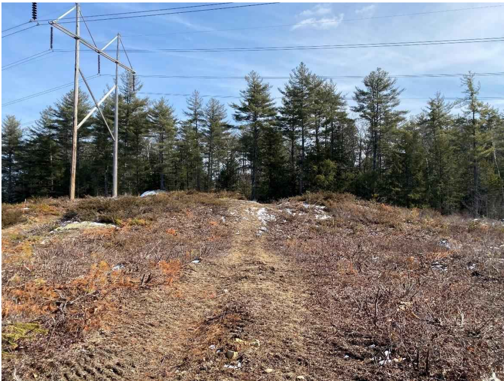
Photograph No. 22: View of proposed access and work pad location for 373 Line Structure 247.
