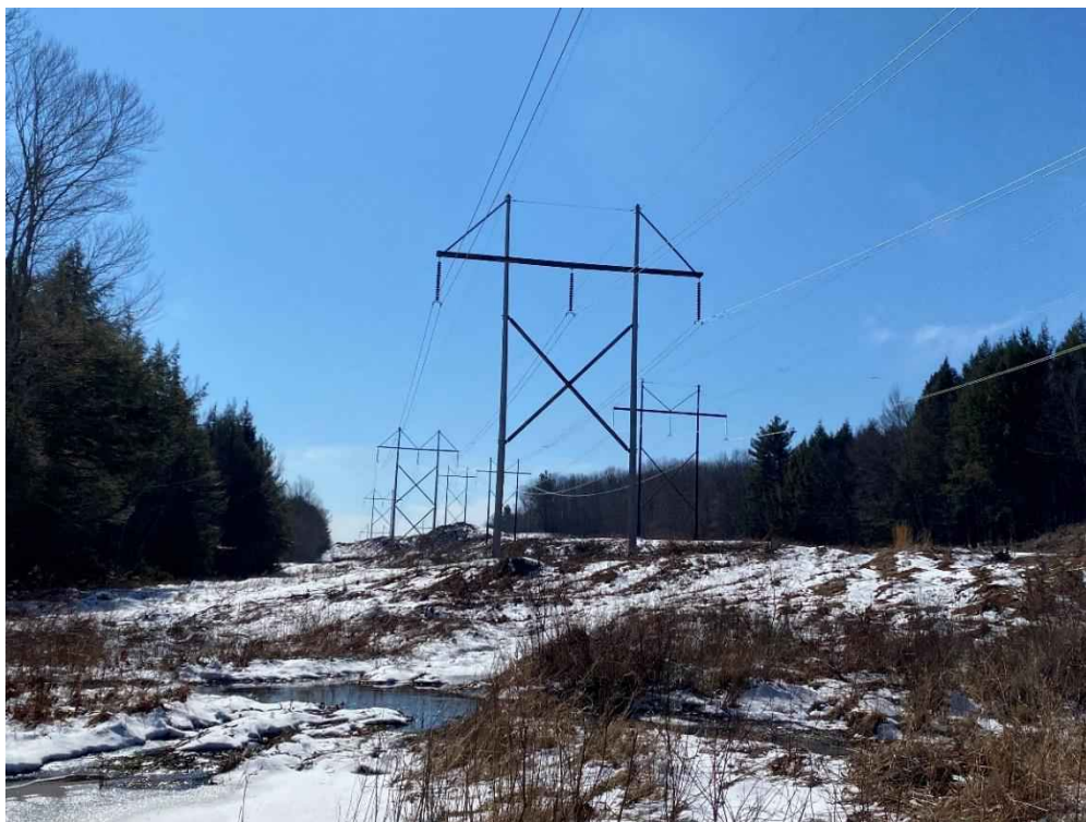
Photograph No. 34: View of proposed access to 391 Line Structure 133.
