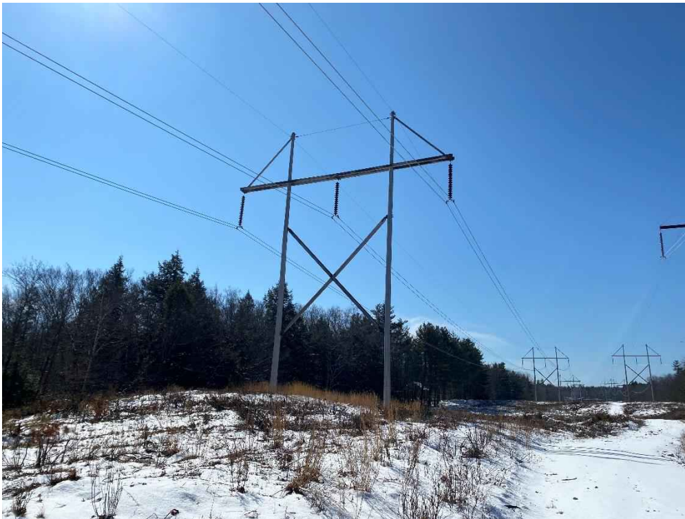
Photograph No. 42: View of proposed access and work pad location for 391 Line Structure 116.
