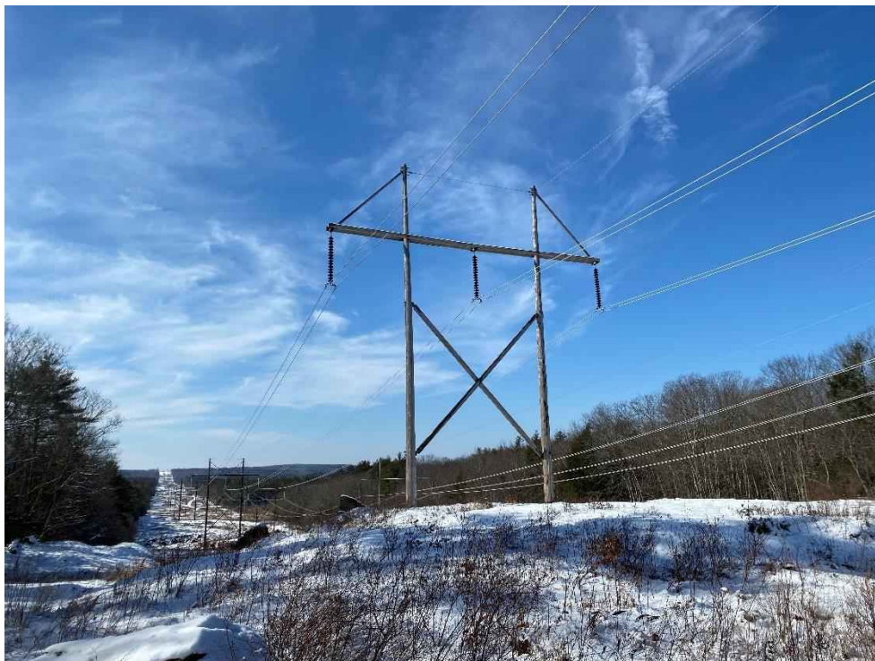
Photograph No. 48: View of proposed access and work pad location for 391 Line Structure 78.
