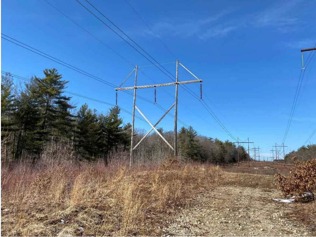
Photograph No. 21: View of proposed access and work pad location for 373 Line Structure 255.
