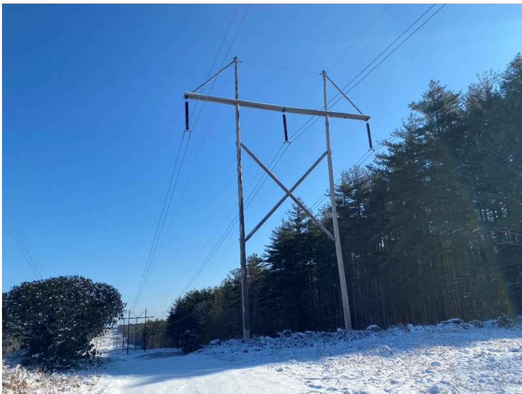
Photograph No. 60: View of proposed access and work pad location for 391 Line Structure 46.
