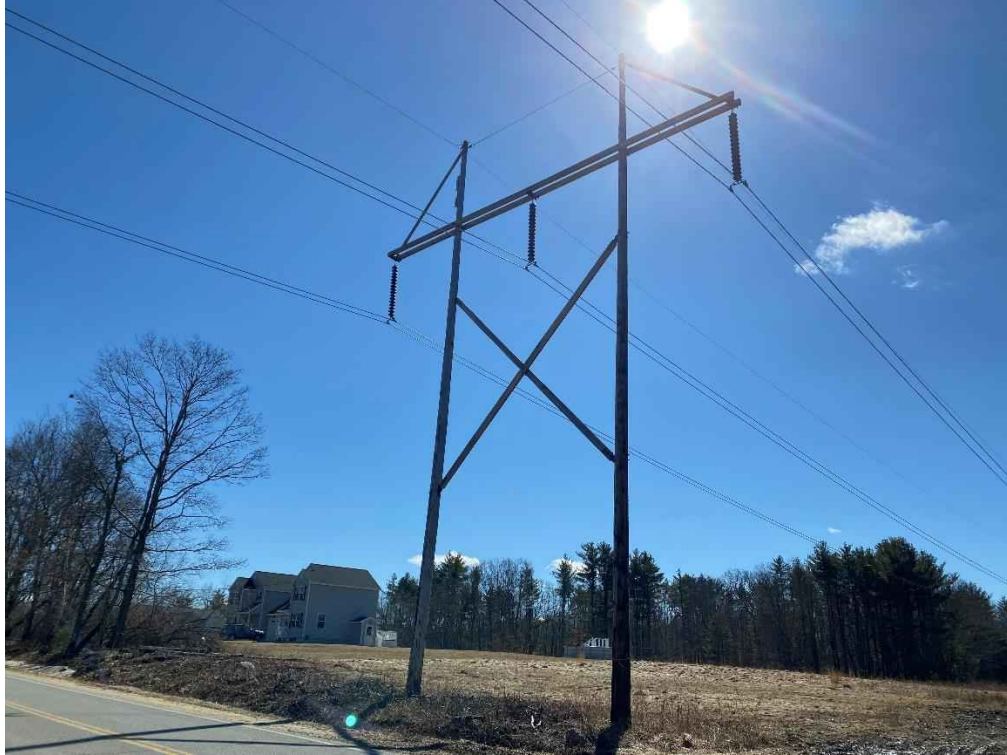
Photograph No. 57: View of proposed access and work pad location for 391 Line Structure 71 from Second Crown Point Road.
