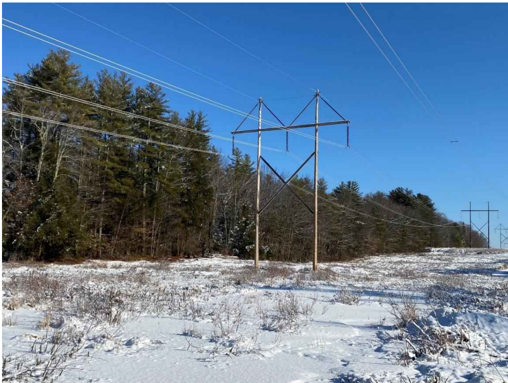
Photograph No. 62: View of proposed access and work pad location for 385 Line Structure 33.
