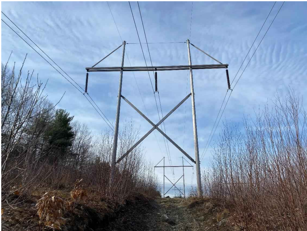
Photograph No. 26: View of proposed access and work pad location for 391 Line Structure 191.
