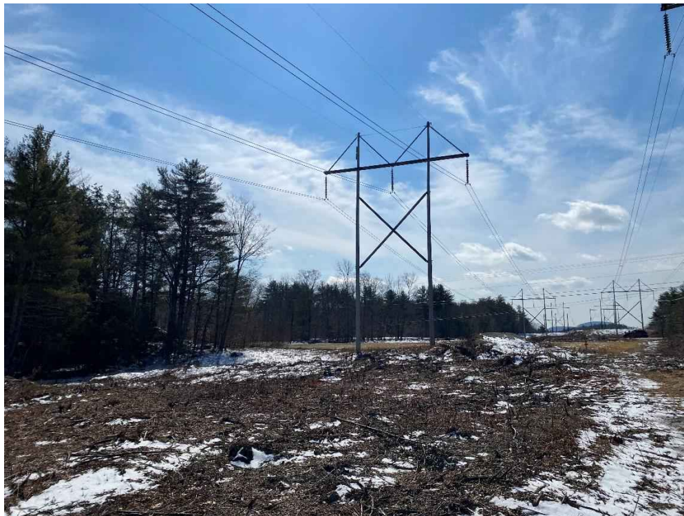
Photograph No. 32: View of proposed access to 373 Line Structure 146.
