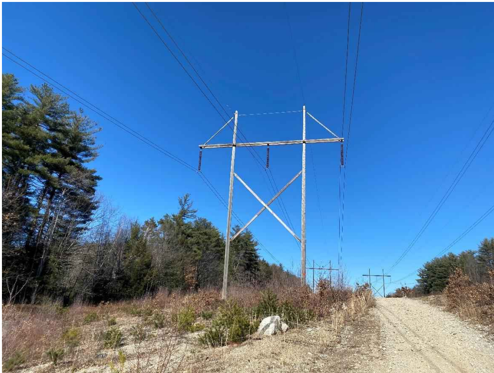
Photograph No. 24: View of proposed access and work pad location for 373 Line Structure 235.
