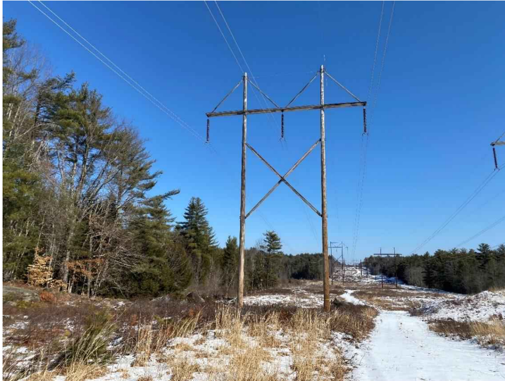
Photograph No. 45: View of proposed access and work pad location for 385 Line Structure 77.
