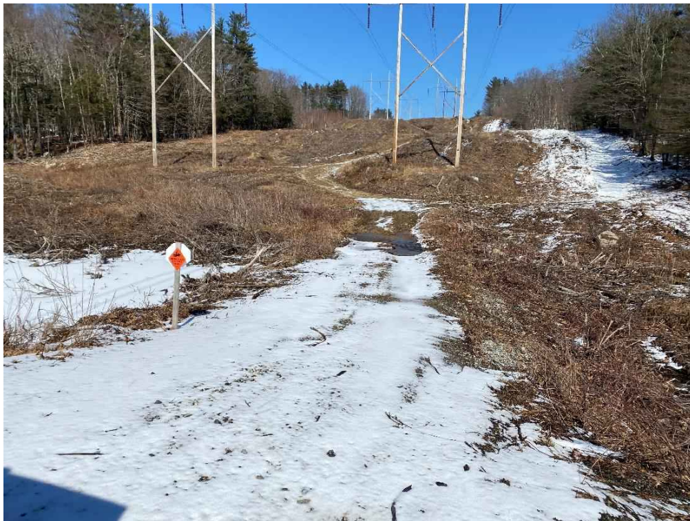
Photograph No. 36: View of proposed access to 385 Line Structure 127.
