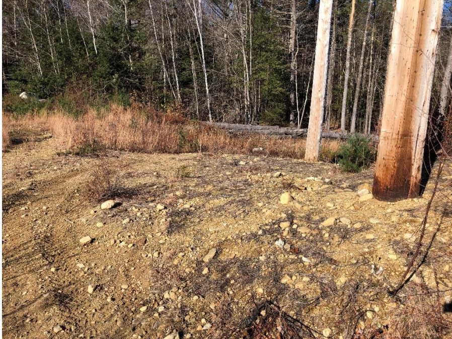
Photograph No. 19: Looking northwesterly at proposed structure replacement 385 structure 154 work pad in Deerfield.
