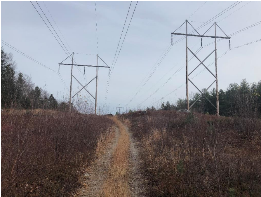
Photograph No. 42: Looking northeasterly at proposed access route lead to 391 Structures 98 and 385 Structure 93 in Strafford.
