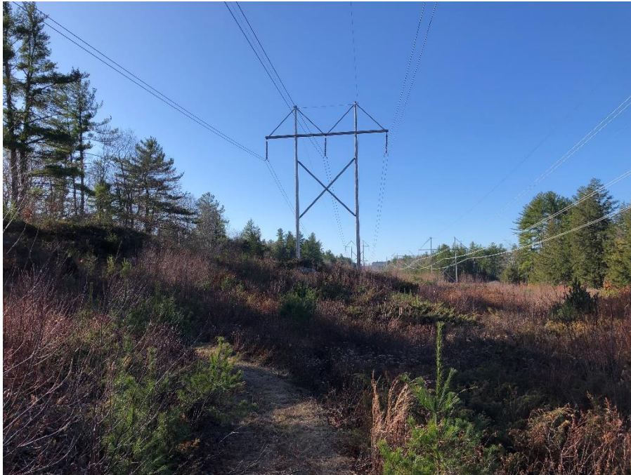
Photograph No. 9: Looking southwesterly at proposed structure replacement 391 structure 162 and proposed access in Deerfield.
