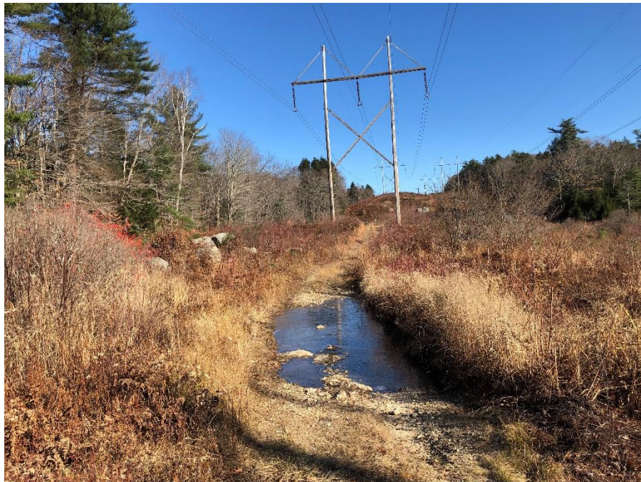
Photograph No. 22: Looking northeasterly at proposed access route and proposed structure replacement 385 structure 153 in Deerfield.
