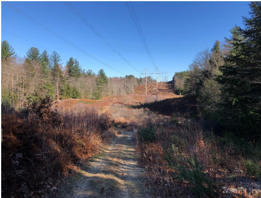
Photograph No. 20: Looking northeasterly at proposed access route between structures 158 & 157 on the 391 line in Deerfield.
