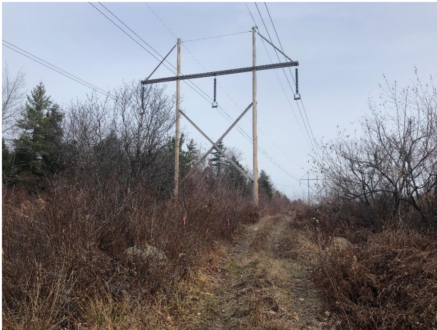
Photograph No. 40: Looking northeasterly at proposed access route and work pad location adjacent to 385 Line Structure 94 Strafford.
