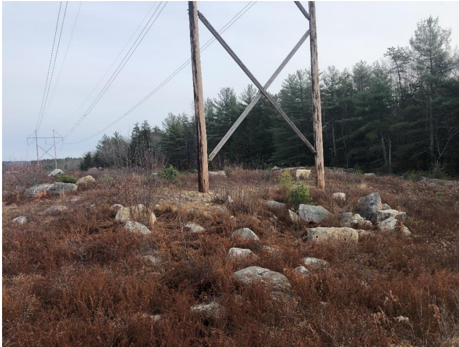
Photograph No. 43: Looking northeasterly at proposed work pad location adjacent to 391 Line Structure 98 Strafford.
