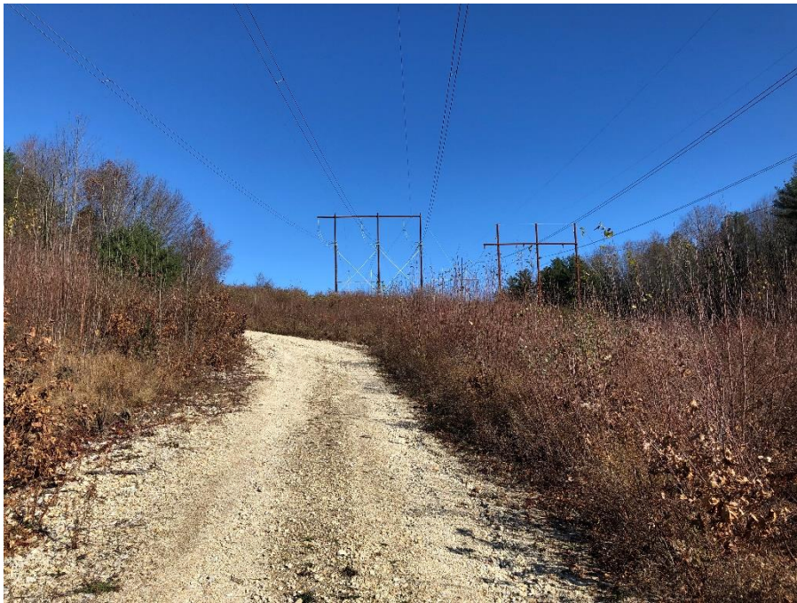
Photograph No. 36: Looking northeasterly at proposed existing access route between structures 146 & 147 on the 385 line in Northwood.
