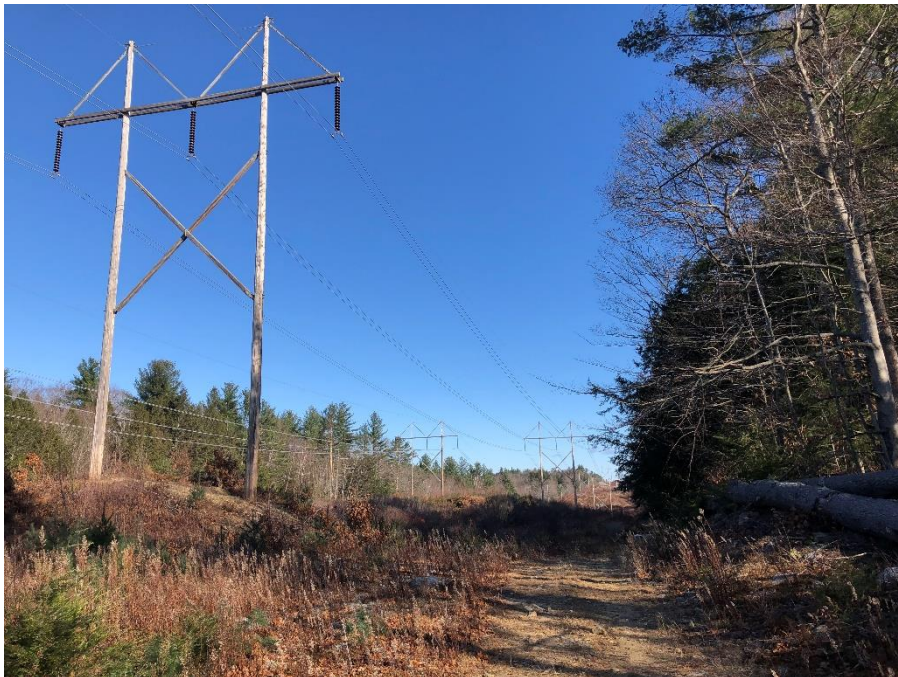
Photograph No. 16: Looking northerly at proposed structure replacement 391 structure 159 (right) with proposed access (left) in Deerfield.
