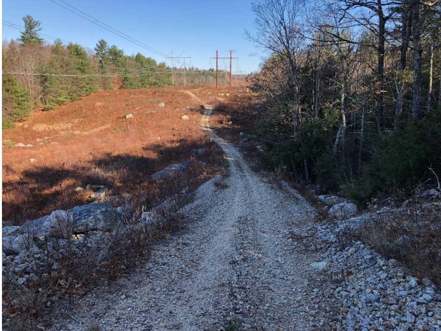
Photograph No. 29: Looking northeasterly at proposed existing access route between structures 154 & 153 on the 391 line in Northwood.
