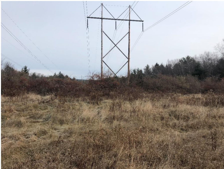
Photograph No. 38: Looking easterly at proposed structure replacement 391 structure 99 in Strafford.
