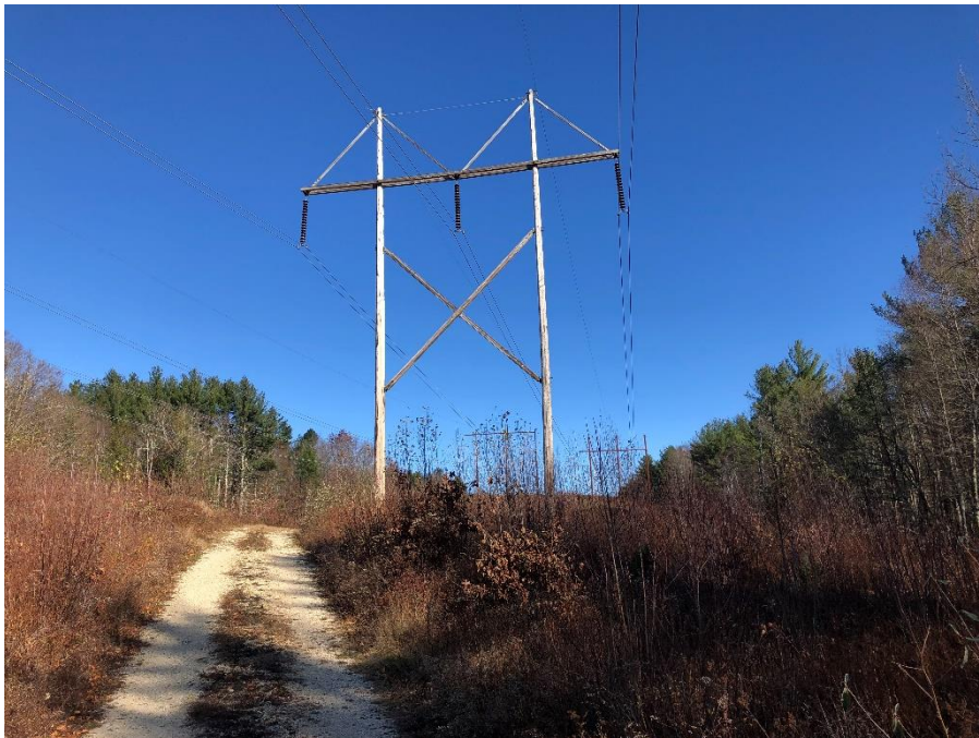
Photograph No. 34: Looking northeasterly at proposed existing access route towards 391 structure 150 in Northwood.
