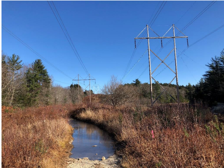
Photograph No. 21: Looking northeasterly at proposed access route (left) and proposed structure replacement 391 structure 157 (right) in Deerfield.
