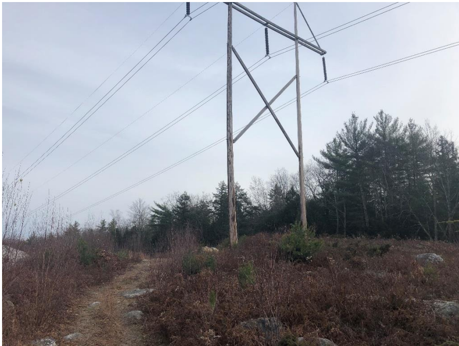
Photograph No. 46: Looking easterly at proposed work pad location adjacent to 391 Line Structure 97 Strafford.
