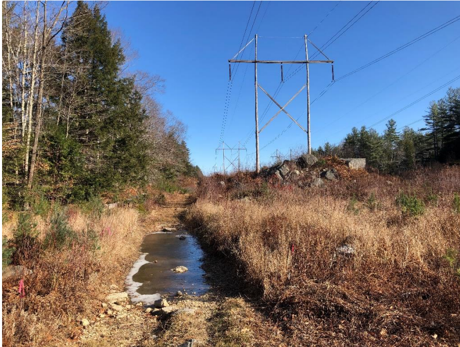
Photograph No. 7: Looking northwesterly at proposed structure replacement 385 structure 157 with proposed access route in Deerfield.
