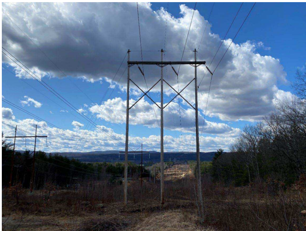
Photograph No. 10: Looking at proposed access and work pad location for N186 Structure 246.
