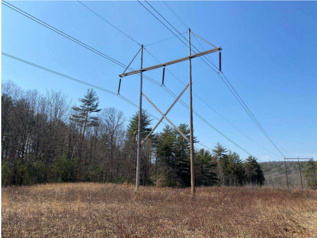
Photograph No. 23: Looking at proposed access and work pad location adjacent to 379 Structure 529.
