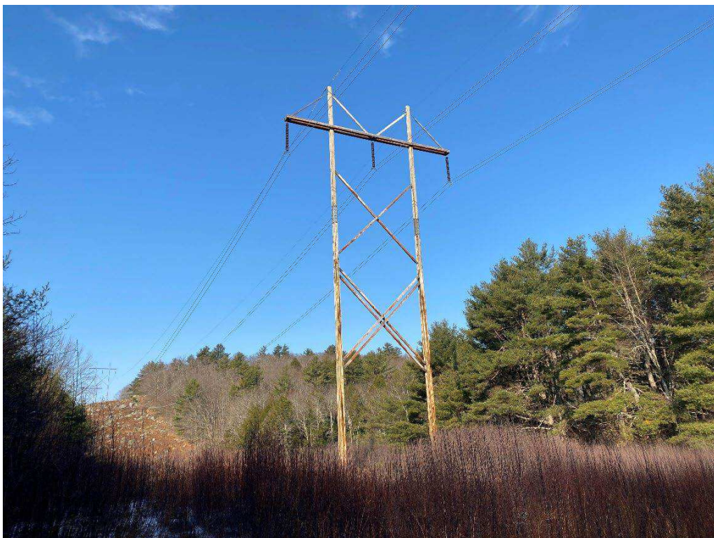
Photograph No. 34: Looking at proposed access and work pad location for 379 Structure 440.
