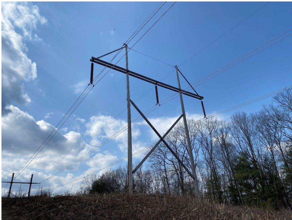
Photograph No. 18: Looking at proposed work pad location adjacent to 379 Structure 544.
