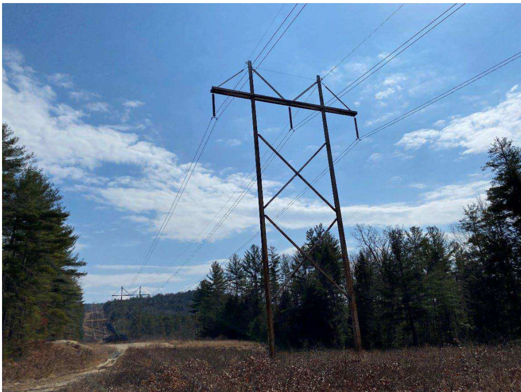
Photograph No. 24: Looking at proposed access and work pad location for 379 Structure 524.
