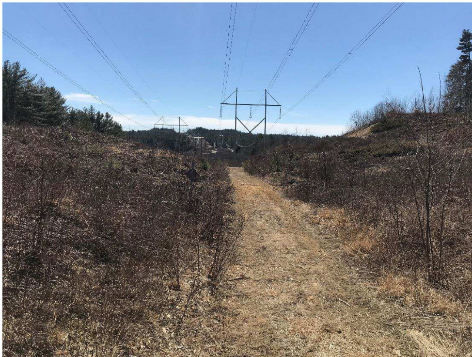
Photograph No. 10: Looking northerly toward 391 Structure 217 along existing access to be improved in Deerfield.
