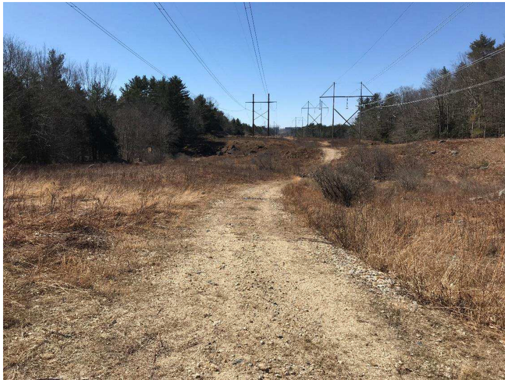
Photograph No. 12: Looking southwesterly toward 385 Structure 73 along existing access to be improved in Strafford.
