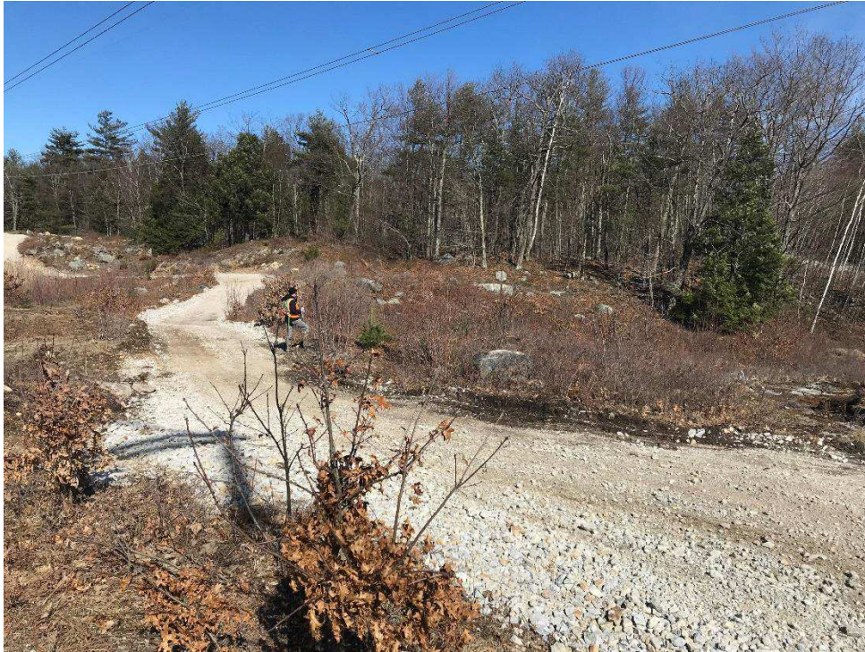
Photograph No. 7: Looking northerly at existing and improved access towards 391 Structure 301 in Chester.
