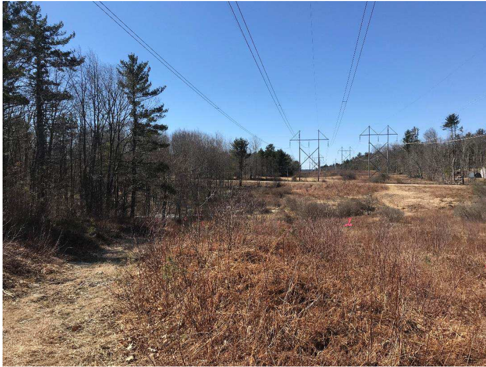
Photograph No. 13: Looking southwesterly toward Wetland SW-7 in Strafford. Temporary timber matting will be used to cross wetland areas.
