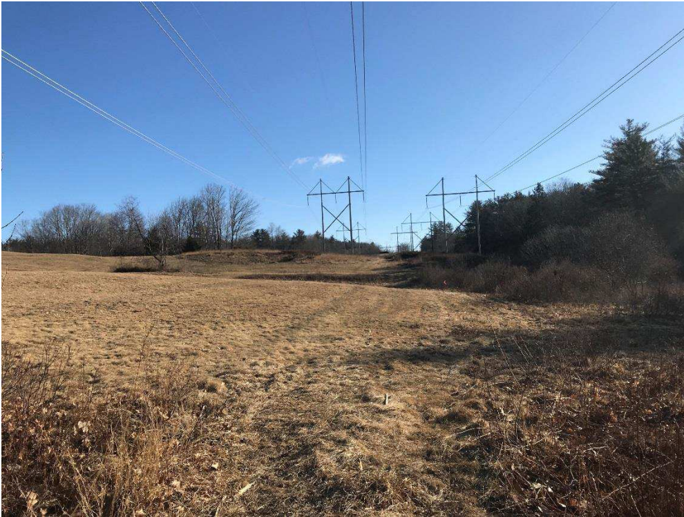
Photograph No. 19: Looking northeasterly toward 391 Structure 54 (right) and across open field where temporary upland matting will be utilized.
