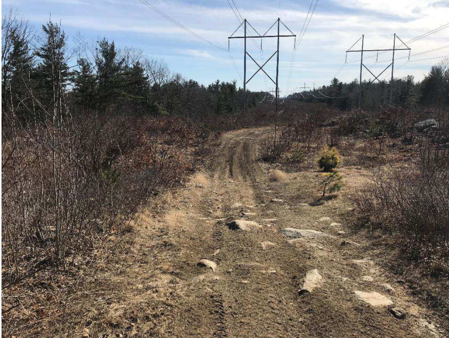
Photograph No. 5: Looking southwesterly at 391 Structure 305 at existing access to be improved in Chester.
