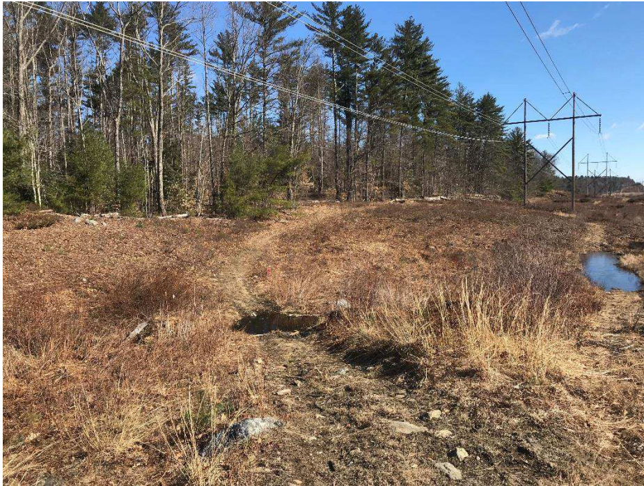
Photograph No. 17: Looking northerly toward proposed wetland crossing over Wetland RW-16 and toward 385 Structure 54 in Rochester.
