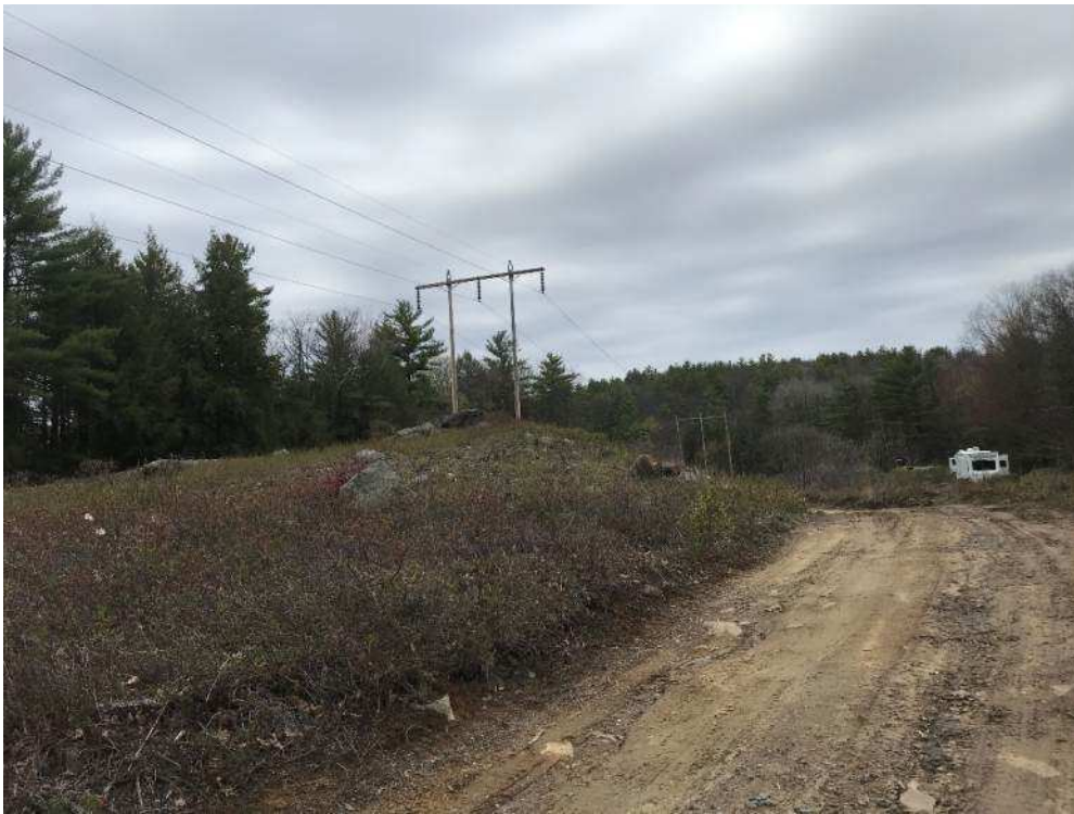
Photo 2: View north of existing structures 84 and 85. 5/3/21
