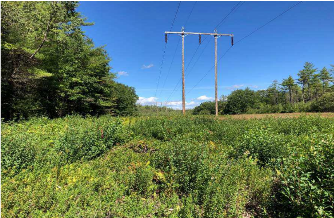
Photo 12: View northwest of Wetland FW-13 toward existing structure 38. 9/4/20
