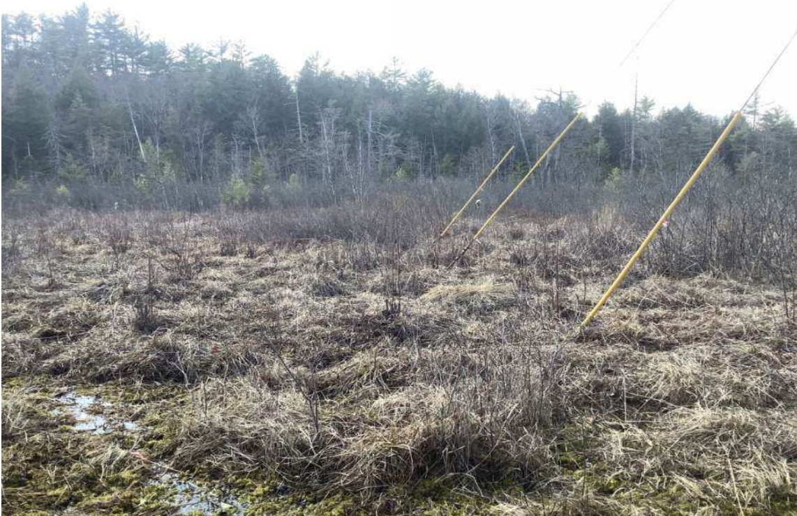
Photo 9: View west of Wetland FW-36 near existing structure 9. 4/14/21
