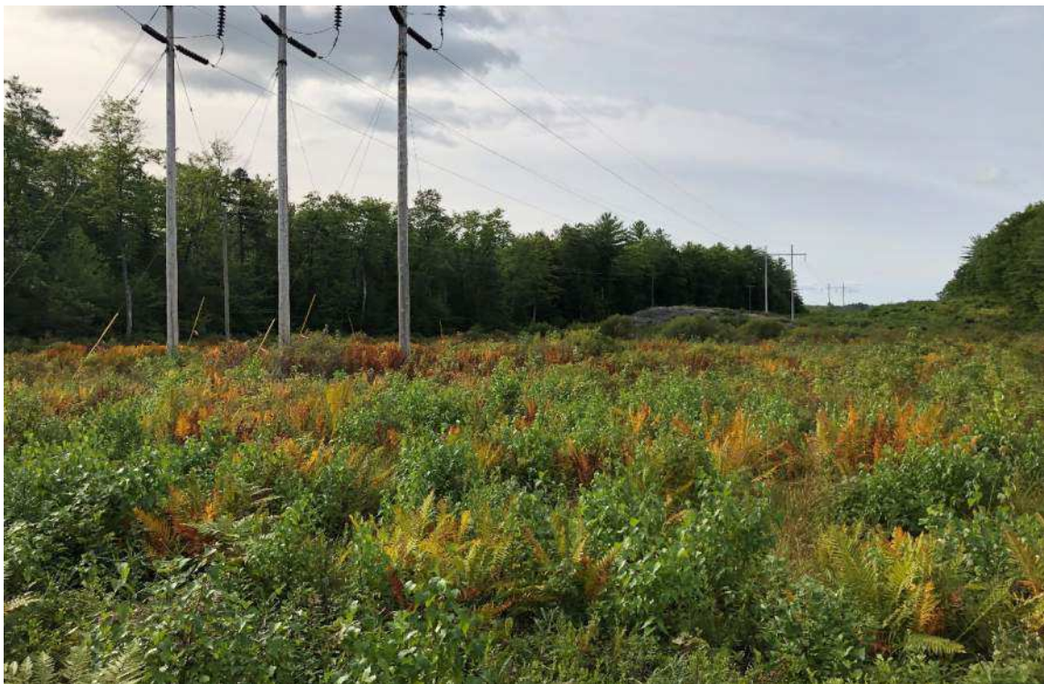
Photo 8: View southeast of Wetland FW-36 toward existing structure 8. 9/14/20
