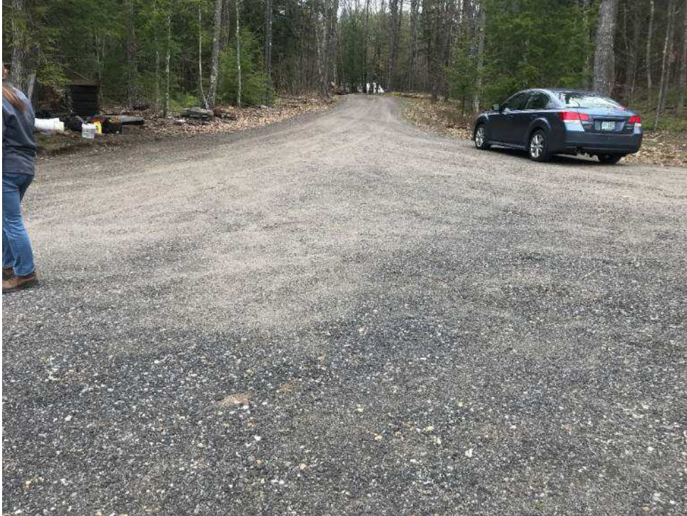
Photo 5: View east of an existing gravel drive toward existing structure 81. 5/3/21
