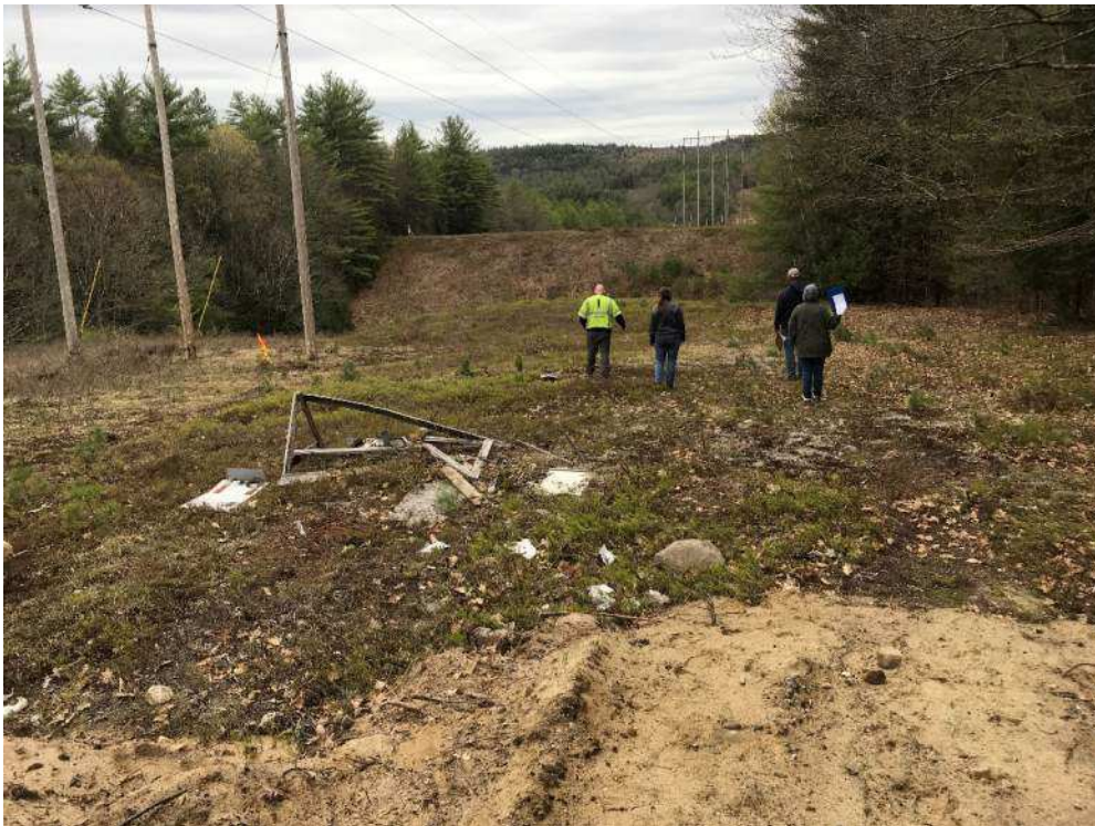
Photo 4: View south of existing structure 82 toward ex. structure 81 in the background. 5/3/21
