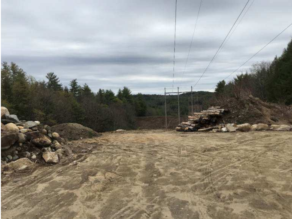
Photo 3: View south of existing structure 82/proposed structure 83. 5/3/21
