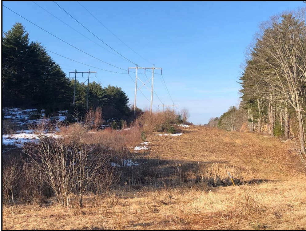
Photo 9: View west along transmission line ROW of Structures 82 and 96.
