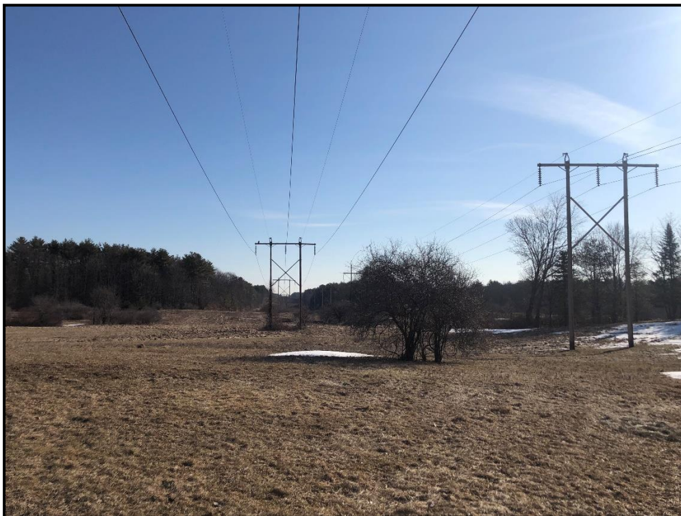
Photo 8: View east along transmission line ROW of Structures 112 and 97.
