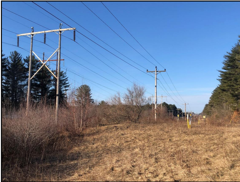
Photo 10: View west at Structure 91 and ROW access from Moulton Avenue.
