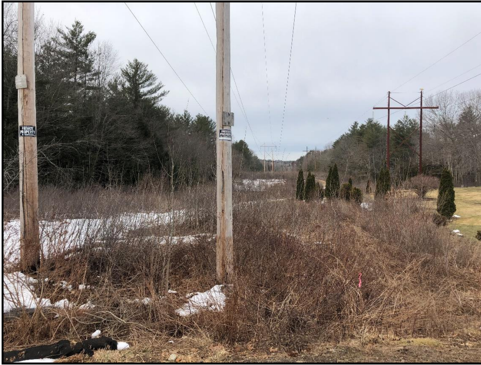
Photo 1: View west along transmission line ROW at the base of Structure 132 with Structure 150 in the background.
