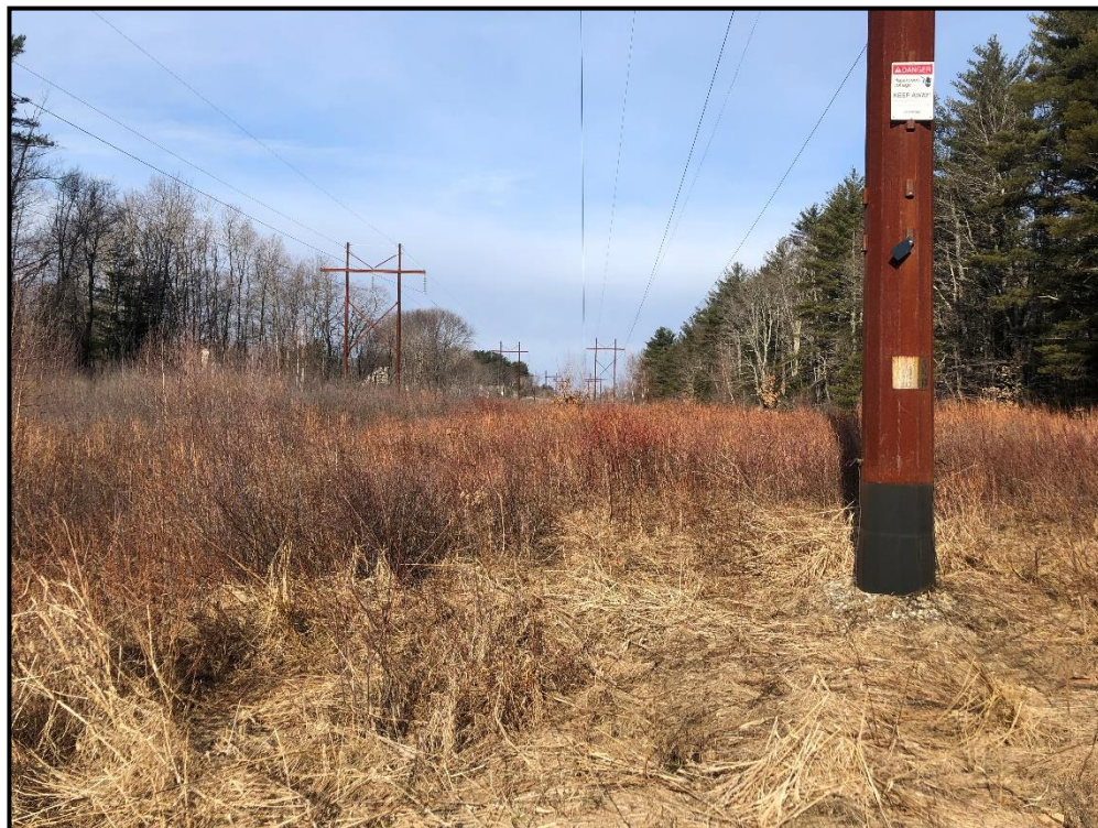
Photo 4: View west along transmission line ROW at the base of Structure 135.
