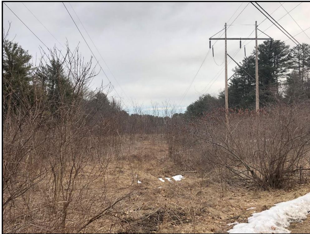
Photo 2: View east along transmission line ROW of Structure 131.
