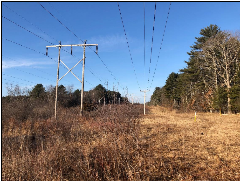
Photo 10: View west along transmission line ROW of Structure 93 and adjacent wetland.
