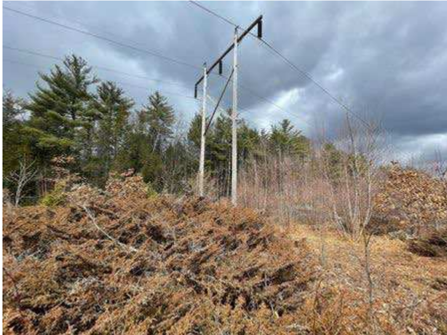
Photo 151. Str. 283 (R193 line) future work area, viewing north.
