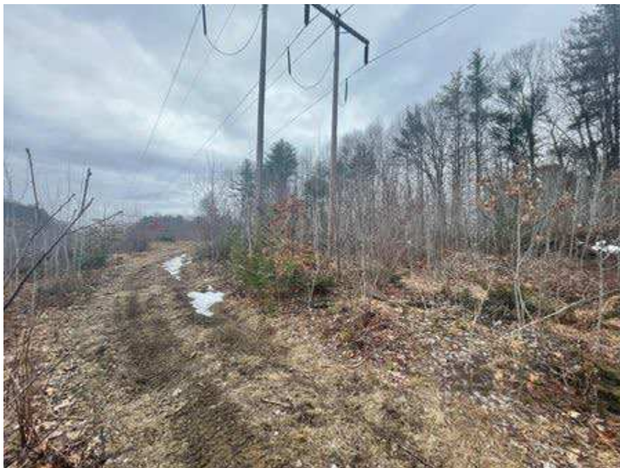
Photo 98. Str. 215 (H141 line) future work area, viewing southeast.
