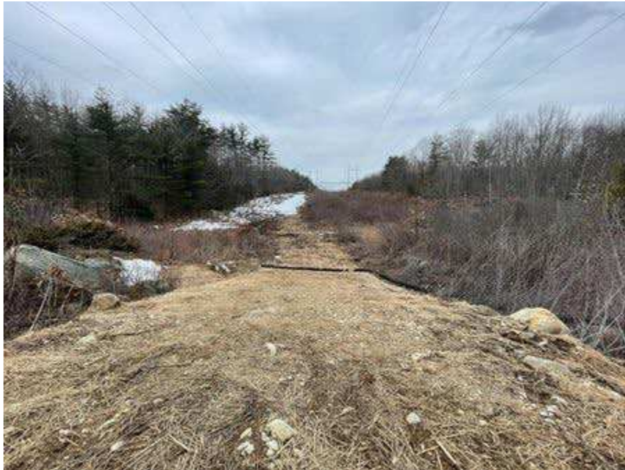
Photo 17. Proposed access route between Strs. 147 and 148 (H141 line), viewing west across stream and PSS1E wetland.
