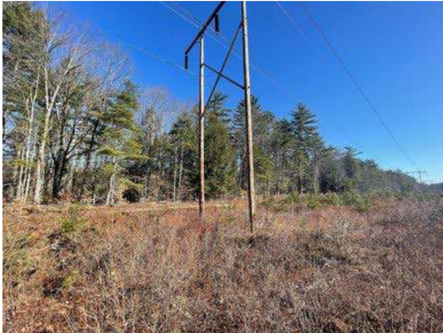
Photo 53. Str. 190 (A126 line) future work area, viewing northeast.
