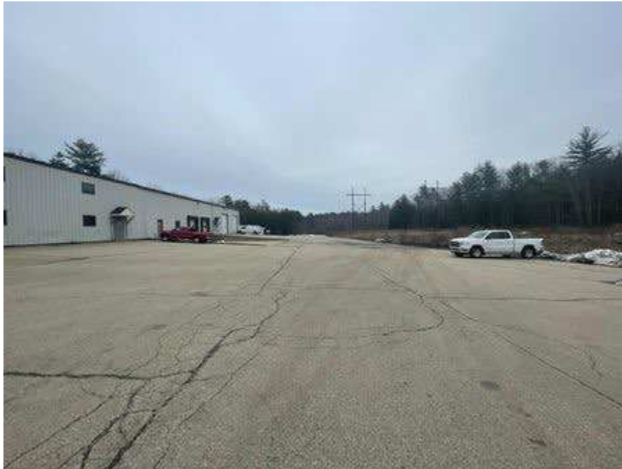
Photo 109. Proposed access route between Str. 219 (H141 line) and Route 125 across the Sunrise Farms Yogurt facility parking lot, viewing east.
