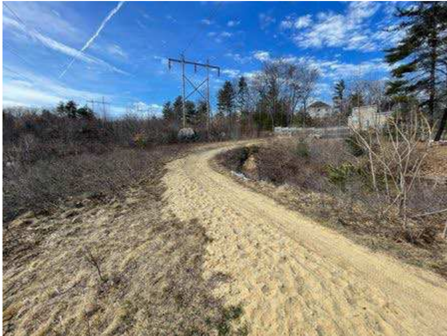
Photo 31. Proposed access route between Strs. 154 and 155 (H141 line), following existing sand/gravel trail, viewing northwest.
