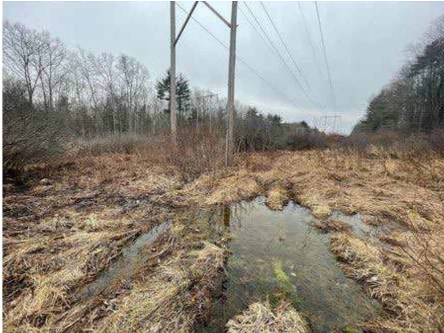
Photo 115. Str. 255 (R193 line) future work area, viewing southwest.
