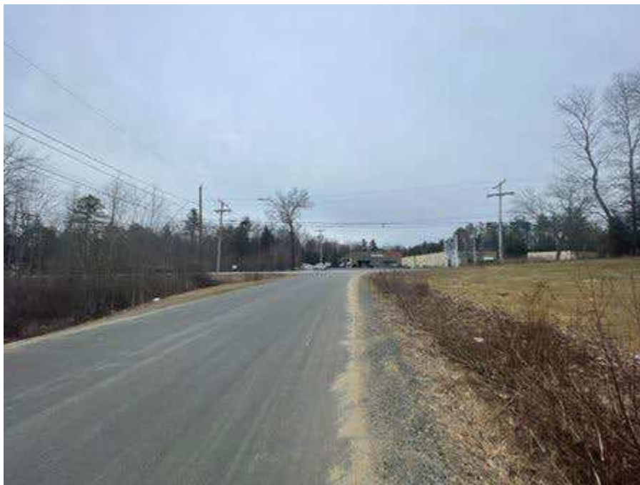
Photo 110. Representative view of the paved portion of the proposed access route between Str. 254 (R193 line) and Route 125, viewing east.
