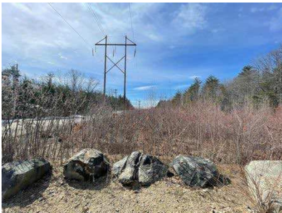
Photo 38. Proposed access route between dirt parking lot and Str. 157 (H141 line), viewing west.
