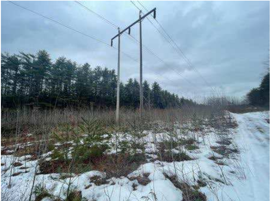
Photo 102. Str. 216 (H141 line) future work area, viewing northeast.
