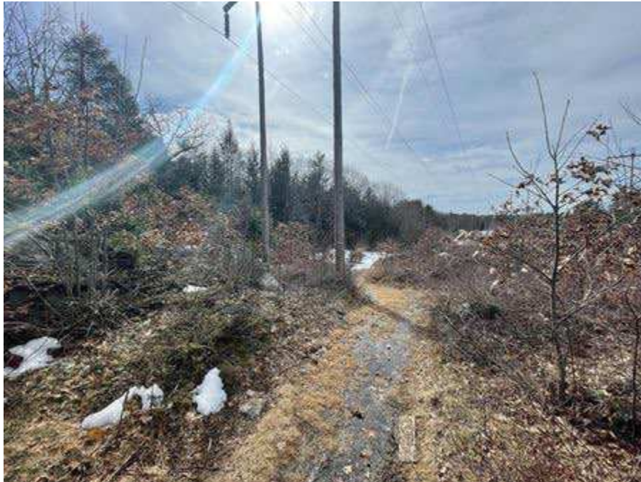
Photo 47. Str. 160 (H141 line) future work area, viewing southwest.
