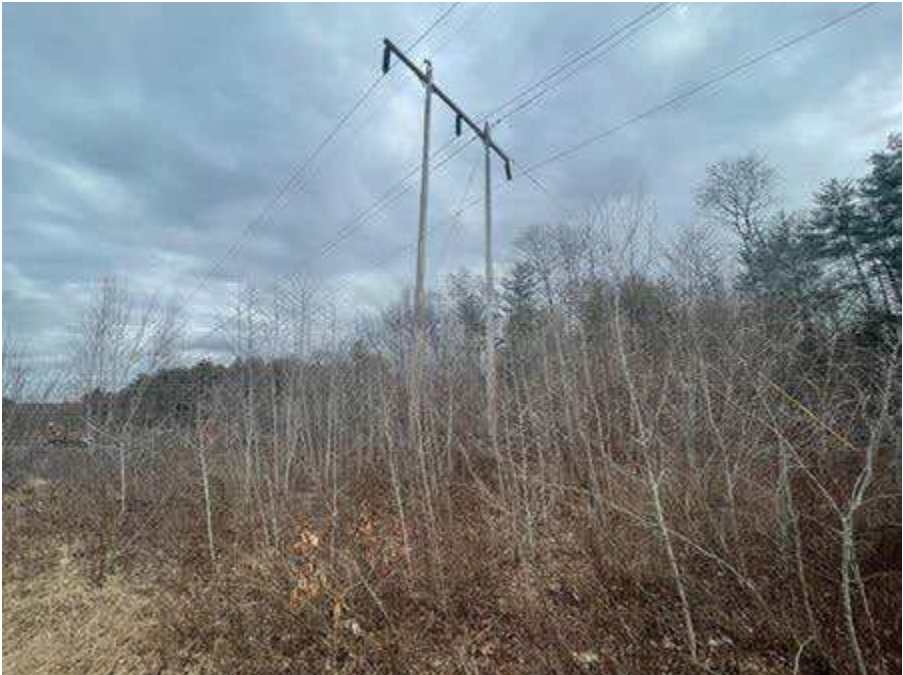
Photo 147. Str. 252 (H141 line) future work area, viewing east.
