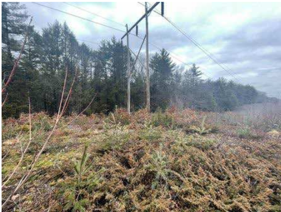
Photo 96. Str. 239 (A126 line) future work area, viewing northeast.
