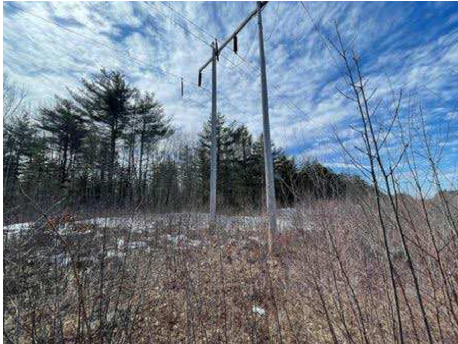
Photo 25. Str. 151 (H141 line) future work area, viewing southwest.
