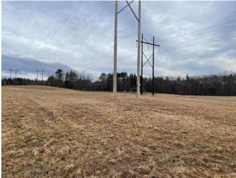
Photo 1. Str. 139 (H141 line) future work area, viewing north.
