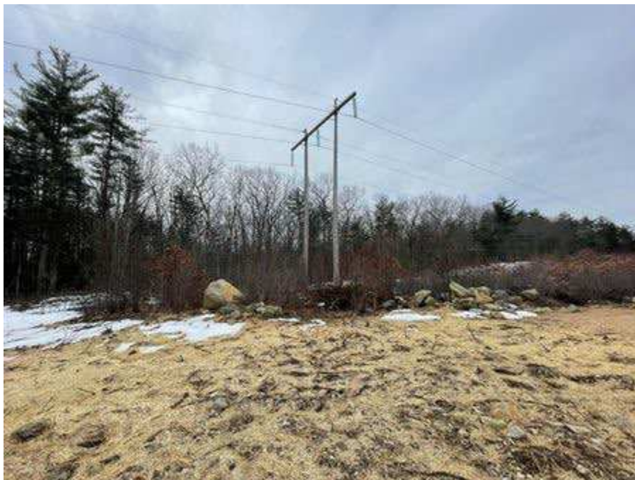
Photo 18. Str. 148 (H141 line) future work area, viewing southwest.
