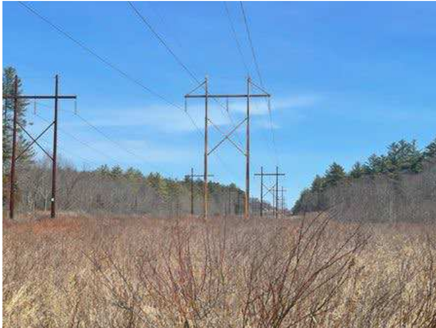
Photo 85. Proposed access route between Strs. 205 and 204 (H141 line), viewing northeast. Fencing prevented closer access to the future work area for Str. 204.
