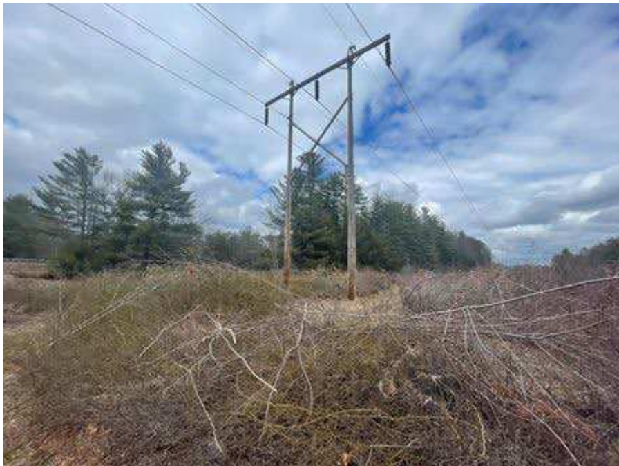
Photo 142. Str. 278 (R193 line) future work area, viewing north.
