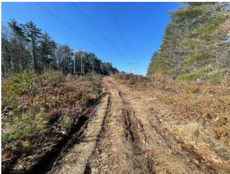
Photo 54. Proposed access route between Strs. 190 and 191 (A126 line), viewing west.
