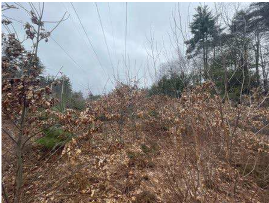
Photo 122. Proposed access route between Strs. 258 and 259 (R193 line), viewing west.
