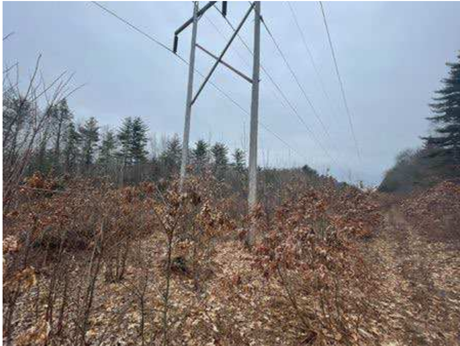
Photo 117. Str. 256 (R193 line) future work area, viewing southwest.
