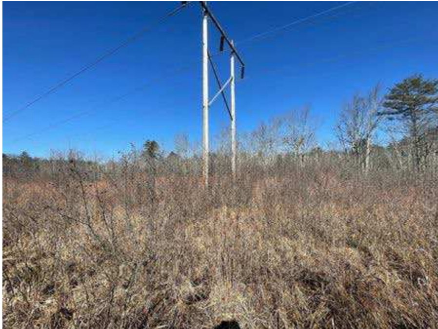
Photo 65. Str. 195 (A126 line) future work area, viewing northwest.
