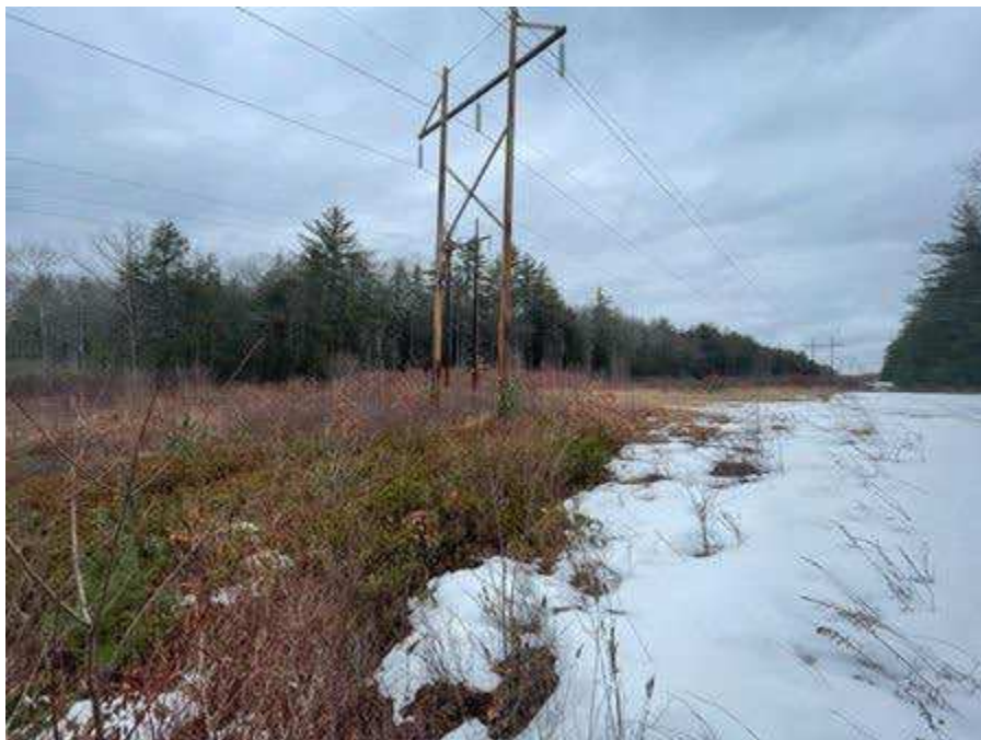
Photo 106. Str. 219 (H141 line) future work area, viewing northeast.
