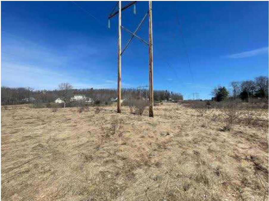
Photo 80. Str. 194 (H141 line) future work area, viewing northeast.
