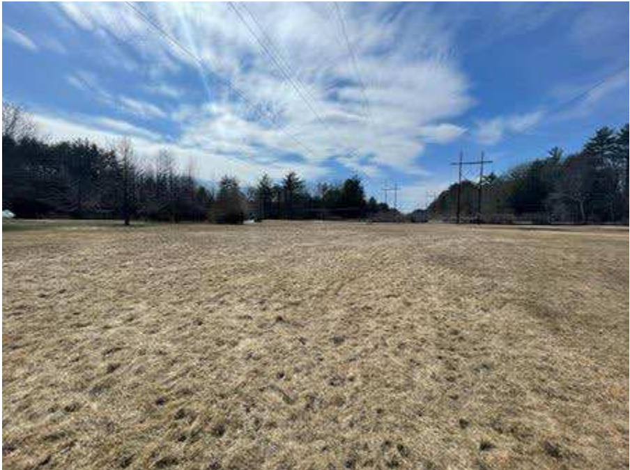
Photo 83. Proposed access route between Prescott Road and Str. 205 (H141 line), viewing southwest.
