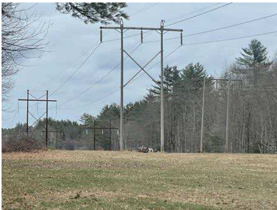
Photo 90. Str. 237 (A126 line) future work area, viewing east from behind the private electric fence.
