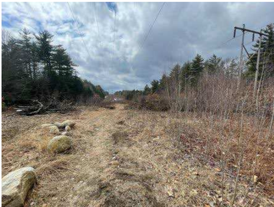
Photo 152. Proposed access route between Strs. 283 and 284 (R193 line), viewing west.
