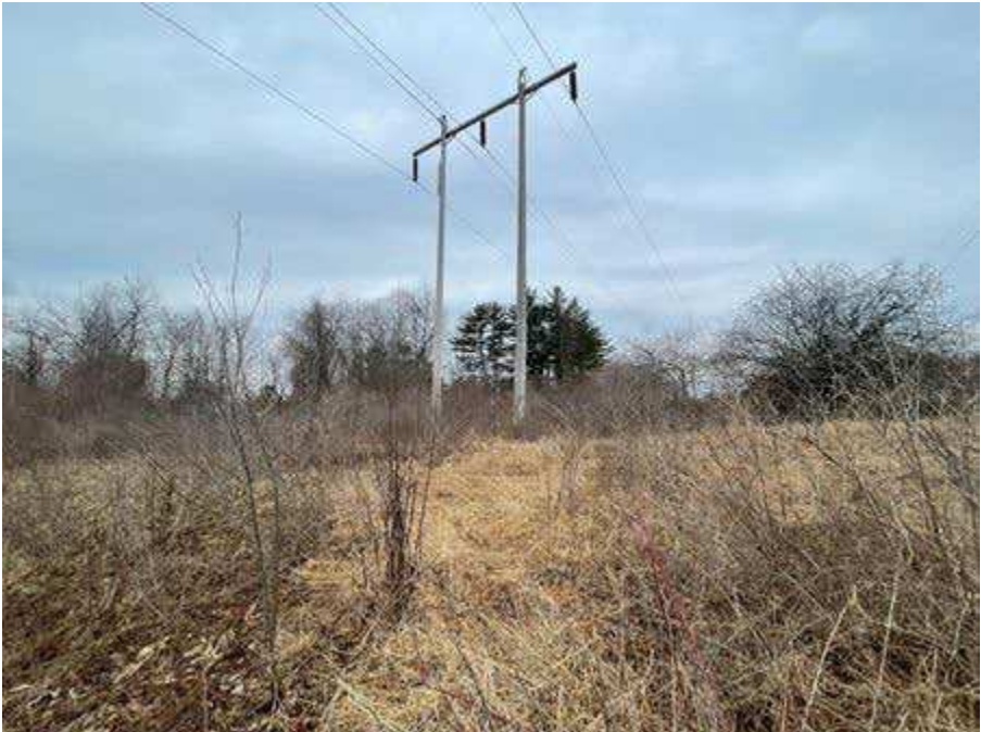
Photo 4. Str. 141 (H141 line) future work area, viewing west.
