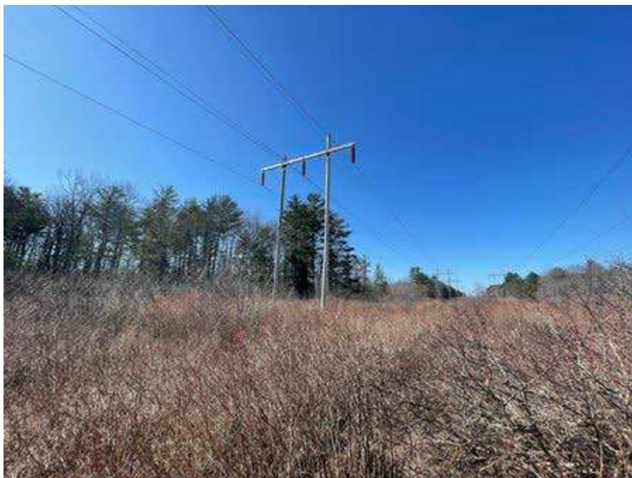
Photo 66. Str. 174 (H141 line) future work area, viewing southwest.
