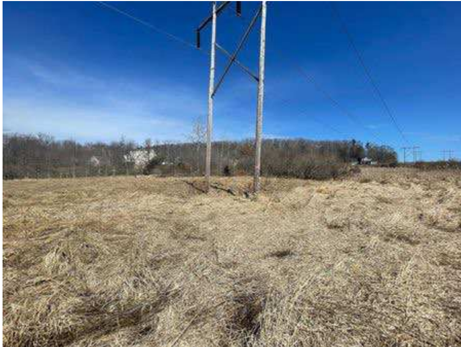
Photo 81. Str. 217 (A126 line) future work area, viewing northeast.
