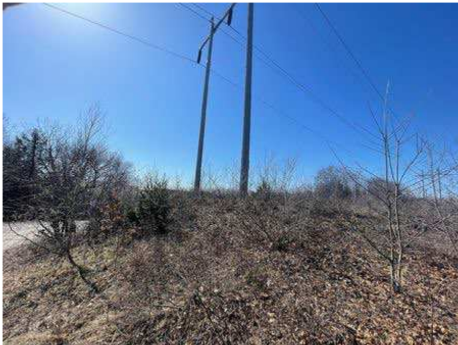
Photo 68. Str. 181 (H141 line) future work area, viewing southwest.
