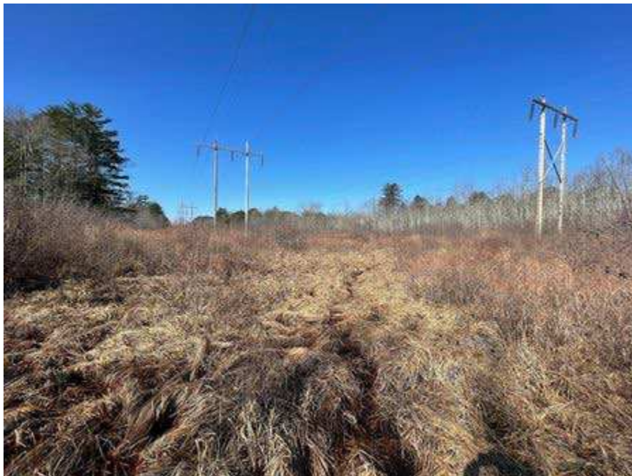
Photo 64. Proposed access route between Str. 193 and 194 (A126 line) branches to right, viewing west.
