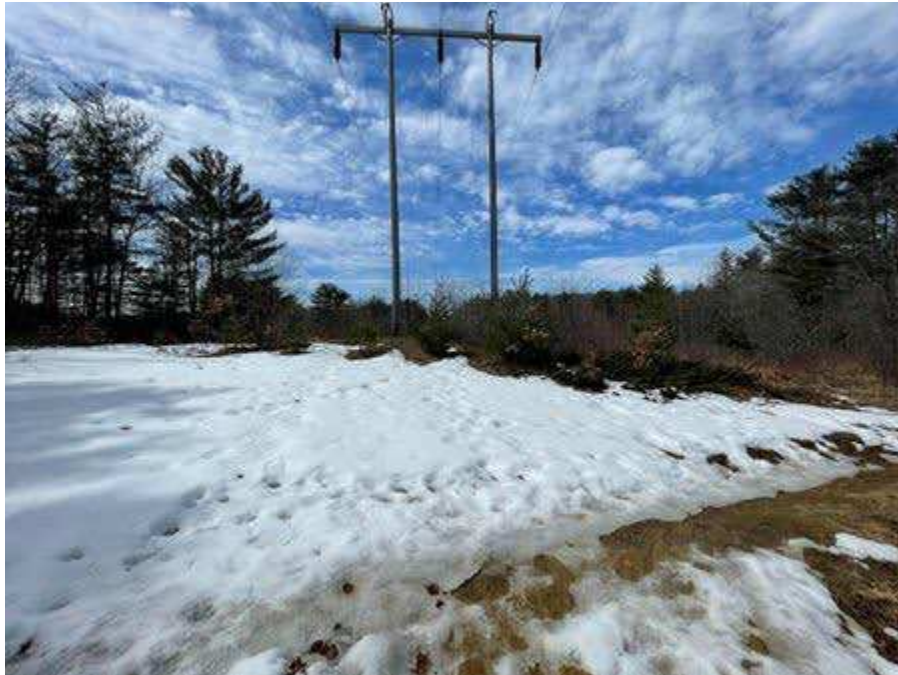
Photo 29. Str. 153 (H141 line) future work area, viewing west.
