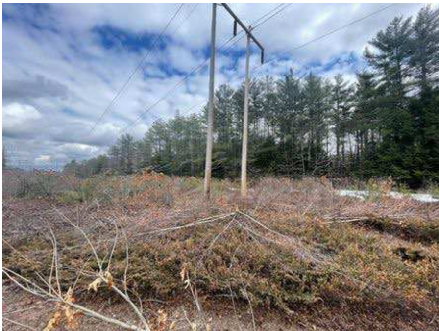
Photo 144. Str. 251 (H141 line) future work area, viewing east.
