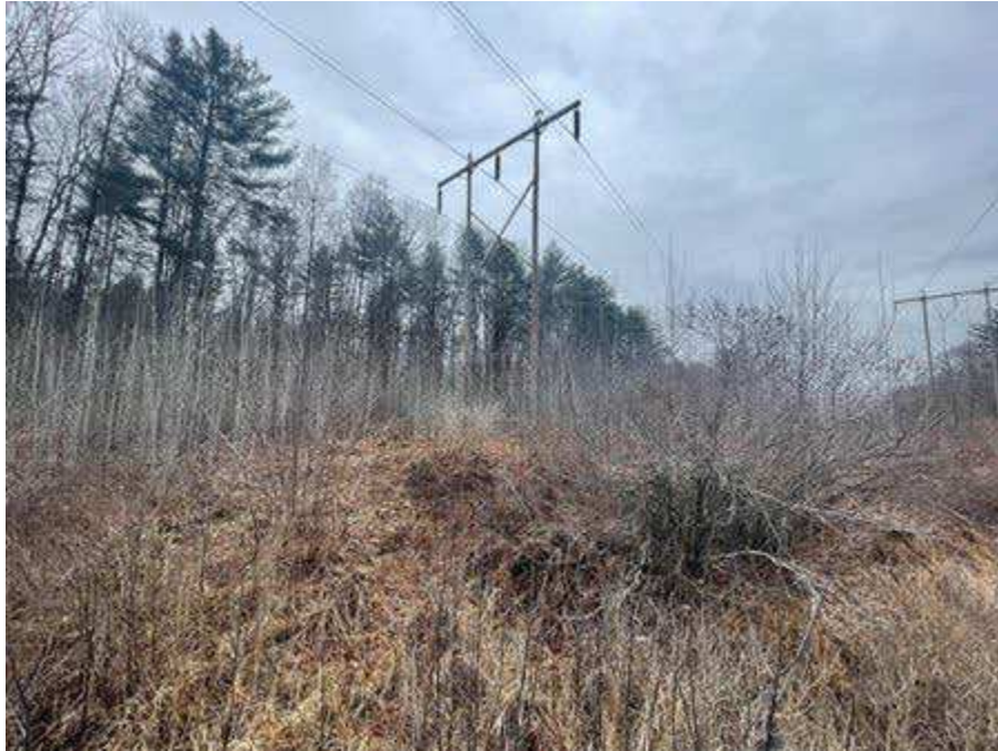
Photo 91. Str. 238 (A126 line) future work area, viewing northeast.
