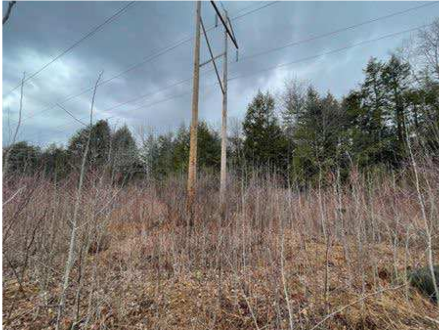
Photo 153. Str. 284 (R193 line) future work area, viewing northwest.
