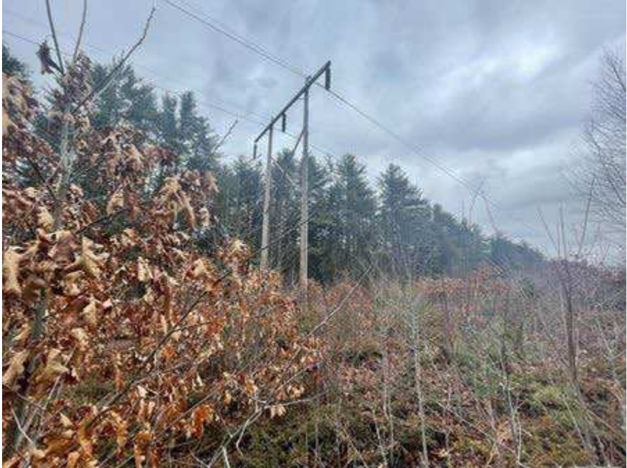
Photo 101. Str. 240 (A126 line) future work area, viewing northeast.
