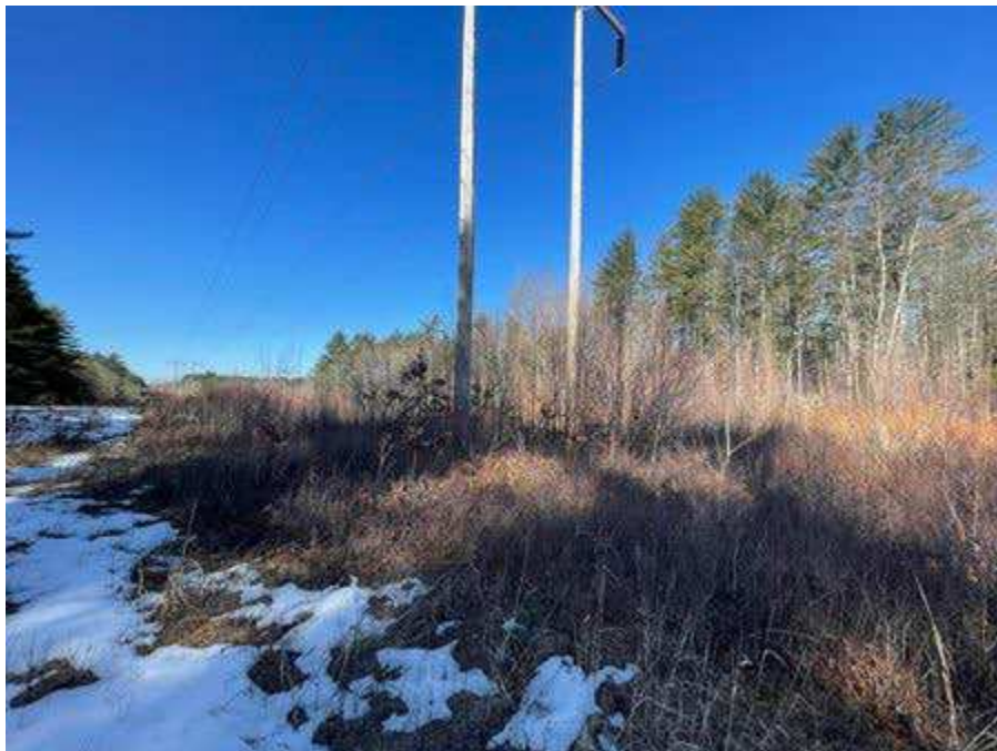
Photo 60. Str. 193 (A126 line) future work area, viewing northwest.
