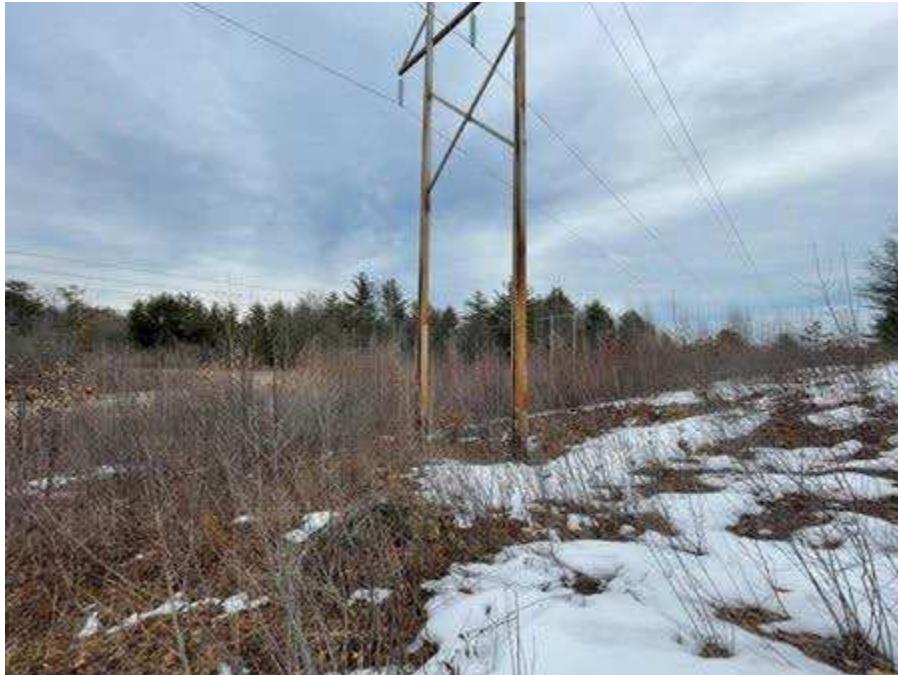
Photo 7. Str. 143 (H141 line) future work area, viewing northeast.
