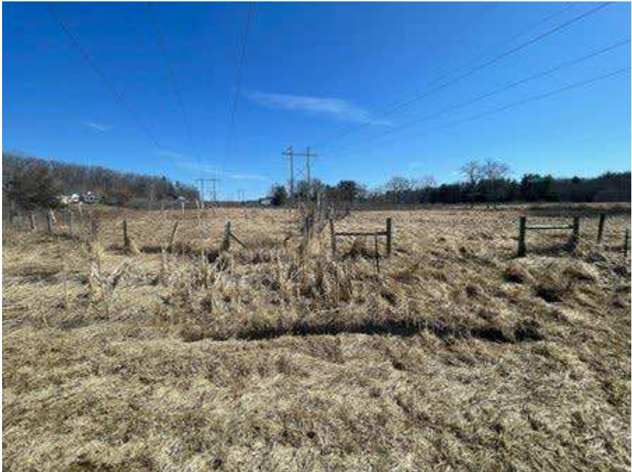
Photo 79. Proposed access road to Str. 194 of the H141 line and Str. 217 of the A126 line, viewing east.
