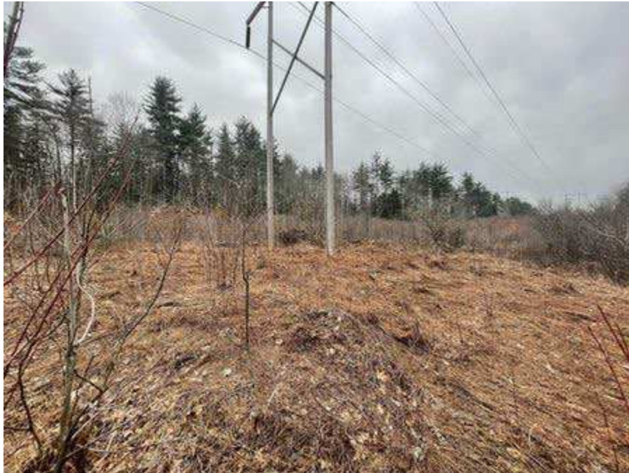
Photo 123. Str. 259 (R193 line) future work area, viewing southwest.
