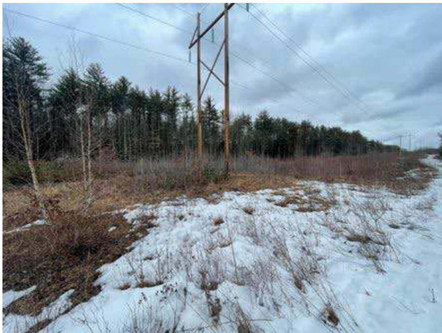
Photo 104. Str. 217 (H141 line) future work area, viewing northeast.
