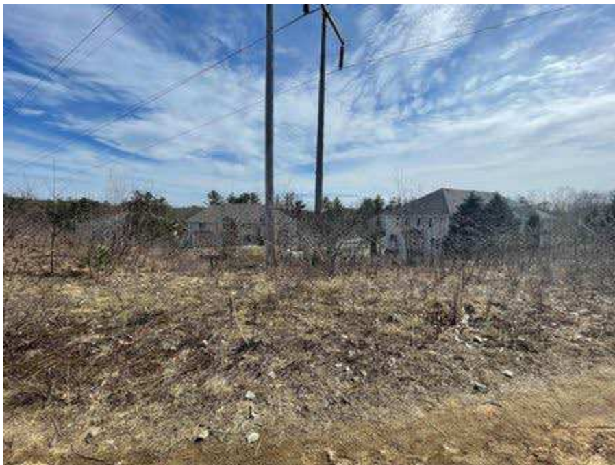
Photo 32. Str. 155 (H141 line) future work area, viewing south.
