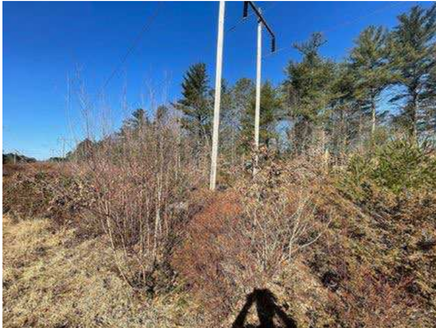
Photo 55. Str. 191 (A126 line) future work area, viewing northwest.
