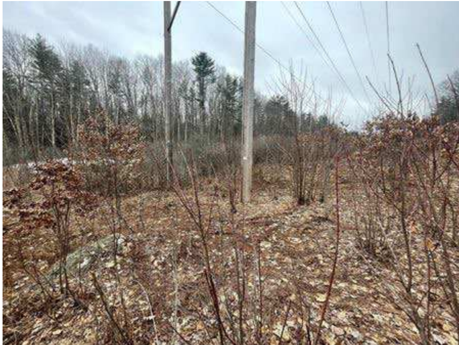
Photo 119. Str. 257 (R193 line) future work area, viewing northeast.
