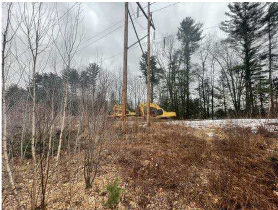
Photo 128. Str. 235 (H141 line) future work area, viewing southeast.
