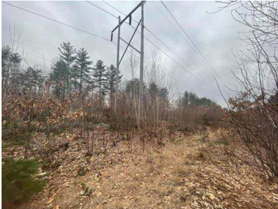
Photo 125. Str. 260 (R193 line) future work area, viewing southwest.
