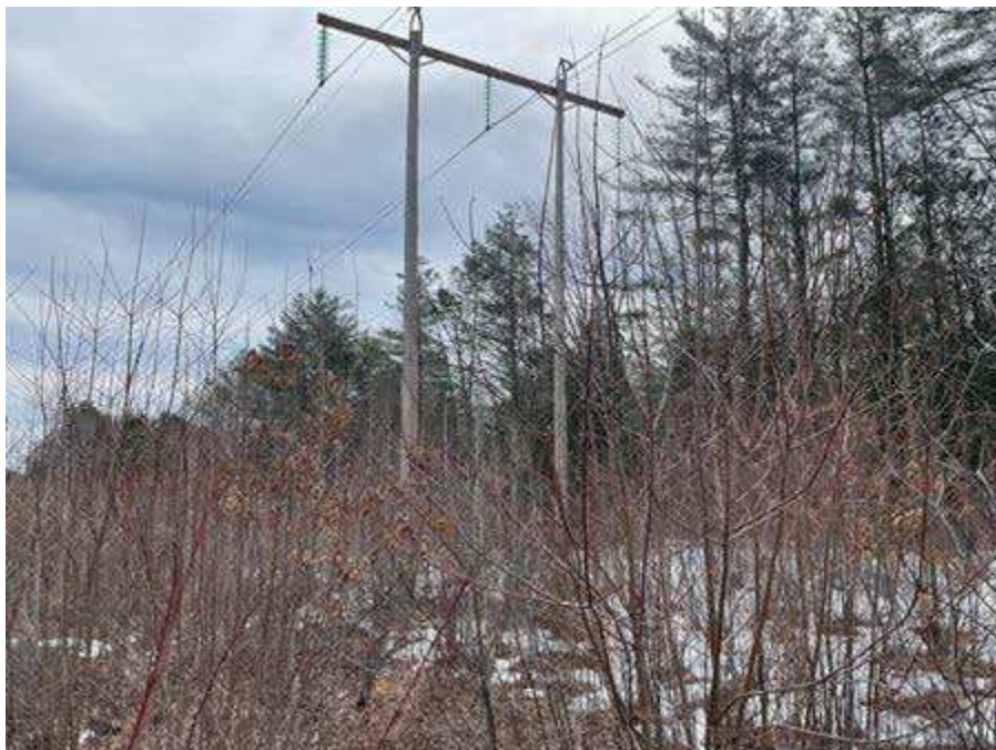
Photo 10. Str. 144 (H141 line) future work area, viewing southeast.
