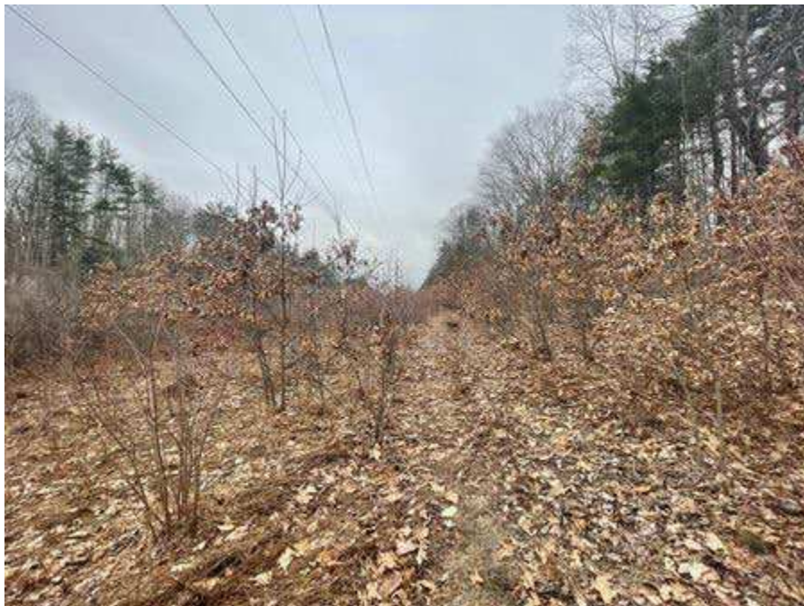
Photo 120. Proposed access route between Strs. 257 and 258 (R193 line), viewing west.
