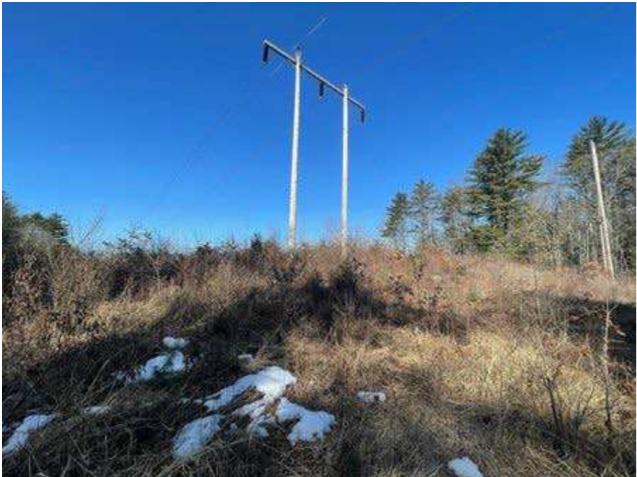
Photo 62. Str. 194 (A126 line) future work area, viewing northwest.
