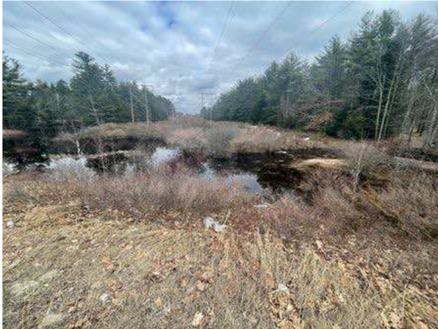
Photo 145. Proposed access route with matted wetland/stream crossing between Danville Road and Strs. 278 (R193 line) 251 (H141 line), viewing northeast.
