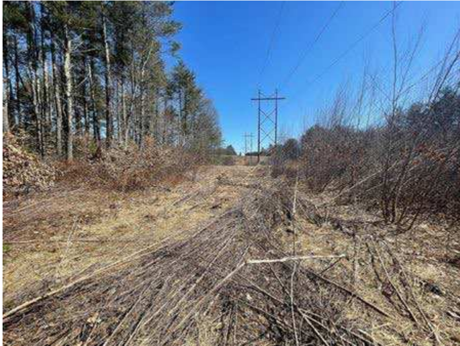
Photo 75. Proposed access route between Strs. 179 and 178 (H141 line), viewing east.
