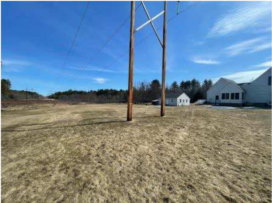
Photo 84. Str. 205 (H141 line) future work area, viewing southeast.
