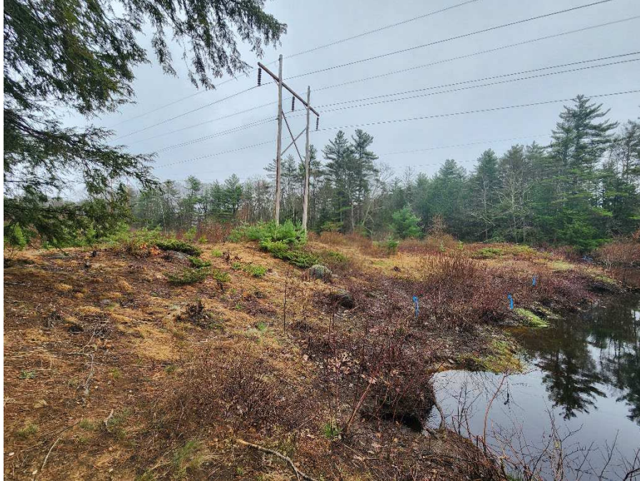
Photo 141. Bank of the Exeter River FRS01 adjacent the Str. 277 (R193 line) future work area, viewing southeast.
