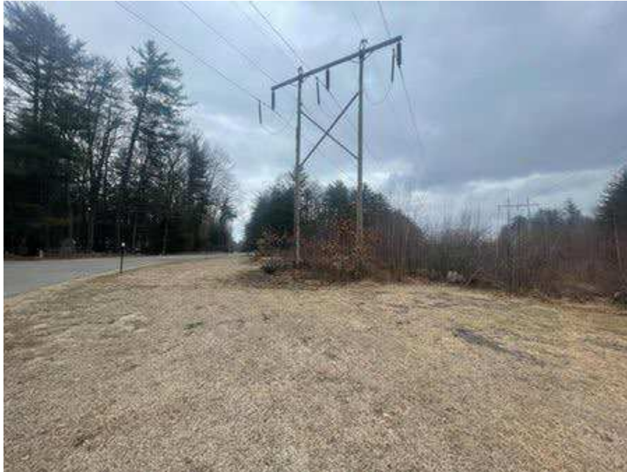
Photo 149. Str. 282 (R193 line) future work area, viewing northeast.
