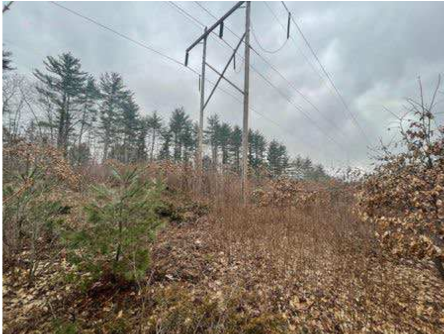
Photo 127. Str. 261 (R193 line) future work area, viewing southwest.
