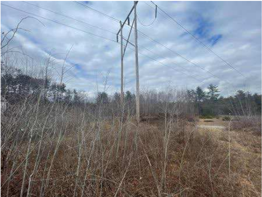
Photo 148. Str. 279 (R193 line) future work area, viewing north.
