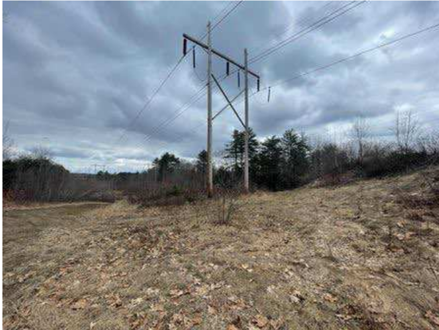
Photo 135. Str. 275 (R193 line) future work area, viewing east.
