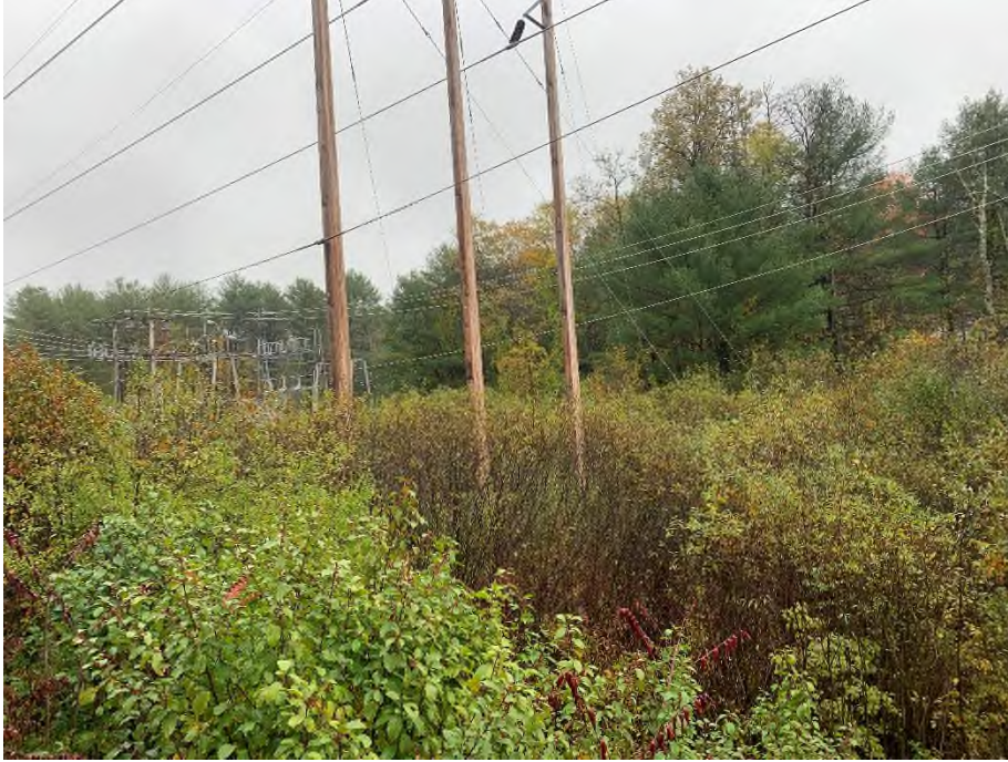
Photograph No. 53: Looking easterly at proposed pad location at Structure 72.
