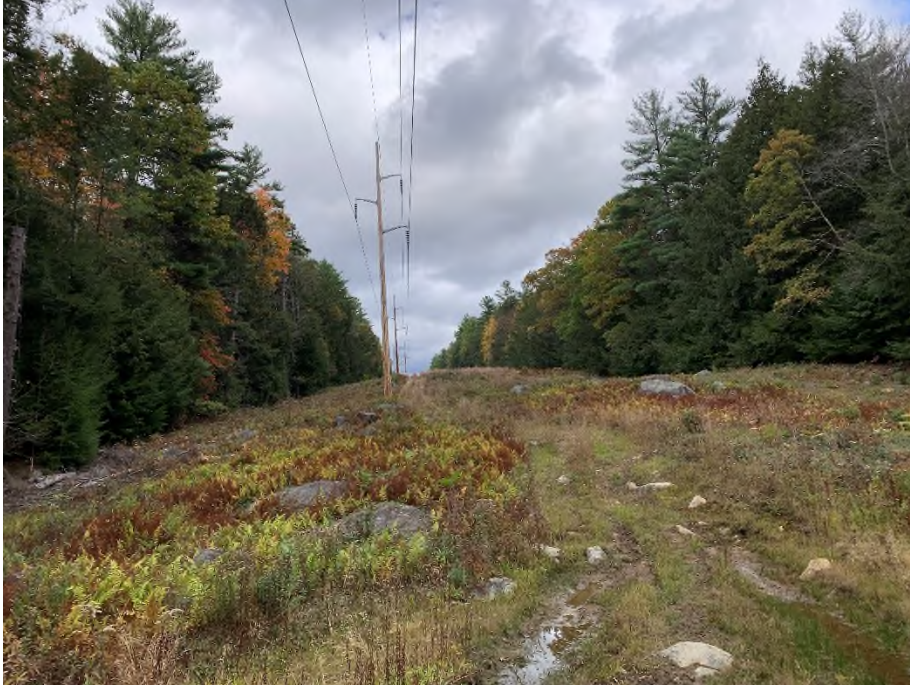
Photograph No. 27: Looking northerly at proposed access to Structure 44.
