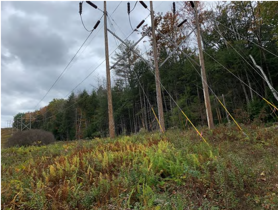
Photograph No. 14: Looking westerly at proposed pad location at Structure 32.
