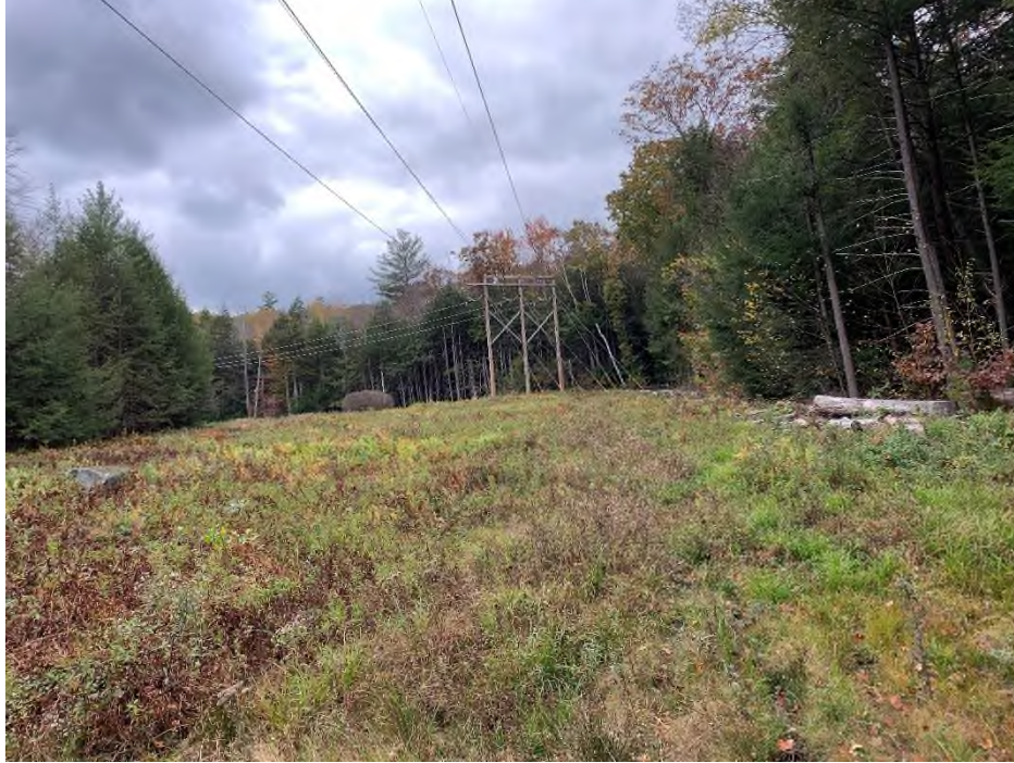
Photograph No. 13: Looking southwesterly at proposed access to Structure 32.
