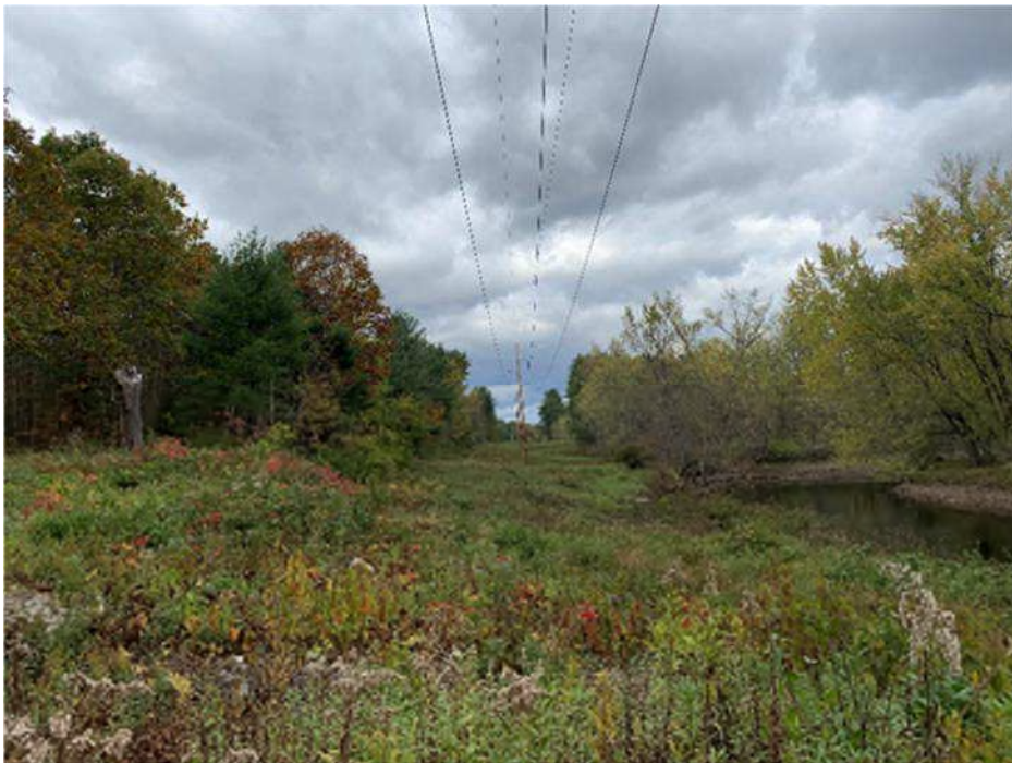
Photograph No. 8: Looking northerly at proposed access to Structure 28
