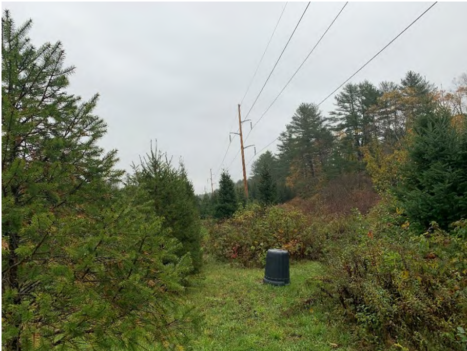
Photograph No. 36: Looking northeasterly at proposed access to Structure 60.
