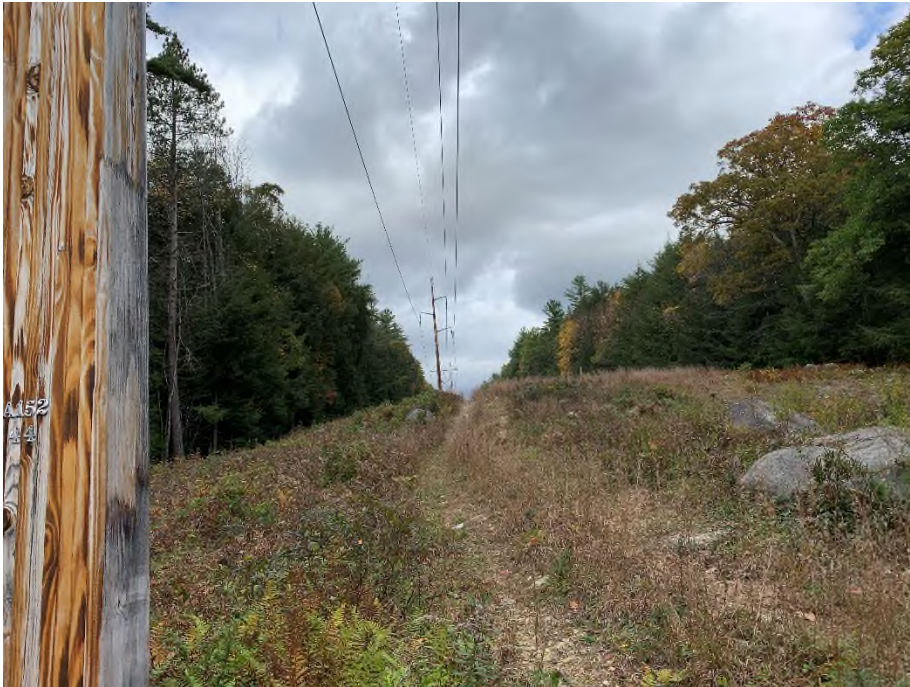
Photograph No. 26: Looking northerly at proposed access and pad location adjacent to Structure 44.
