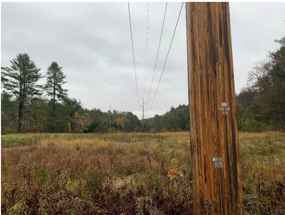
Photograph No. 34: Looking northeasterly at proposed pad location at Structure 58.
