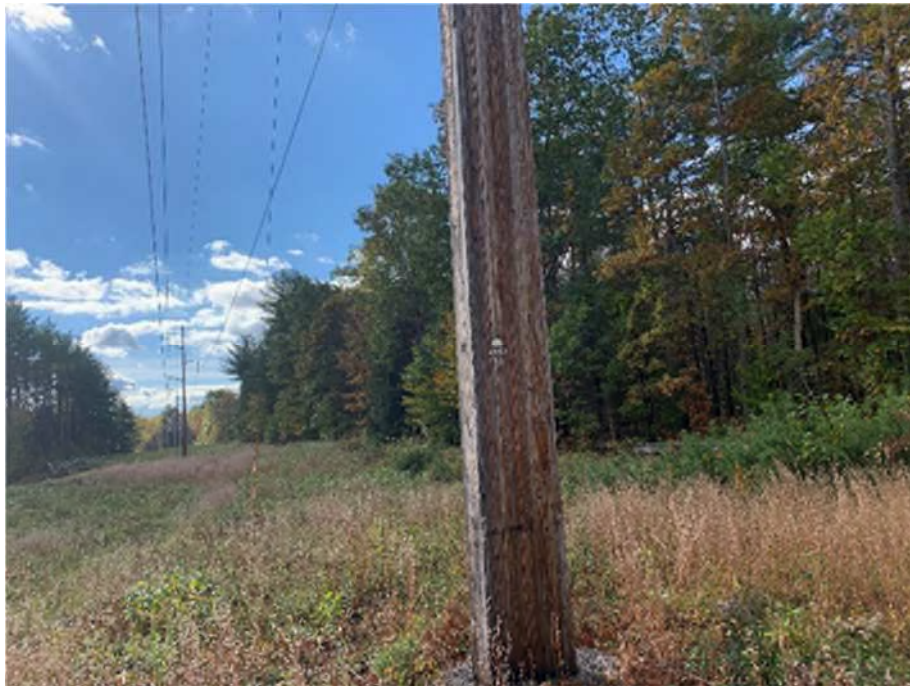
Photograph No. 4: Looking southerly at proposed pad location for Structure 25.
