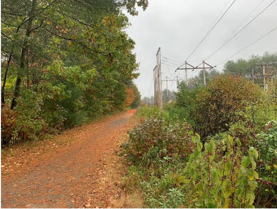
Photograph No. 51: Looking northeasterly at proposed access to Structures 70, 70A, 70B, & 71.
