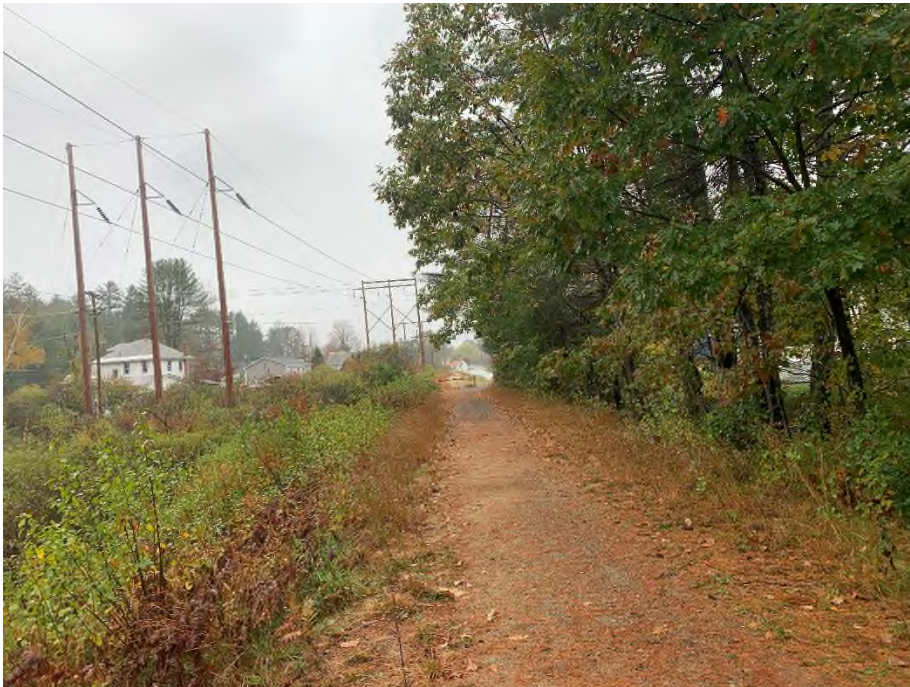
Photograph No. 52: Looking southwesterly at proposed access to Structure 72.
