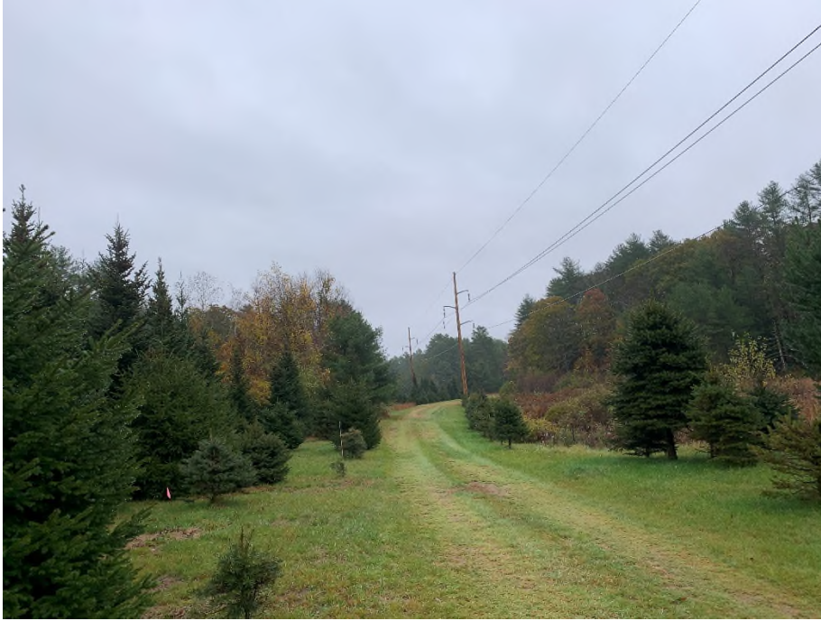
Photograph No. 31: Looking northeasterly at proposed access to Structure 56.
