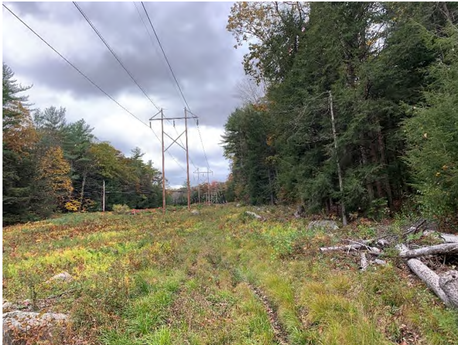
Photograph No. 10: Looking southwesterly at proposed access to Structure 30.
