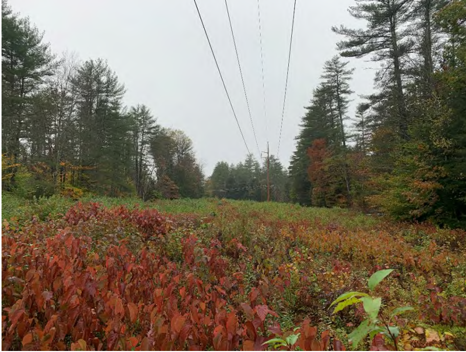
Photograph No. 41: Looking southwesterly at proposed access to Structure 65.
