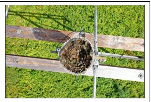
Structure 286 – Top rot, hollow at pole top
