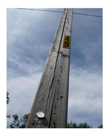
Side Crack – S188 Line, Structure #49
