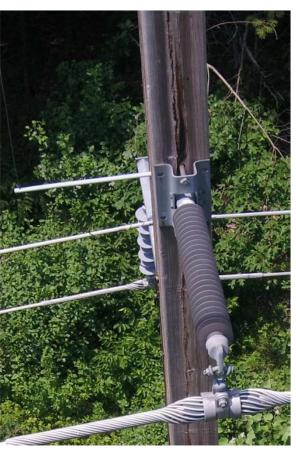
Side Crack – V191 Line, Structure #13
