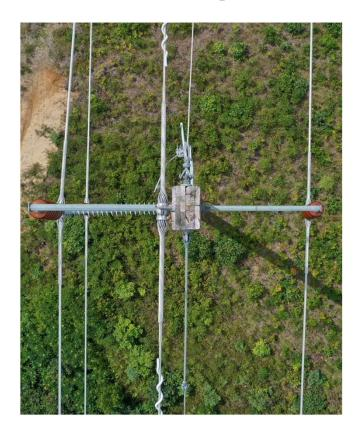
Pole Top Cracking – A152 Line, Structure #46
