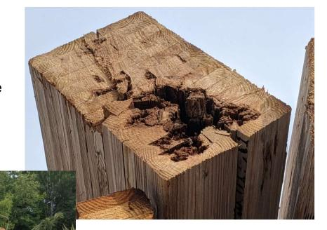
Above: G128 Line – Slide Cracking, Rot and Insect Damage
