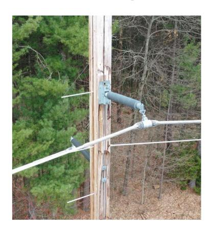
Cracking Laminate Structure – V191 Line, Structure #47
