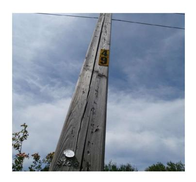
Side Crack – S188 Line, Structure #49
