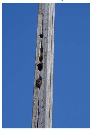
Woodpecker Damage and Cracking – S188 Line, Structure #52
