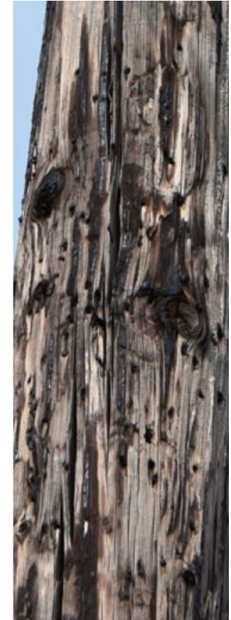
Pole Breaks and Woodpecker Damage – Line 456-522, Structure #54
