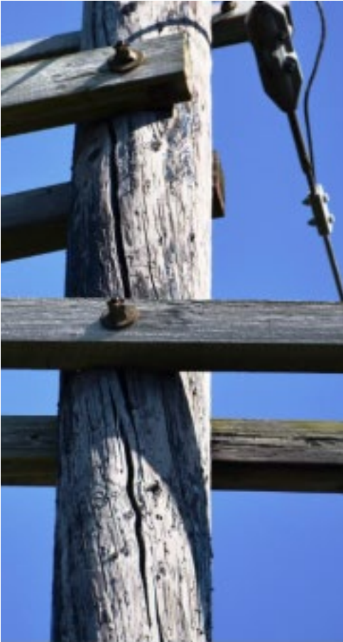
Pole Splits – Line 342-603, Structure #83
