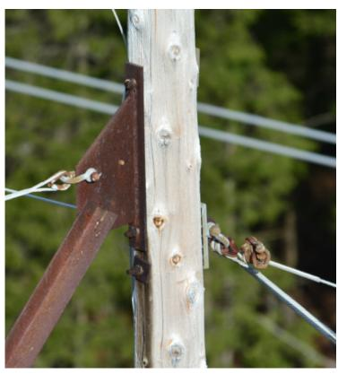
348 Line – CT Shield Wire Disconnected
