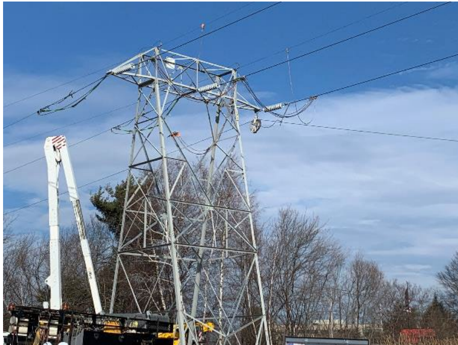
ACCC installation on S145 / T146 Line Wakefield, MA Larger pulling block and shallow line angle used
