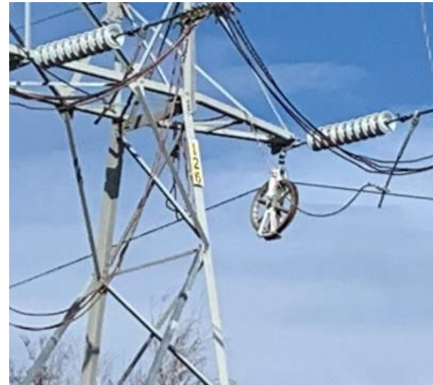
ACCC installation on S145 / T146 Line Wakefield, MA Larger pulling block and shallow line angle used
