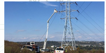
Figure A-38. Tower reconductoring.
