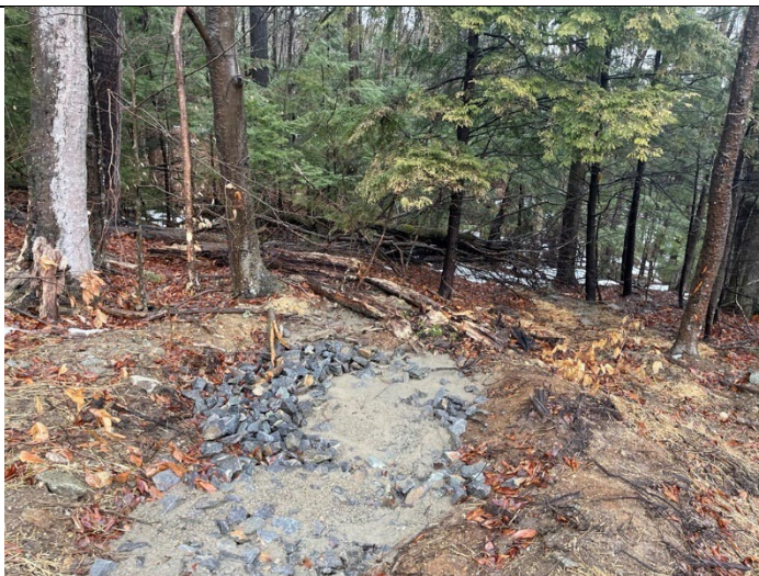
Looking northeast at a sediment trap between Structures 119 to 120 off Mount Israel Road, Sandwich. GZA recommends removal of sediment buildup.
