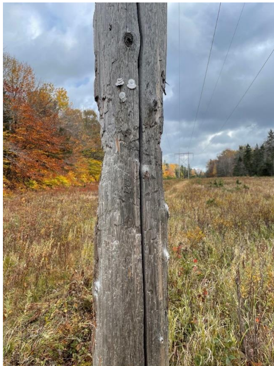
Photograph No. 10: Looking at bear damage to Structure 110.
