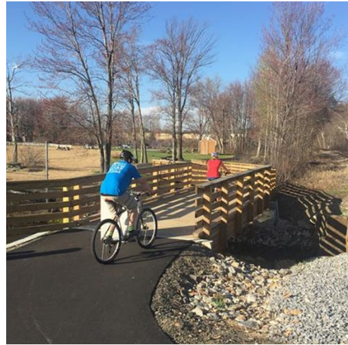
Figure 5: Existing Trail Segment
