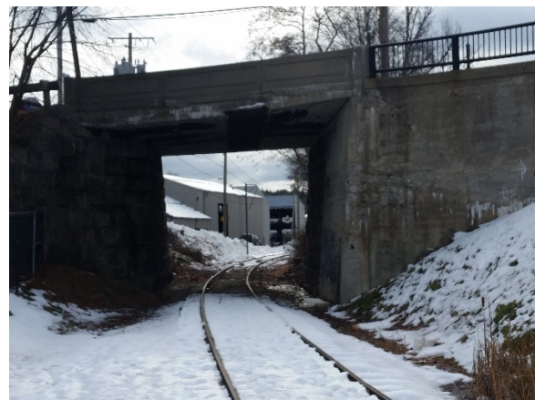
The narrow rail corridor below Route 3 precludes the rail-with-trail alternative to continue directly to Weirs Beach and may require an at-grade crossing of the State highway above the rail corridor.
