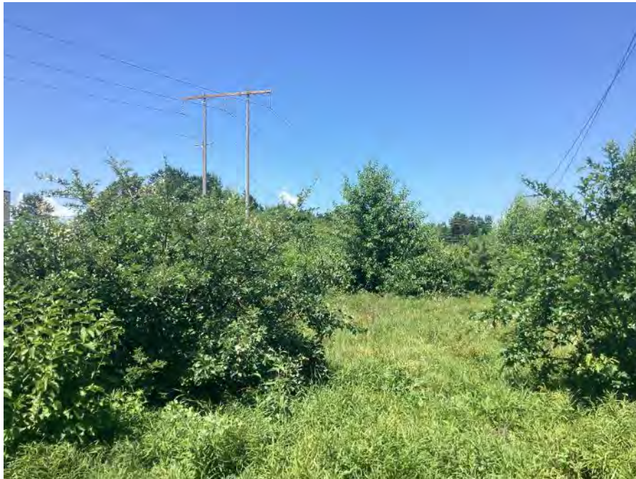
Photo 11. Louden Road to Soucook River Segment: shrub-dominated ROW, view to the west to structure 88. Stantec. July 19, 2022.
