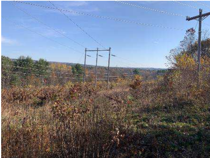
Photo 78. Early-successional, shrub-dominated ROW near H137 Structure 29. November 9, 2021.
