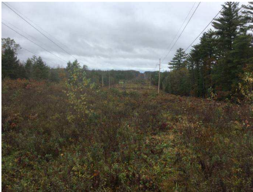
Photo 7. Existing ROW conditions near proposed C189 Structure 16 in Concord, NH. Stantec, October 26, 2021.
