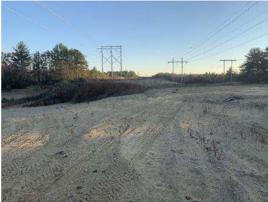
Photo 48. Sand pit with off-road vehicle use in ROW near structure 77. November 8, 2021.
