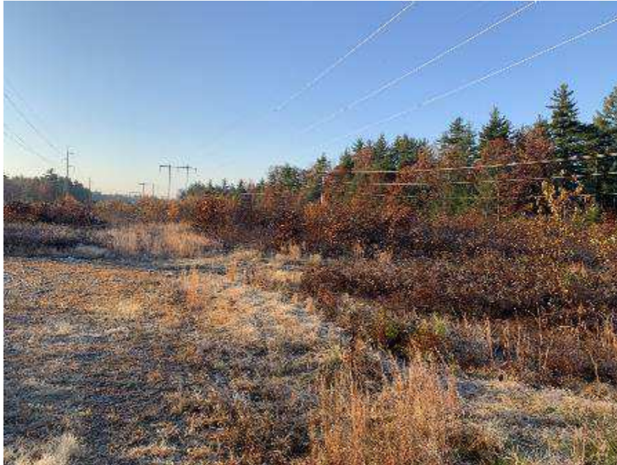
Photo 56. Scrub oak and little bluestem-dominated ROW near structure 71. November 9, 2021.
