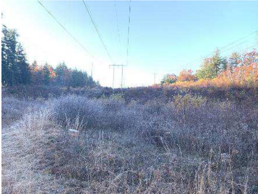
Photo 54. Scrub oak-dominated ROW near structure 74. November 9, 2021.
