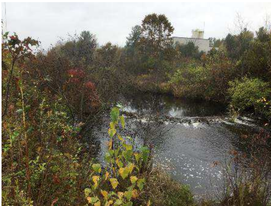
Photo 96. Bow Bog Brook near H137 Structure 8. October 27, 2021.
