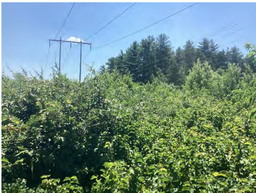
Photo 12. Louden Road to Soucook River Segment: dense shrub-dominated ROW, view to the west to structure 86. Stantec. July 19, 2022.
