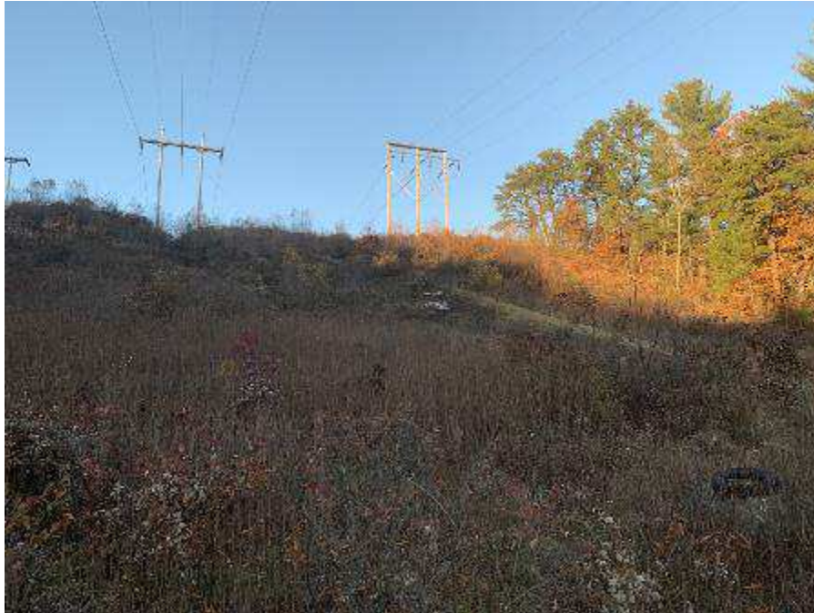
Photo 50. Sandy south-facing embankment north of Soucook River near structure 76. November 8, 2021.
