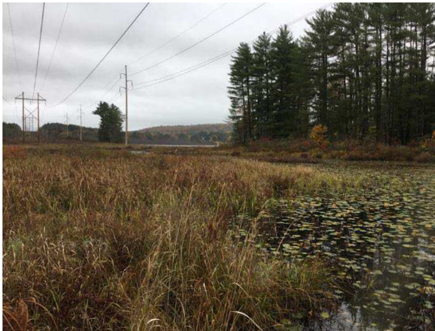
Photo 5. Existing ROW conditions near proposed C189 Structure 23 and Turtle Pond outlet in Concord, NH. Stantec, October 26, 2021.
