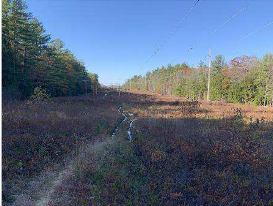
Photo 30. Wetland W18 near C189 Structure 69. November 8, 2021.
