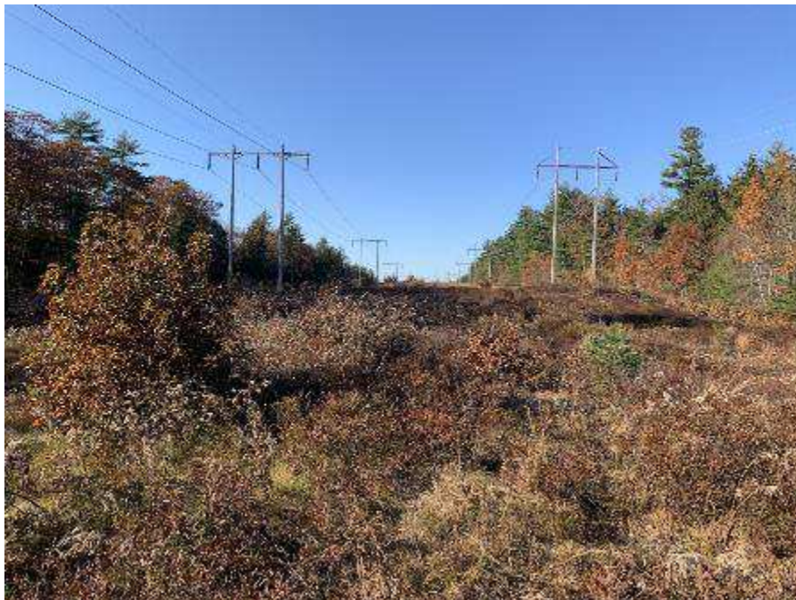
Photo 35. Shrub-dominated ROW uplands near structure 109. November 8, 2021.
