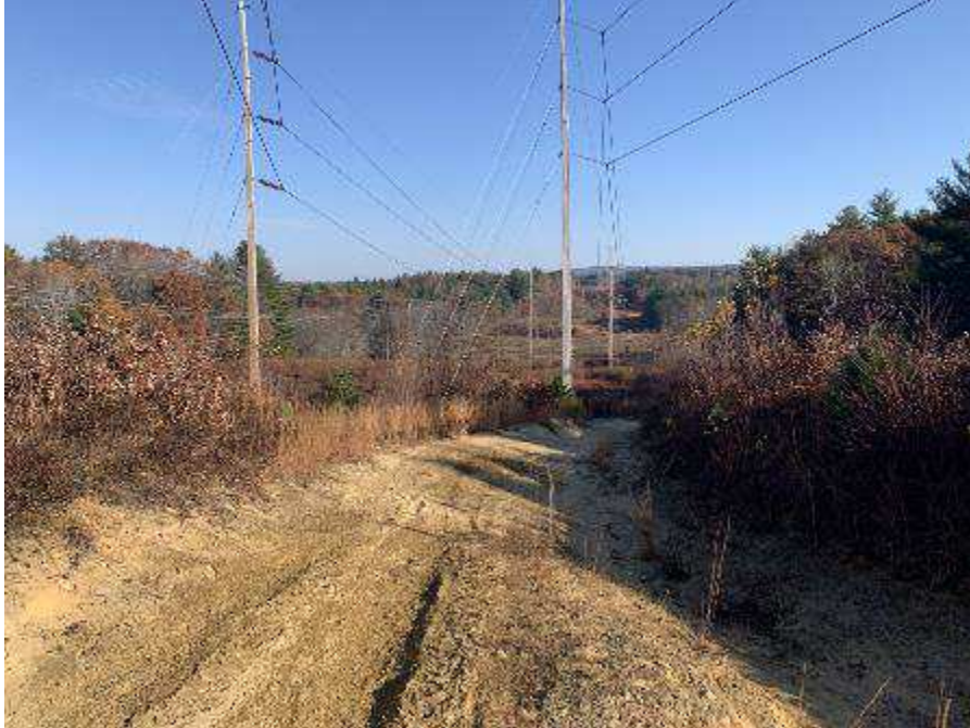
Photo 73. Shrub-dominated ROW and sandy access trail near structure 49. November 9, 2021.
