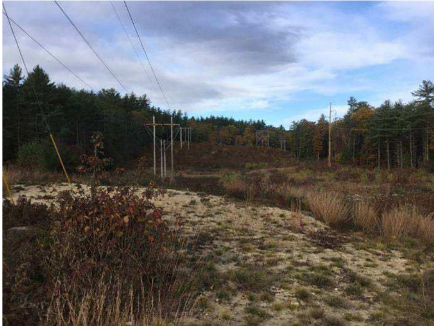
Photo 20. Existing ROW conditions near proposed H137 Structure 17 in Bow, NH. Stantec, October 28, 2021.
