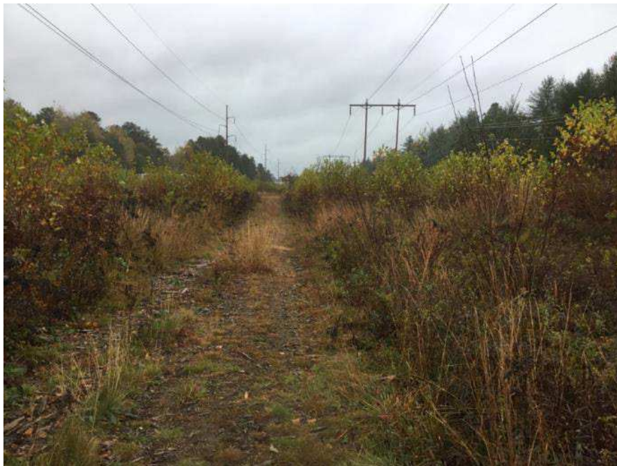
Photo 11. Existing ROW conditions and access road near proposed M108 Structure 50 in Concord, NH. Stantec, October 26, 2021.
