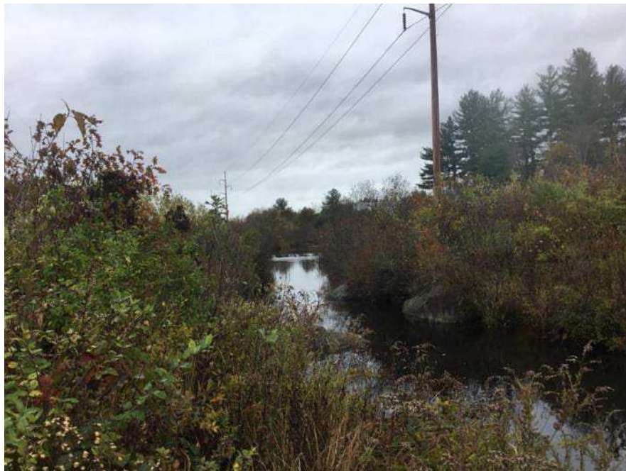
Photo 21. Existing ROW conditions and Bow Bog Brook near proposed H137 Structure 8 in Bow, NH. Stantec, October 27, 2021.
