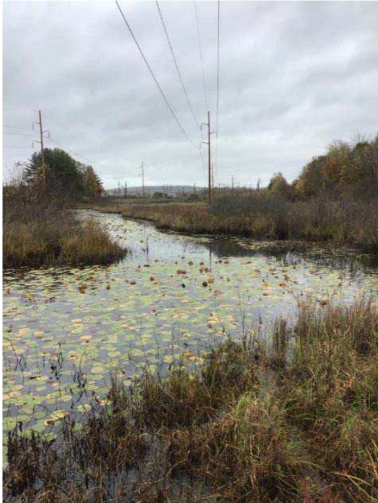
Photo 23. Existing ROW conditions and large ponded wetland near proposed H137 Structure 2 and the Merrimack substation in Bow, NH. Stantec, October 27, 2021.
