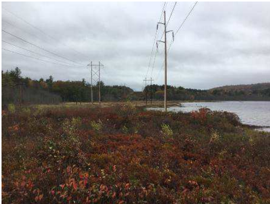
Photo 17. Wetland W15 scrub-shrub portion with Turtle Pond near C189 Structure 182. October 26, 2021.
