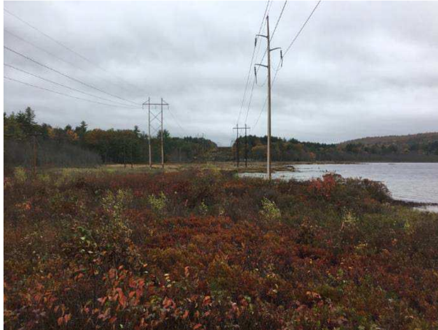
Photo 4. Existing ROW conditions near proposed C189 Structure 25 and Turtle Pond in Concord, NH. Stantec, October 26, 2021.
