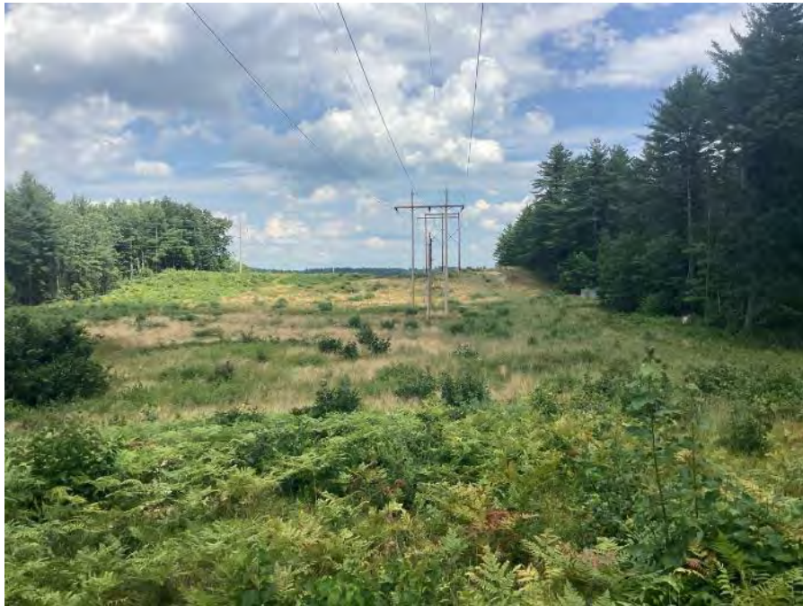
Photo 57. Structure 23 to Ferry Road Segment: sandy grassland area near structure 21, view to the east. Stantec. July 21, 2022.
