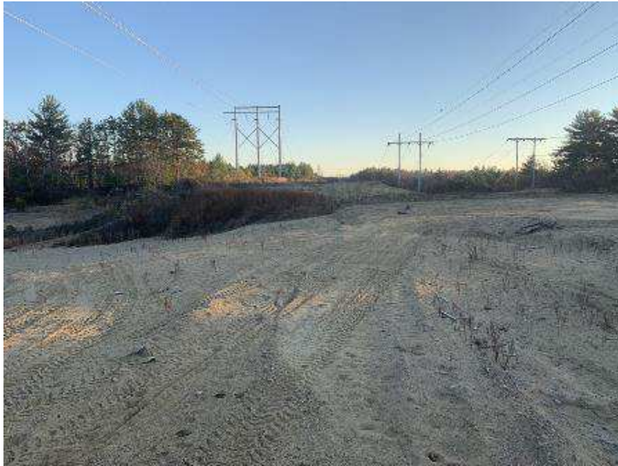
Photo 48. Sand pit with off-road vehicle use in ROW near M108 Structure 33. November 8, 2021.
