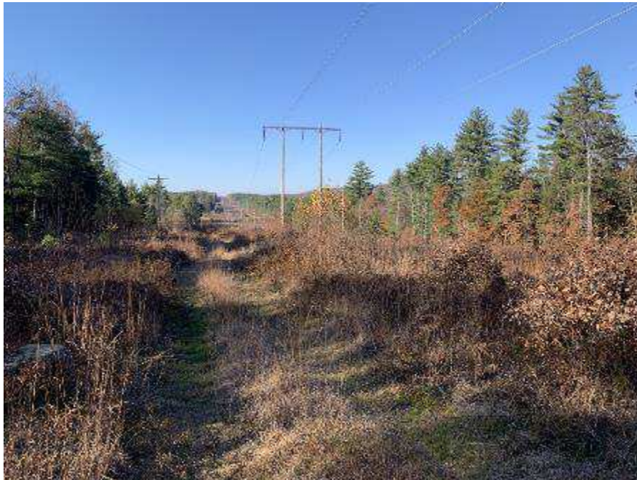
Photo 27. Scrub oak-dominated ROW near structure 121. November 8, 2021.
