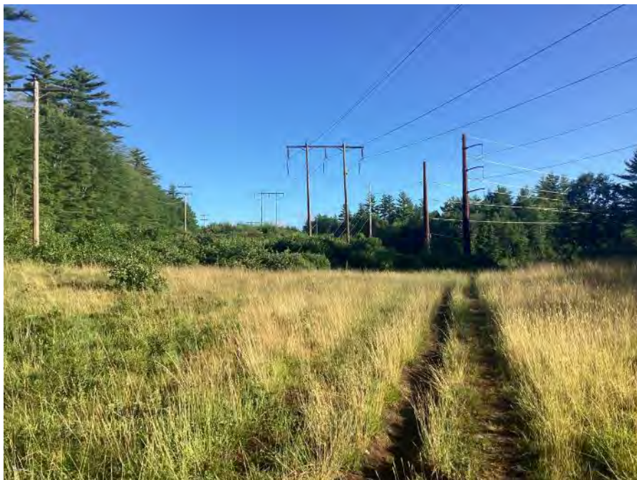
Photo 4. Structure 114 to Portsmouth Street Segment: view to the north to structure 108. Stantec. May 16, 2022.
