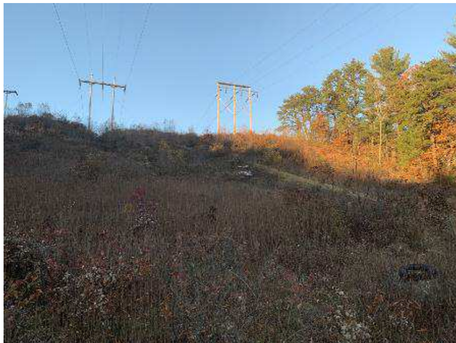
Photo 50. Sandy south-facing embankment north of Soucook River near M108 Structure 32. November 8, 2021.
