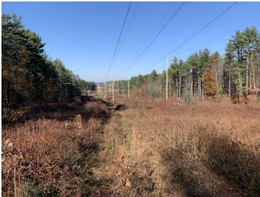
Photo 6. Representative shrub-dominated ROW uplands near C189 Structure 105. November 8, 2021.
