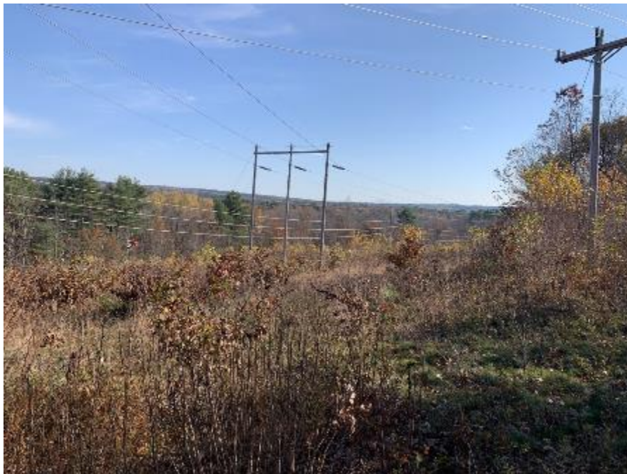
Photo 78. Early-successional, shrub-dominated ROW near H137 Structure 29. November 9, 2021.
