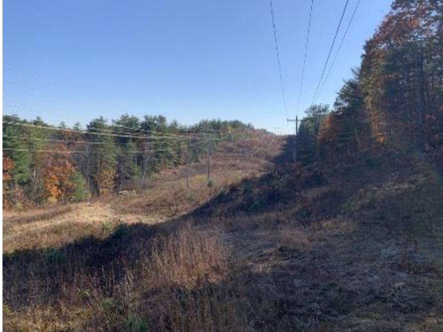
Photo 7. Representative ROW uplands near C189 Structure 99. November 8, 2021.
