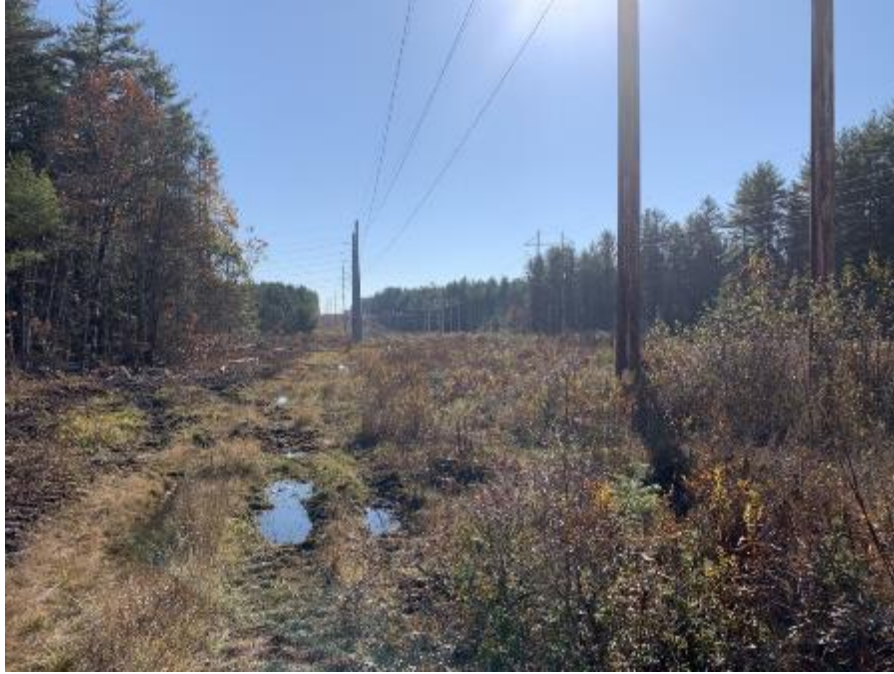
Photo 3. Row near C189 Structure 109, view to the south. November 8, 2021.
