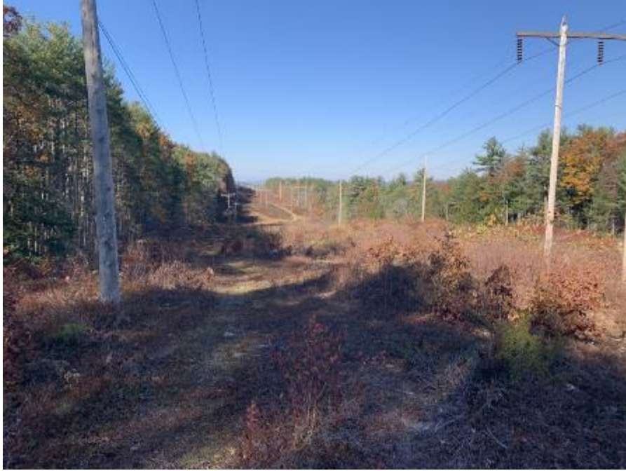
Photo 9. Representative ROW uplands near C189 Structure 96. November 8, 2021.
