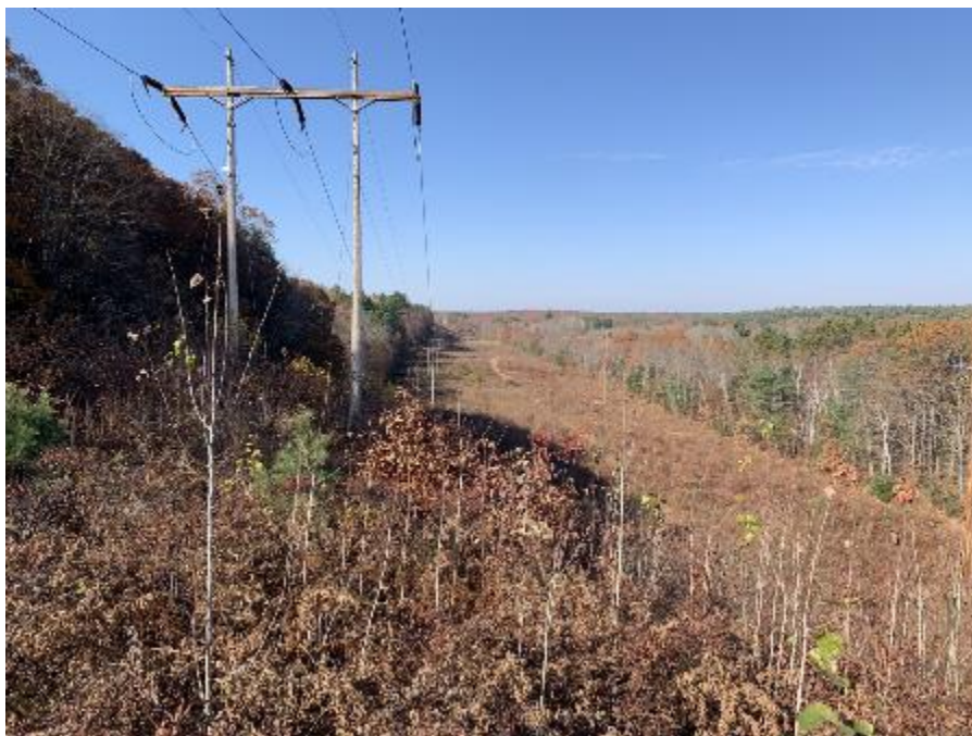
Photo 85. Representative ROW from H137 Structure 20. November 9, 2021.
