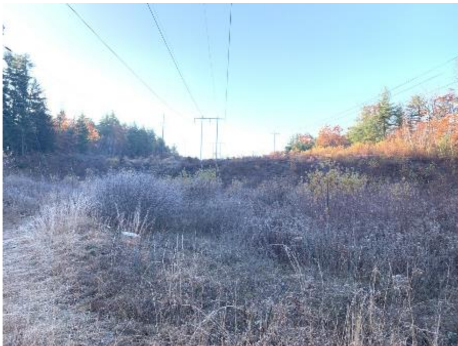
Photo 54. Scrub oak-dominated ROW near M108 Structure 31. November 9, 2021.
