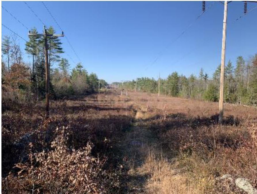
Photo 25. Shrub-dominated ROW near C189 Structure 74. November 8, 2021.
