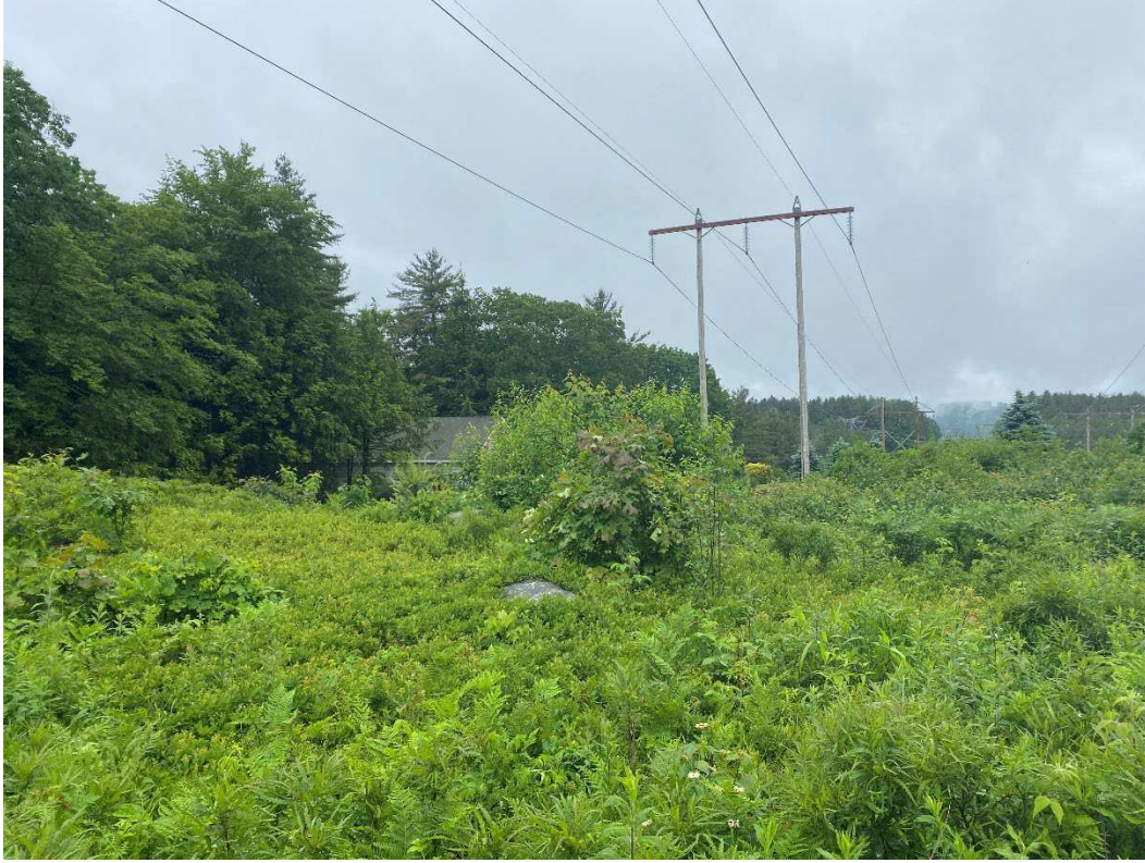
Photograph No. 19: Looking at proposed work pad location for Q171 Structure 122.
