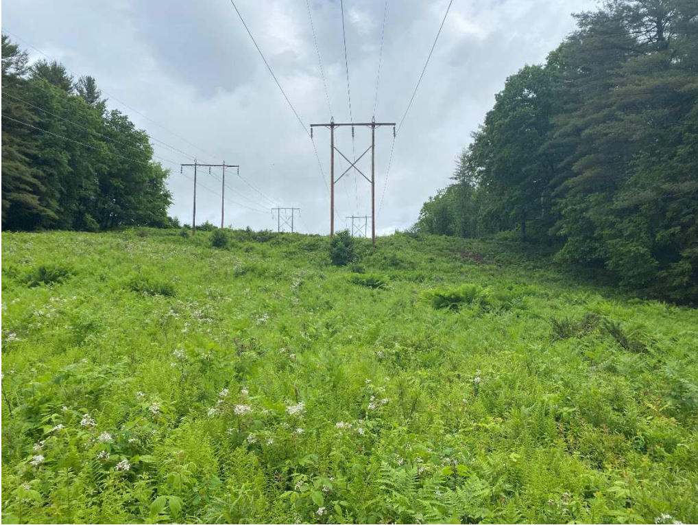
Photograph No. 29: Looking at proposed access and work pad location for Q171 Structure 109.
