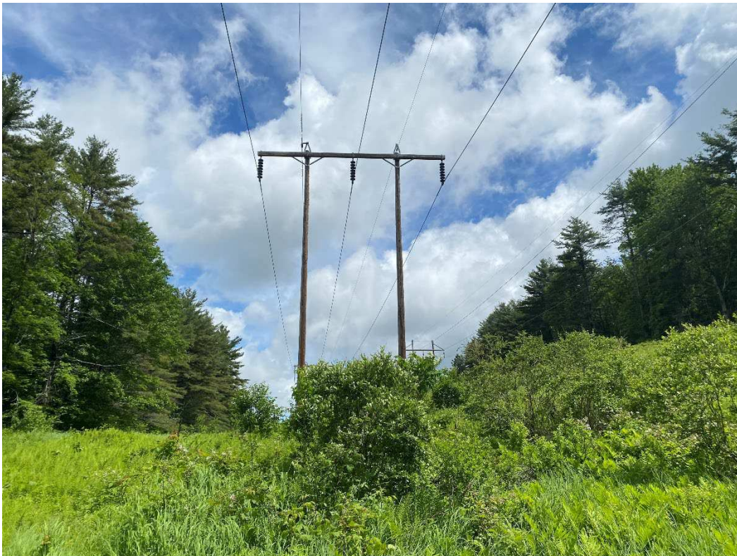
Photograph No. 38: Looking at proposed access for C196 Structure 92.
