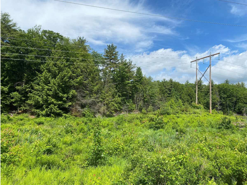
Photograph No. 43: Looking at proposed access and work pad location adjacent to C196 Structure 89.
