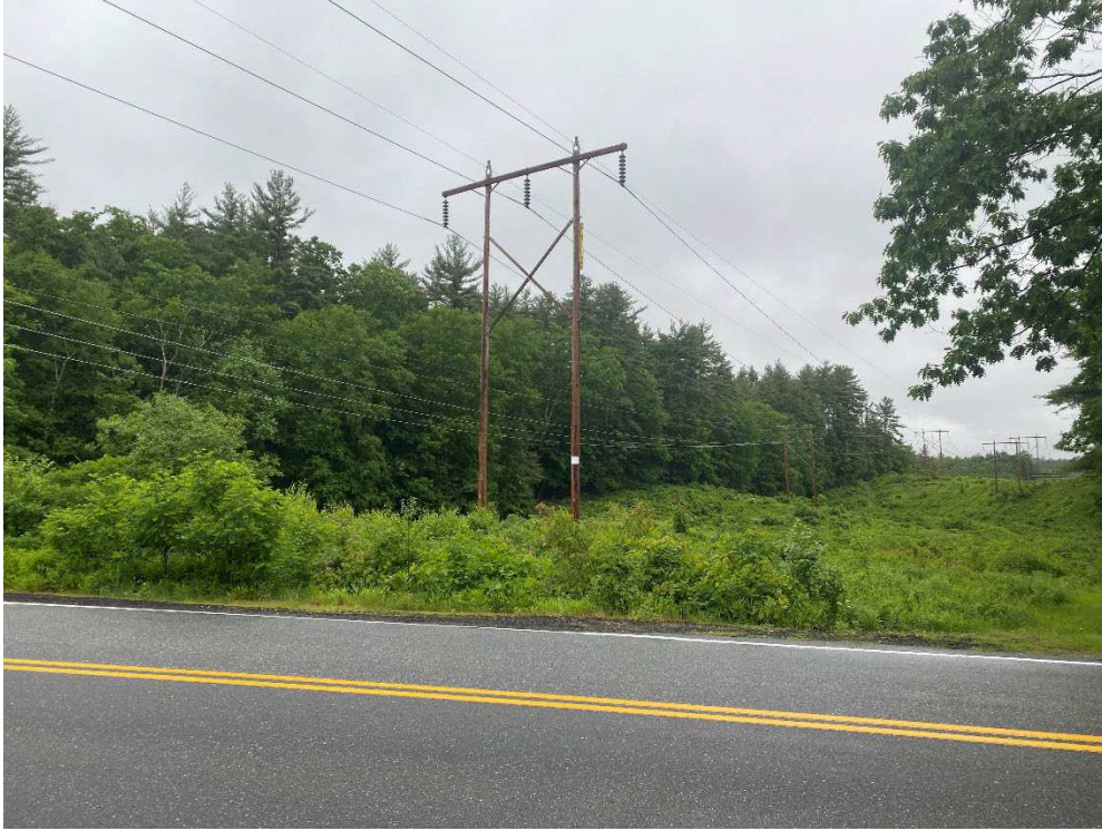
Photograph No. 9: Looking at proposed access and work pad location from Locus Hill Road to Q171 Structure 130.
