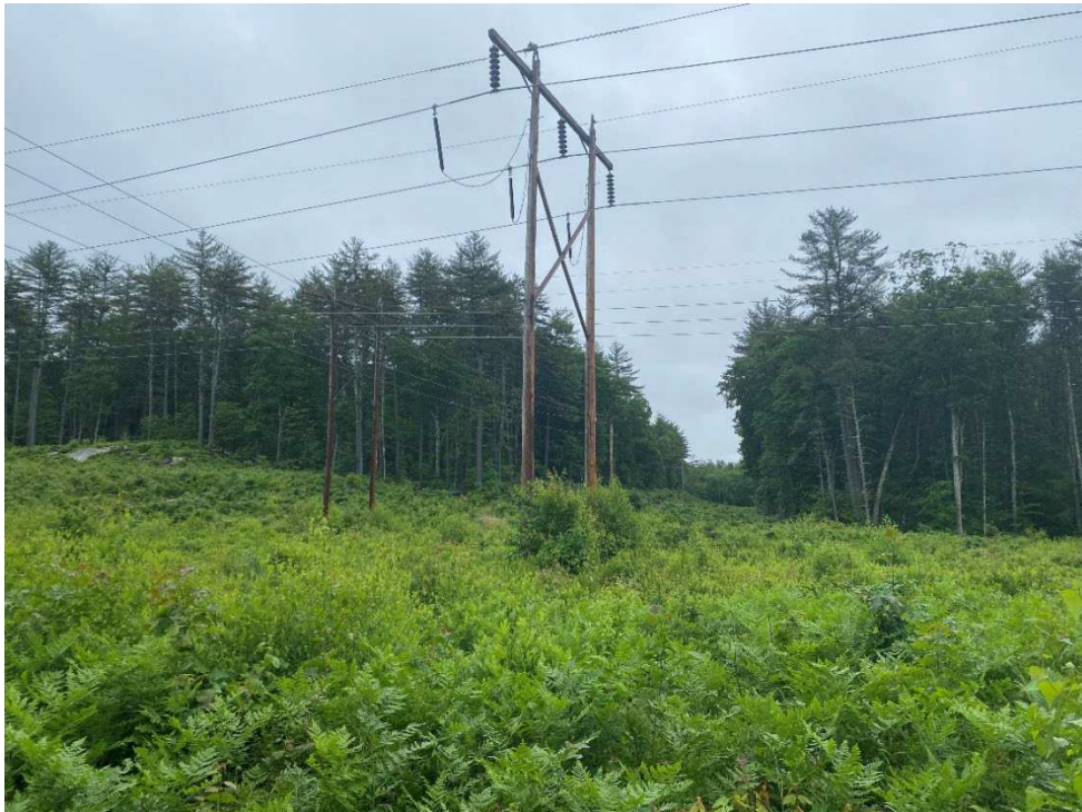
Photograph No. 4: Looking at proposed access and work area for C196 Structure 141.
