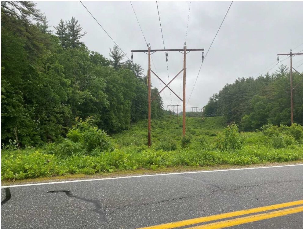
Photograph No. 10: Looking at proposed access and work pad location from Locus Hill Road for C196 Structure 135.
