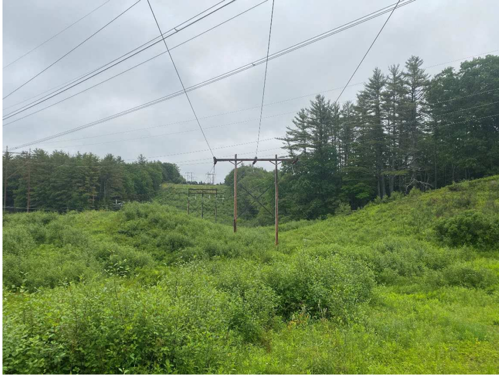
Photograph No. 15: Looking at proposed access and work pad location for Q171 Structure 126.
