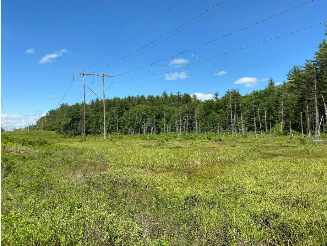
Photograph No. 57: Looking at proposed access and work pad location for Q171 Structure 68
