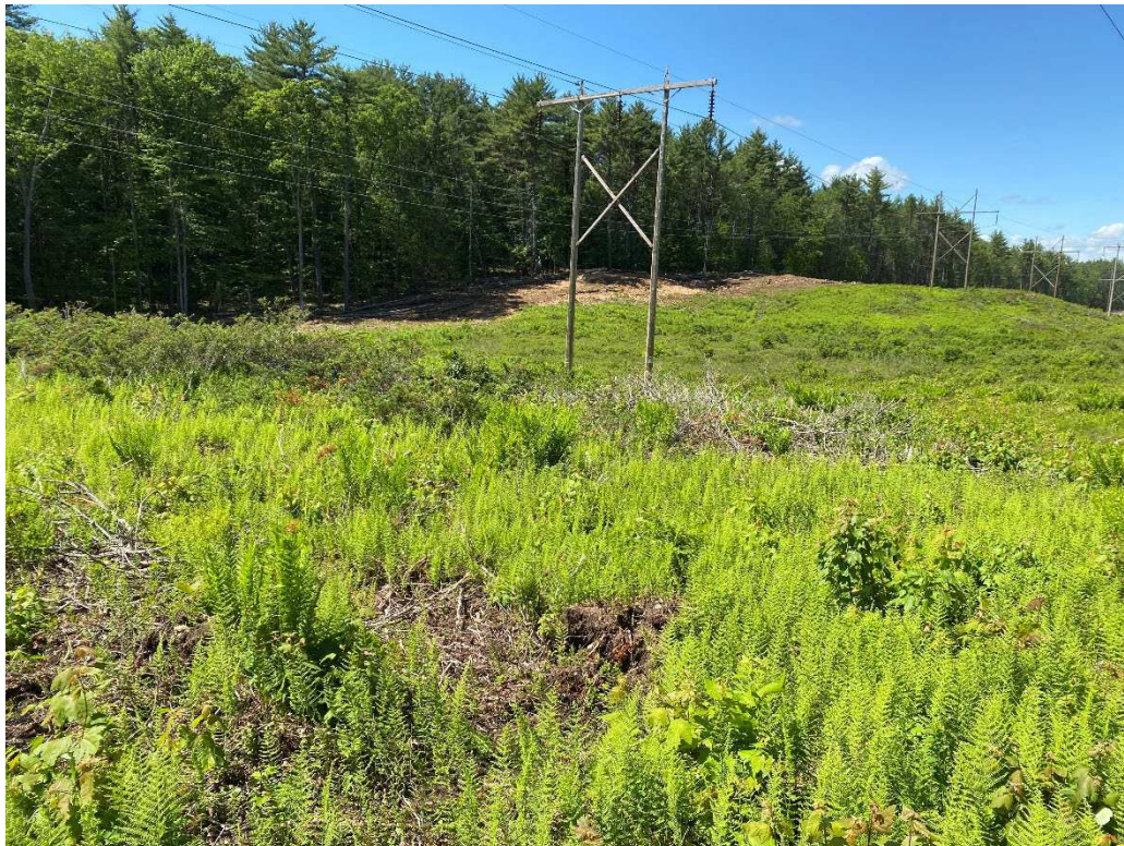
Photograph No. 54: Looking at proposed access and work pad location for C196 Structure 71.
