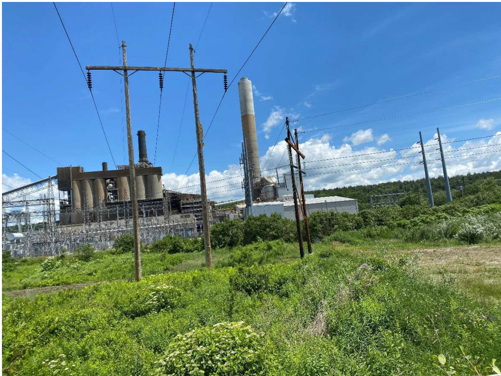
Photograph No. 88: Looking at proposed access and work pad location for Q171 Structure 1.
