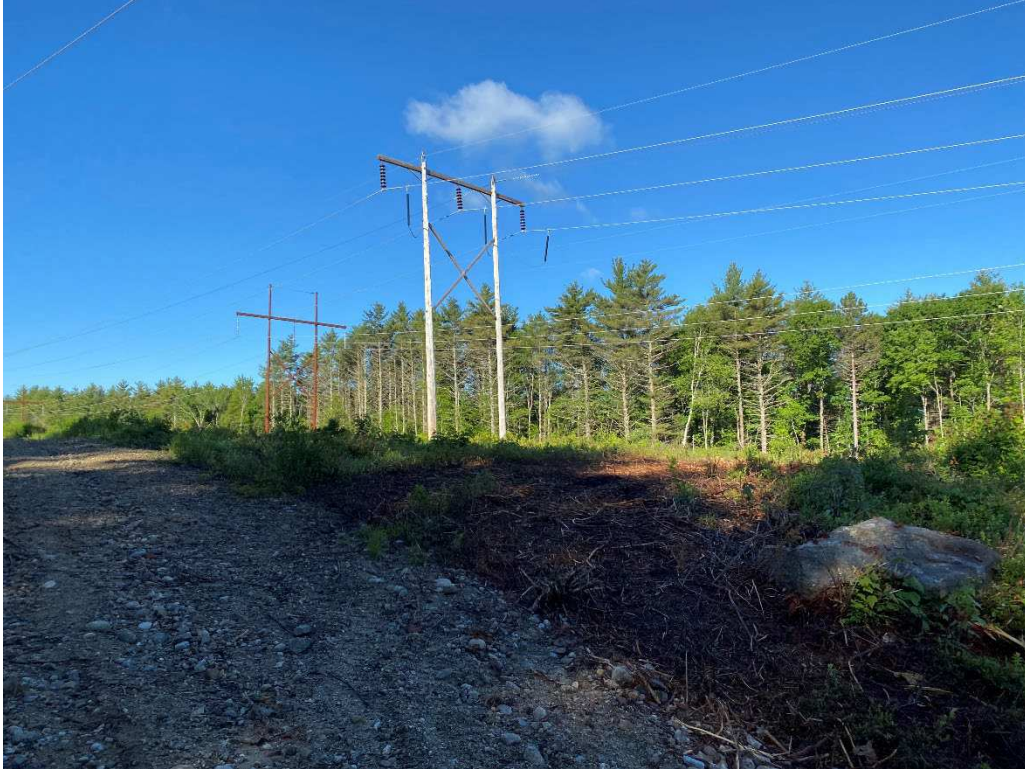
Photograph No. 63: Looking at proposed access and work pad location for C196 Structure 65.
