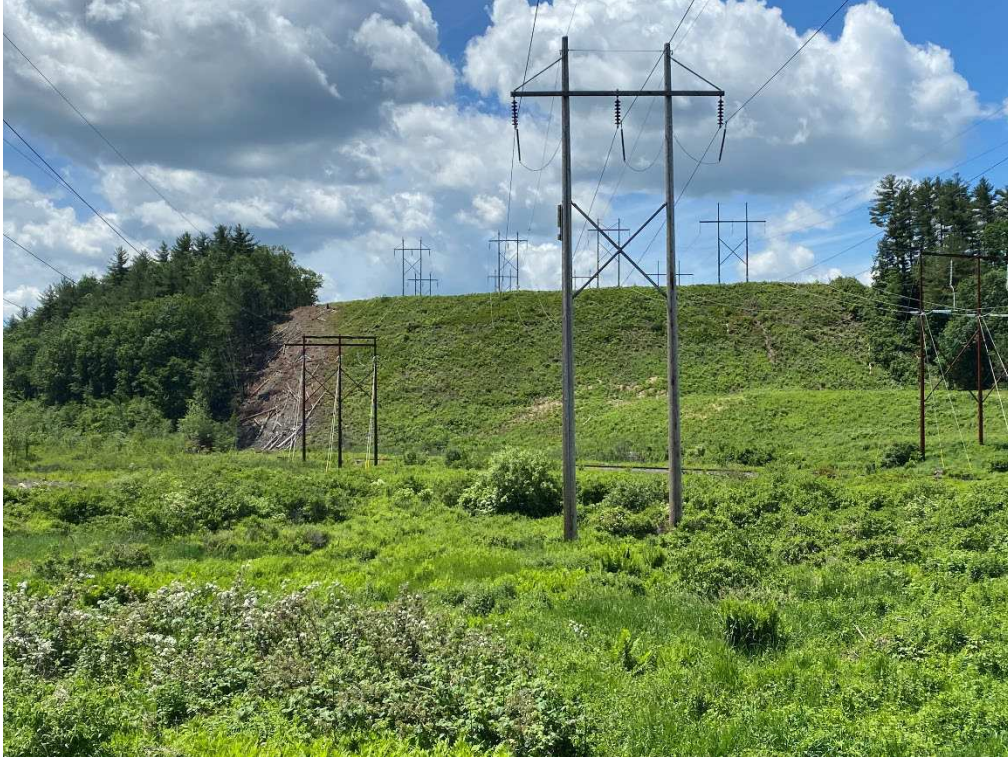
Photograph No. 83: Looking at proposed access and work pad location for Q171 Structure 4.
