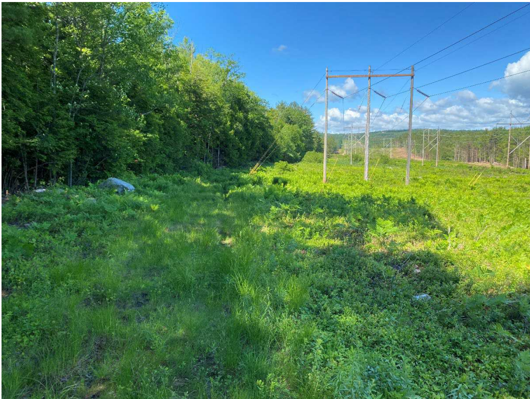
Photograph No. 78: Looking at proposed access and work pad location for Q171 Structure 32.
