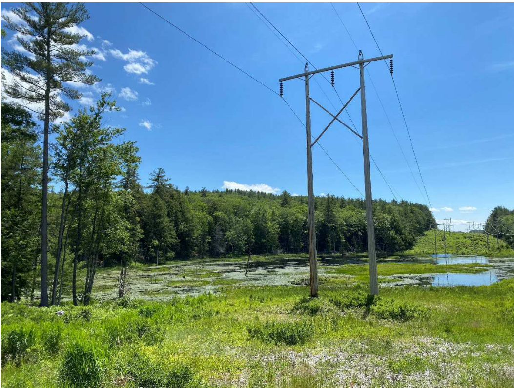
Photograph No. 46: Looking at proposed access and work pad location for Q171 Structure 86.
