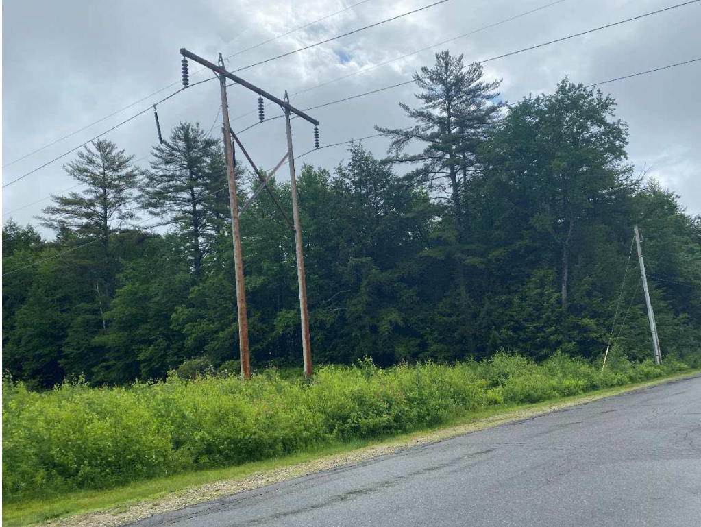
Photograph No. 23: Looking at proposed access and work pad location from Kimberly Lane for Q171 Structure 119.
