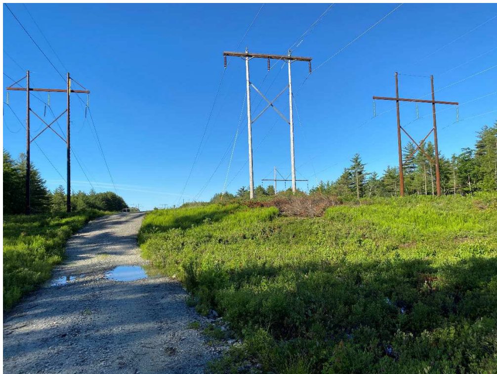
Photograph No. 66: Looking at proposed access and work pad location for C196 Structure 63.
