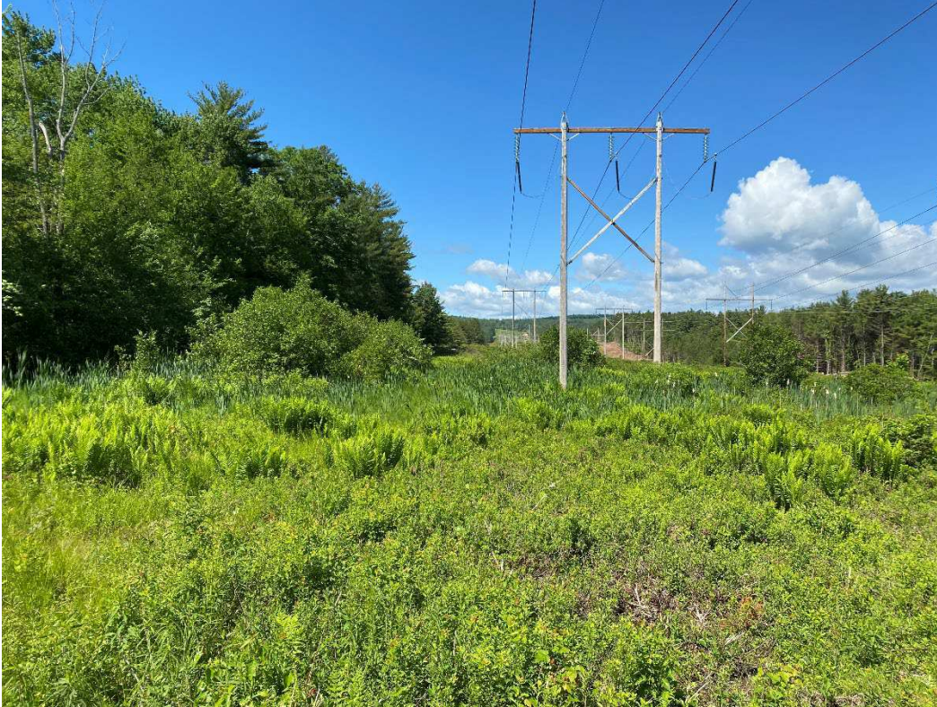
Photograph No. 77: Looking at proposed access and work pad location for Q171 Structure 33.
