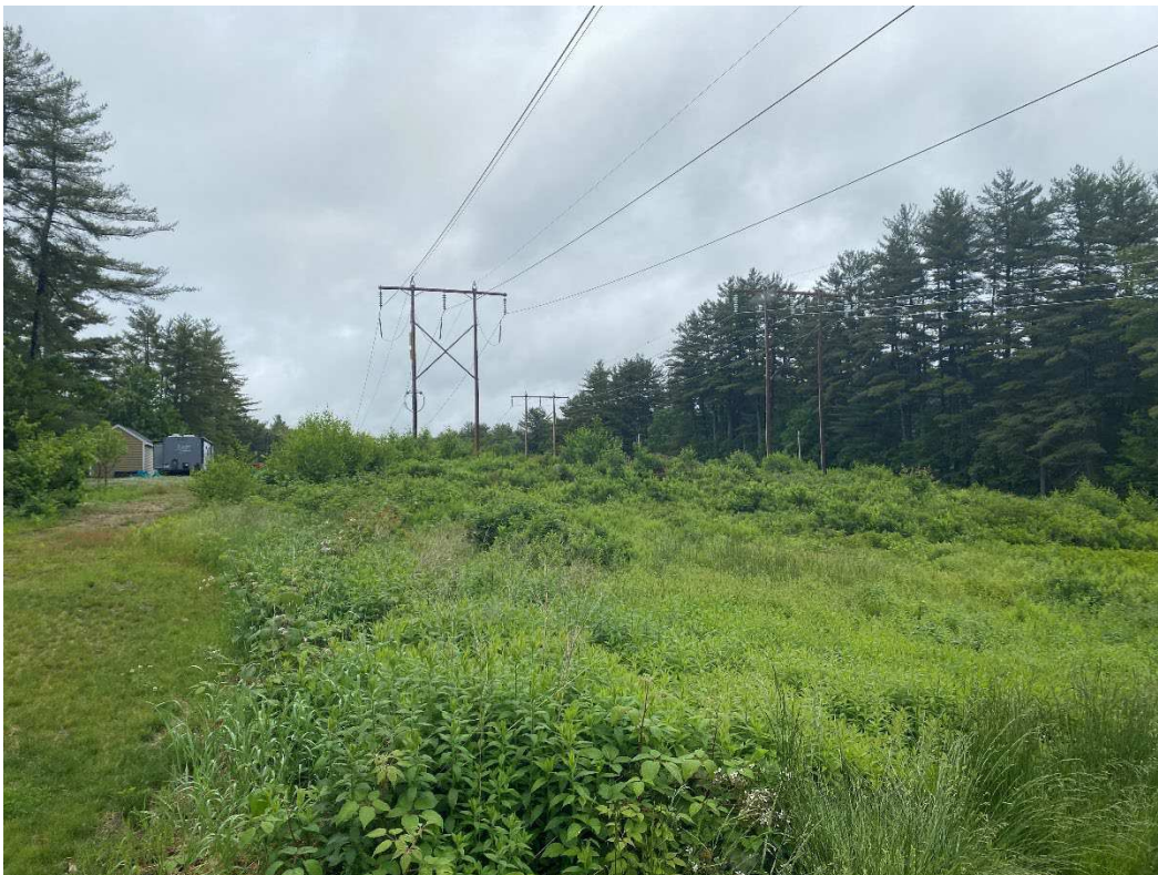
Photograph No. 26: Looking at proposed access and work pad location for Q171 Structure 112.
