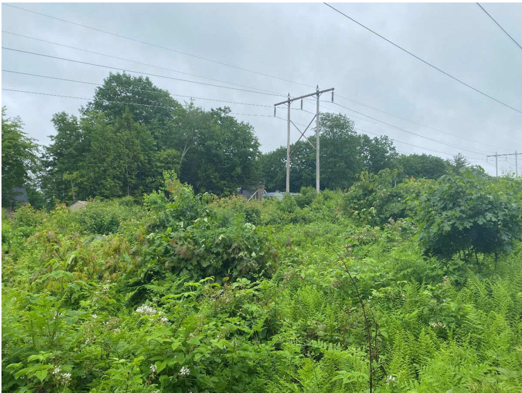
Photograph No. 22: Looking at proposed access and work pad location for Q171 Structure 120.
