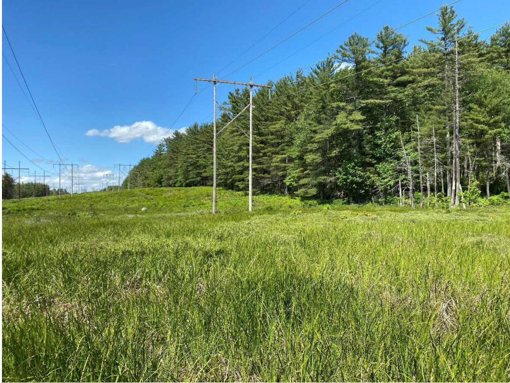
Photograph No. 59: Looking at proposed access and work pad location for Q171 Structure 67.
