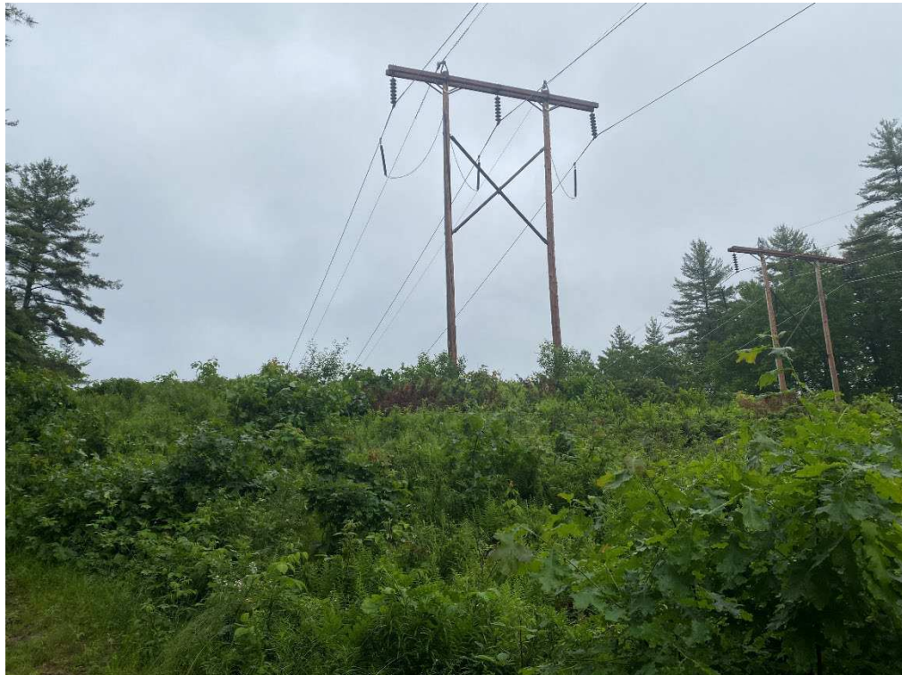
Photograph No. 12: Looking at proposed access and work pad location for C196 Structure 133.
