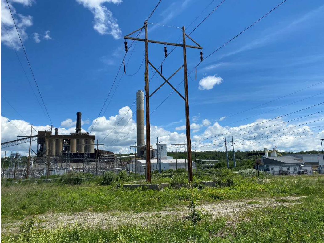
Photograph No. 87: Looking at proposed access and work pad location for C196 Structure 1A.
