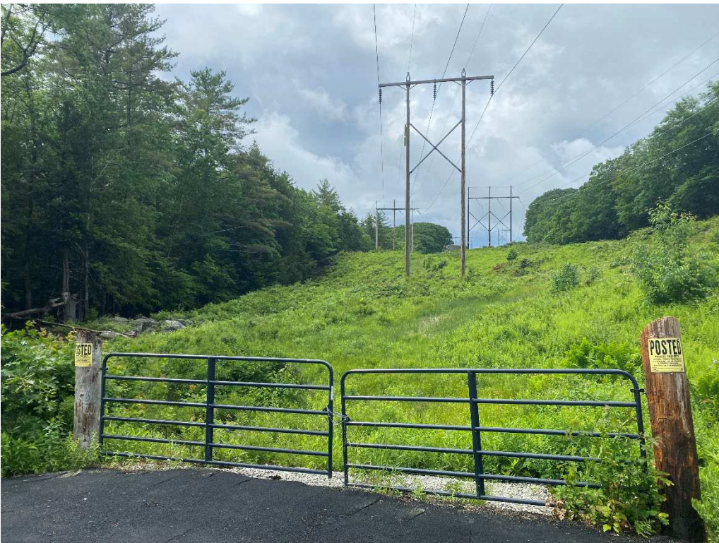
Photograph No. 30: Looking at proposed access and work pad location from Black Brook Road for Q171 Structure 104.
