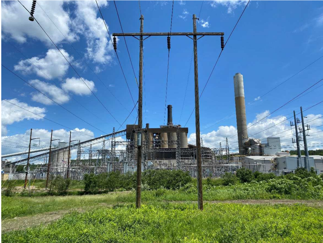
Photograph No. 89: Looking at proposed access and work pad location for C196 Structure 1.
