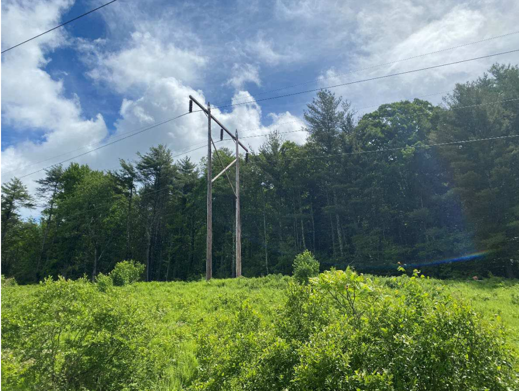
Photograph No. 37: Looking at proposed access and work pad location for Q171 Structure 90.
