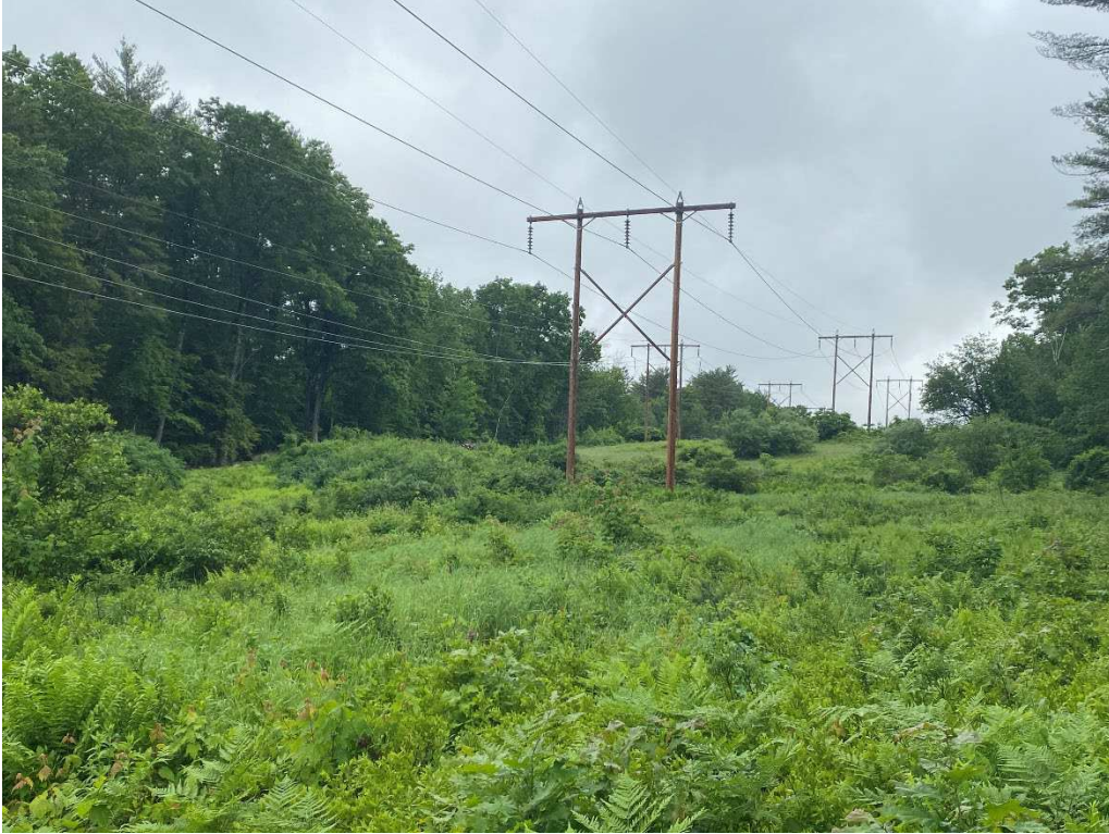
Photograph No. 25: Looking at proposed access and work pad location for Q171 Structure 117.
