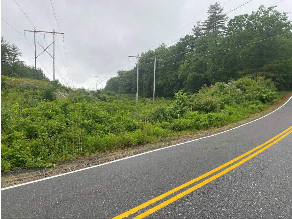
Photograph No. 7: Looking at proposed access and work pad location from Locus Hill Road for C196 Structure 136 (right).
