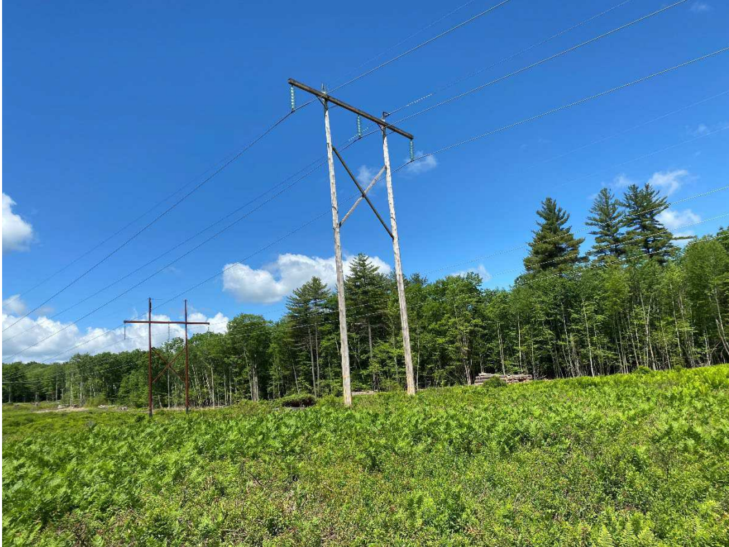
Photograph No. 81: Looking at proposed access and work pad location for C196 Structure 20.
