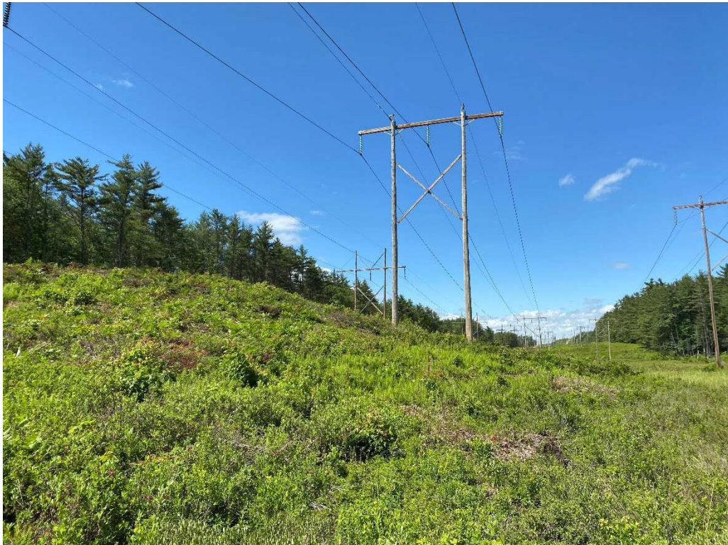
Photograph No. 56: Looking at proposed access and work pad location for C196 Structure 69.
