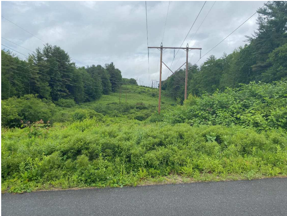
Photograph No. 28: Looking at proposed access and work pad location for Q171 Structure 110.
