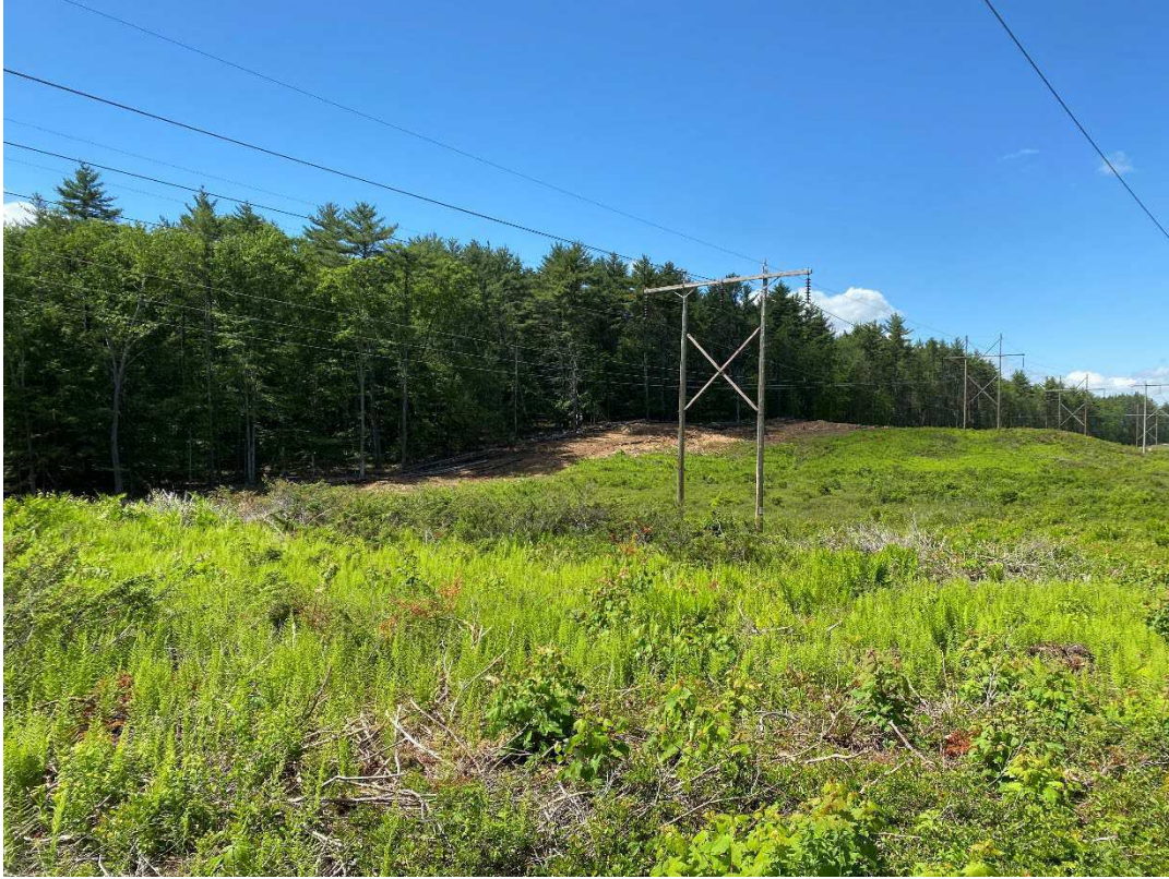
Photograph No. 55: Looking at proposed access and work pad location for C196 Structure 70.
