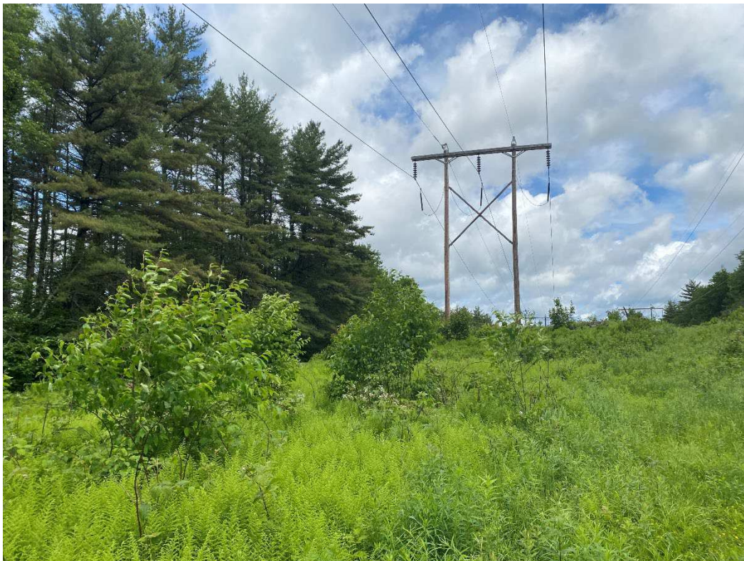
Photograph No. 40: Looking at proposed access and work pad location for C196 Structure 91.
