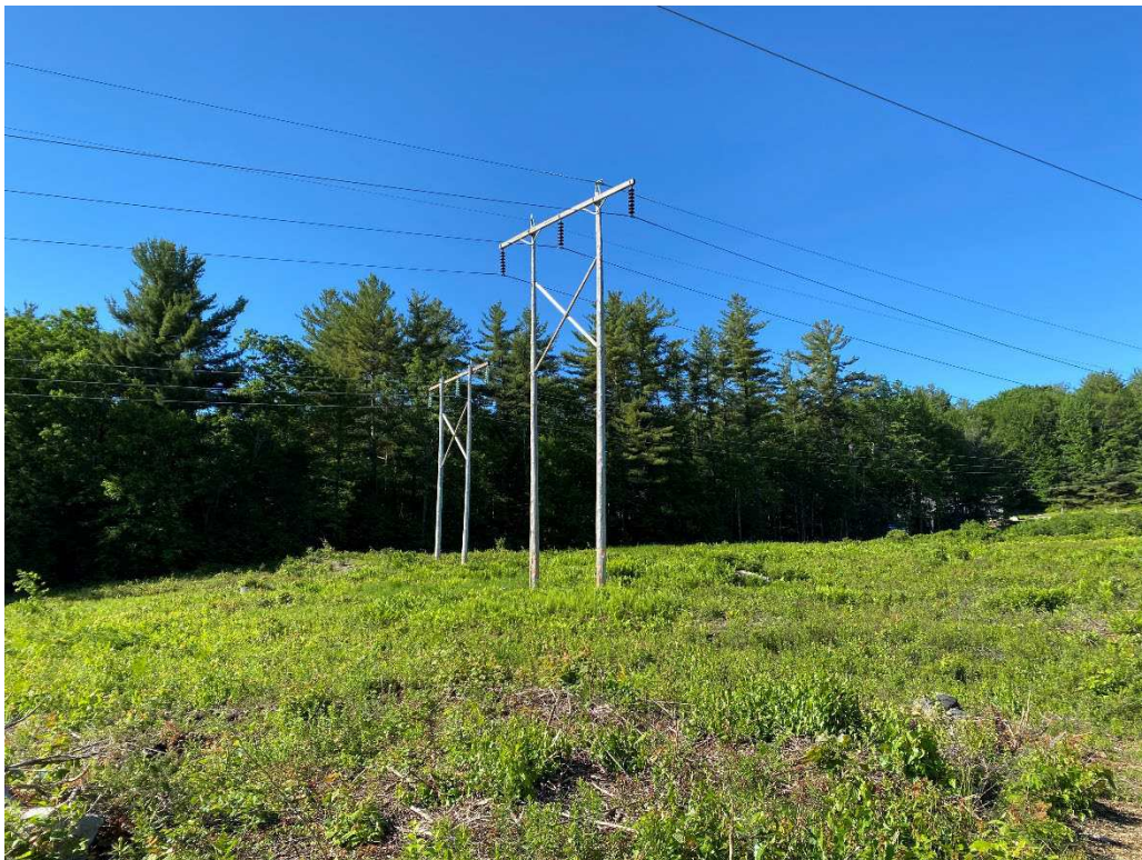
Photograph No. 70: Looking at proposed access and work pad location for C196 Structure 46.
