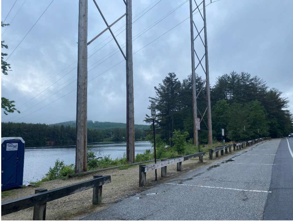
Photograph No. 1: Looking at proposed access and work pad location from Elm Street for Q171 Structure 139 (left).
