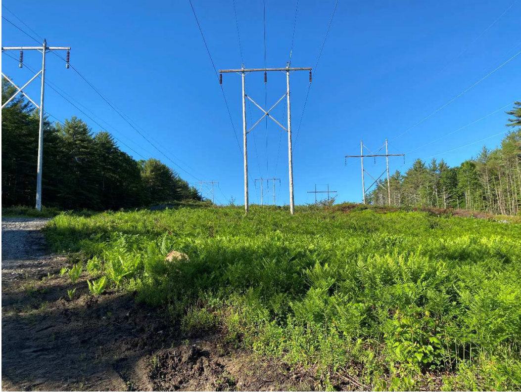
Photograph No. 65: Looking at proposed access and work pad location for C196 Structure 64 (center).
