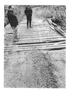
Figure 1 and 2- Shows the broken boards on the bridges that need to be replaced.
