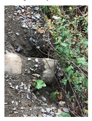
Figure 6- Depicting the area where the water is eroding around the culvert.
