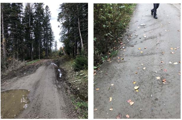
Figure 4- Mud on trail and ATV tracks in ditch and minor sedimentation on trail from water.
