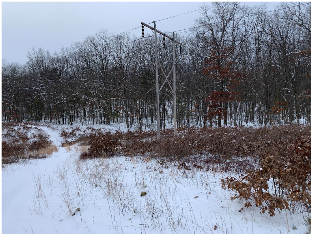
Photograph No. 12: Looking at proposed access and work pad location for Structure 110.
