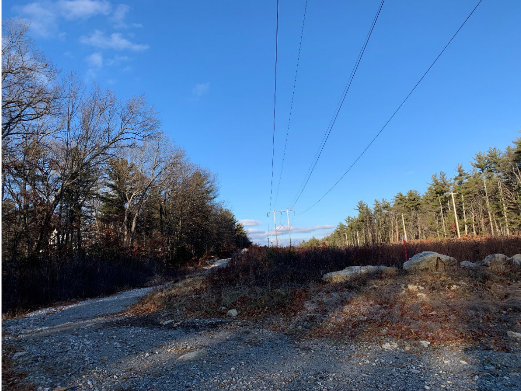
Photograph No. 7: Looking at proposed access and work pad location for Structure 94.
