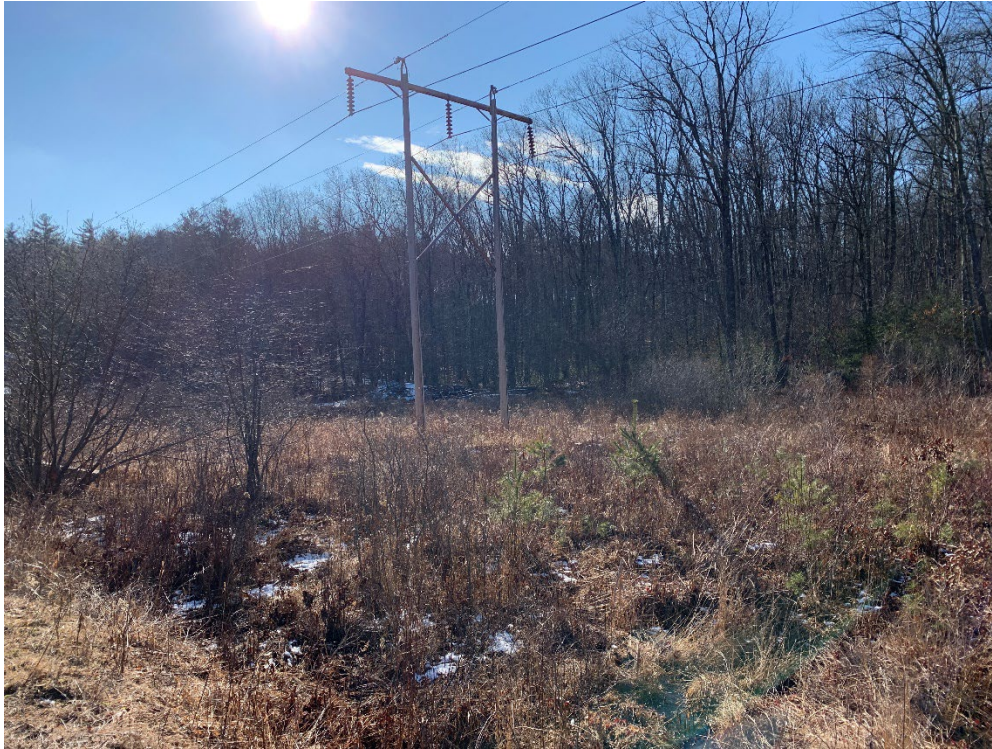
Photograph No. 1: Looking at proposed access and work area for Structure 70.
