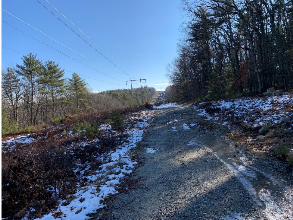
Photograph No. 3: Looking at proposed access and work pad location for Structure 73.
