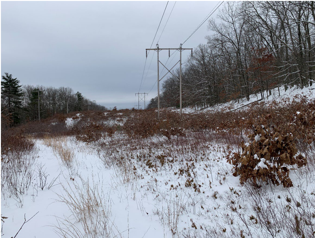
Photograph No. 14: Looking at proposed access and work pad location for Structure 112.
