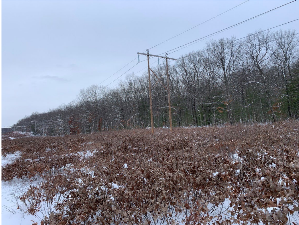
Photograph No. 11: Looking at proposed work pad location for Structure 109.
