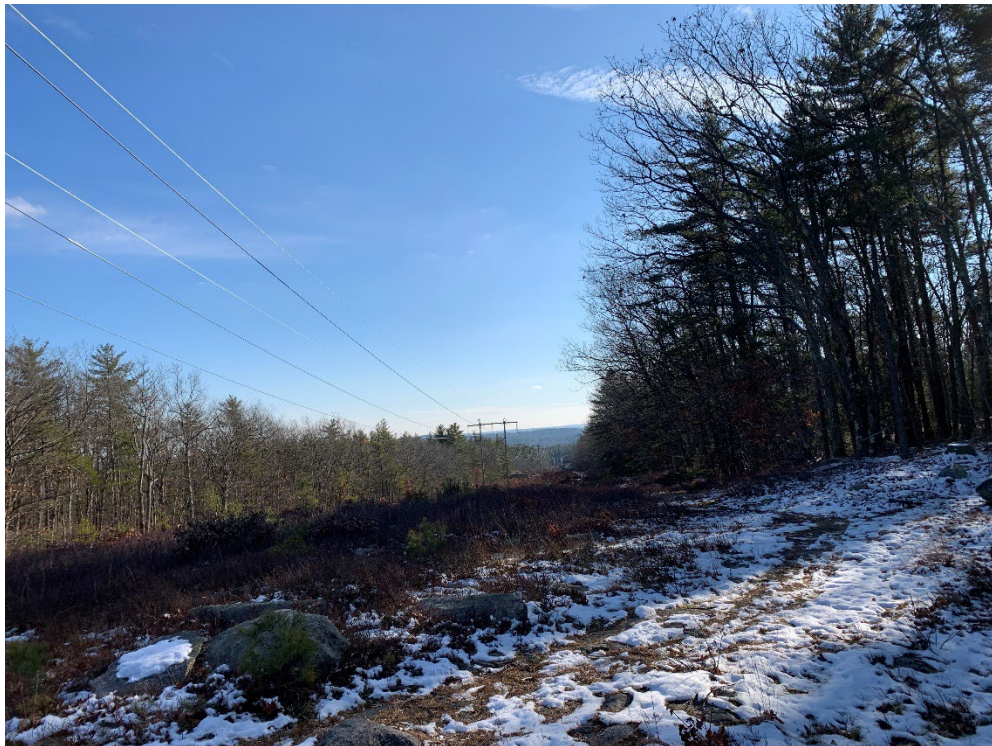
Photograph No. 6: Looking at proposed access and work pad location for Structure 80.
