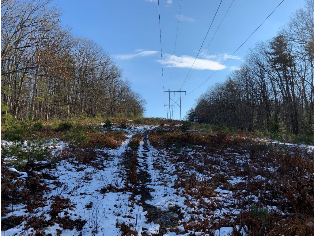
Photograph No. 5: Looking at proposed access and work pad for Structure 79.
