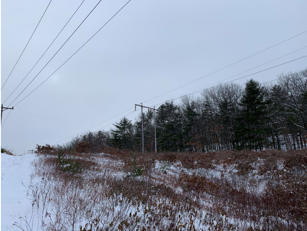
Photograph No. 9: Looking at proposed access and work pad location for Structure 107.
