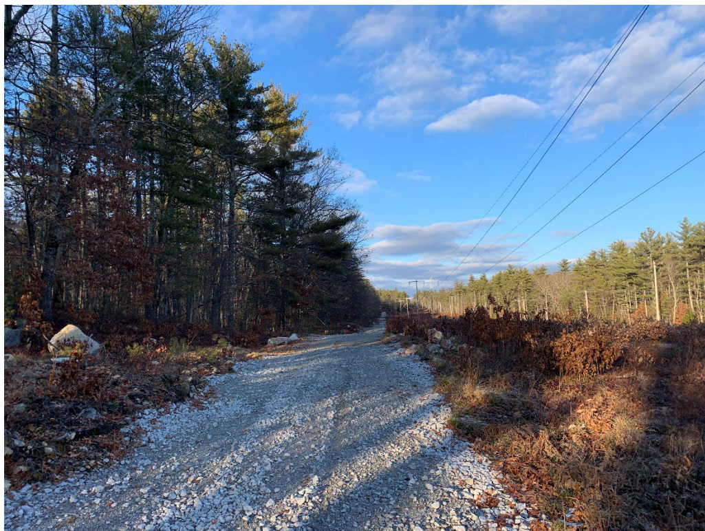
Photograph No. 8: Looking at proposed access and work pad location for Structure 93.
