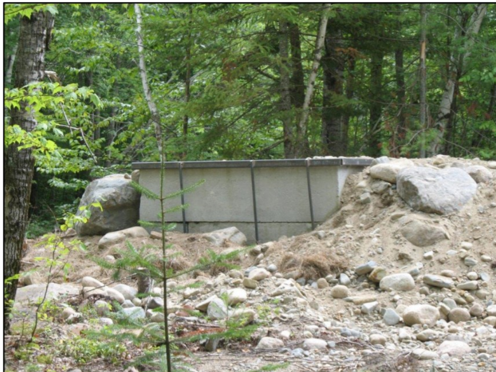
Picture of completed west abutment.
