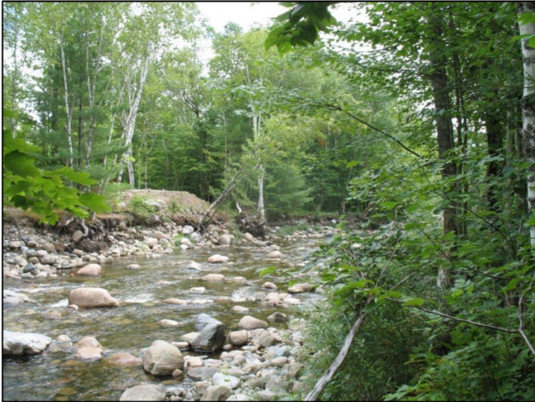
View of river crossing with east abutment shown on the left.
