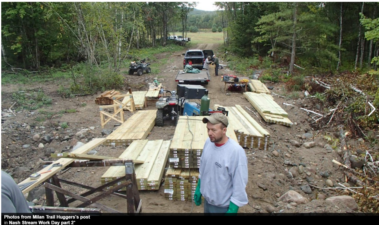
West side of river looking west: September 14, 2019
