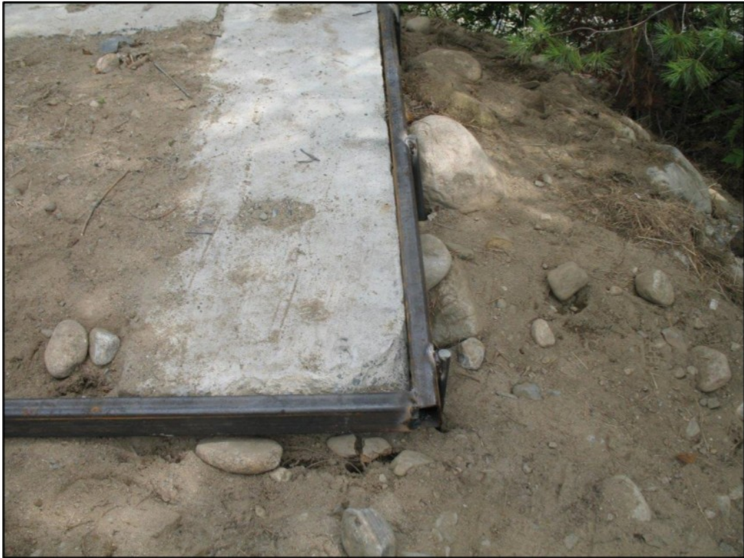
Bridge abutment, August 24, 2019
