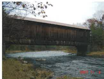
Wright's Covered Railroad Bridge (1906), Newport, N. H. (Photograph by James L. Garvin)
