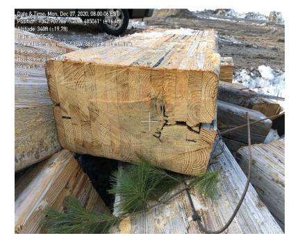
Rot and Splitting at Joints – K105 Line, Structure #32
