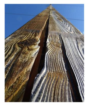
Side Crack – L175 Line, Structure #122
