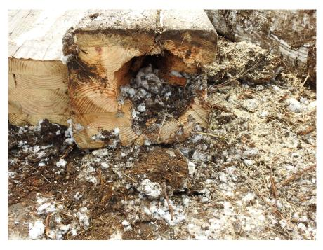
Large Crack – X116 Line, Structure #133 Extensive Rot – Z119 Line, Structure #137
