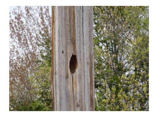
Crack Through Woodpecker Hole – L175 Line, Structure #139
