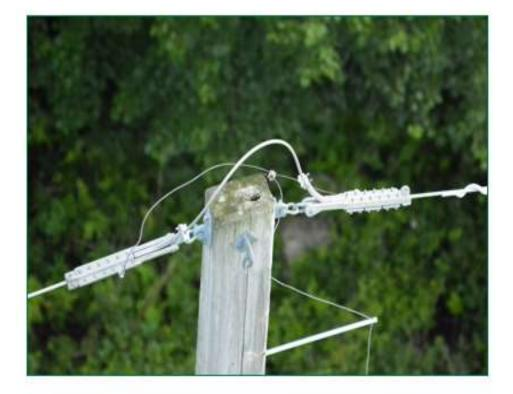
Rotten Pole Top – K105 Line, Structure #20 Woodpecker Damage – K105 Line, Structure #54
