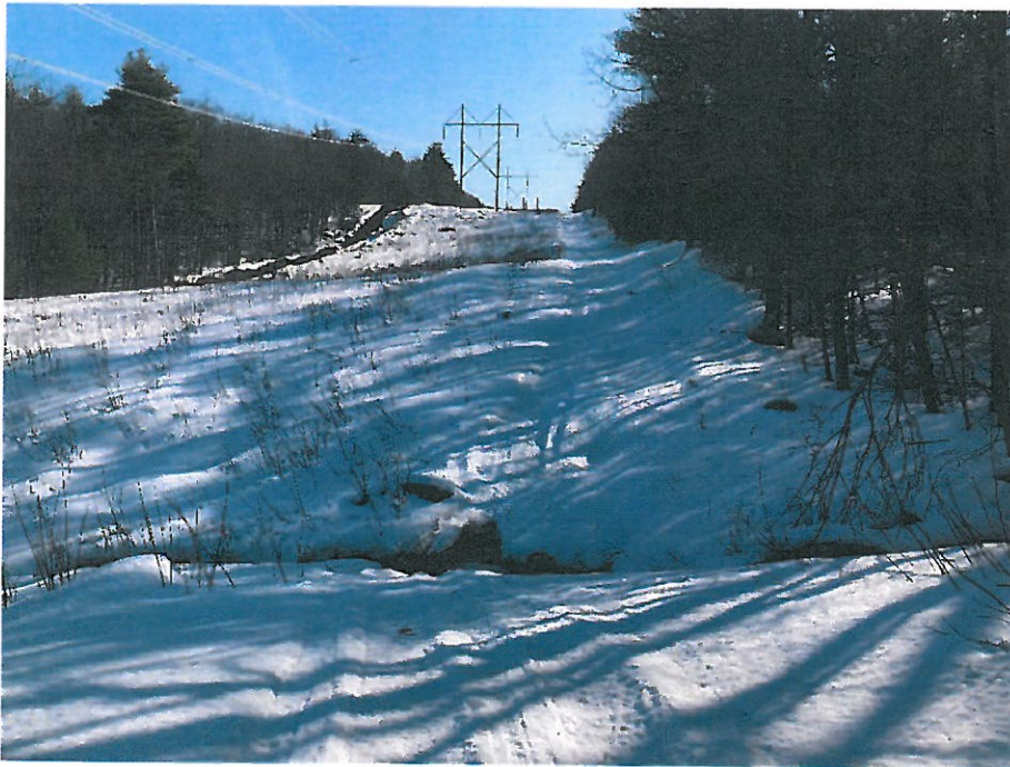
Photograph No. 5: Looking easterly at proposed access route through Wetland IW-24 towards Structure 296. Timber matting will be used through the wetland portion of the access road.
