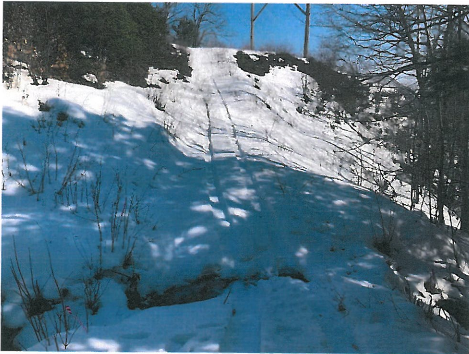
Photograph No. 13: Looking easterly at proposed access route through Wetland IW-19 toward Structure 288 to be replaced. Timber matting will be used through the wetland portion of the access road.
