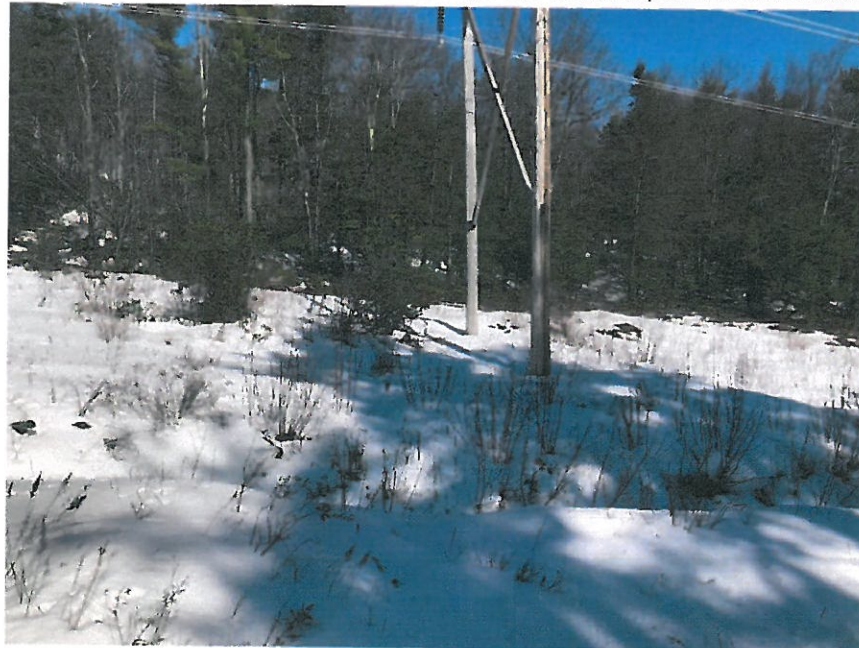
Photograph No. 16: Looking northerly at proposed access route through Wetland IW-16 toward Structure 287 to be replaced. Timber matting will be used through the wetland portion of the access road.
