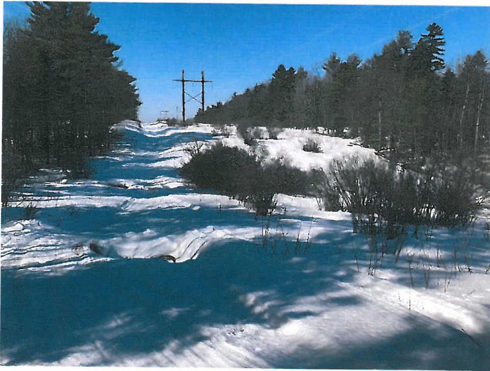
Photograph No. 7: Looking westerly at proposed access route through Wetland IW-22 (left) towards Structure 294. Timber matting will be used through the wetland portion of the access road.
