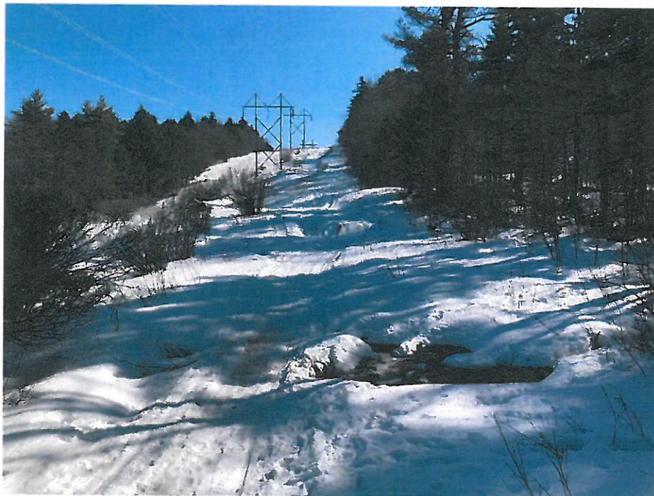
Photograph No. 6: Looking easterly at proposed access route through Wetland IW-22 towards Structure 293. Timber matting will be used through the wetland portion of the access road.
