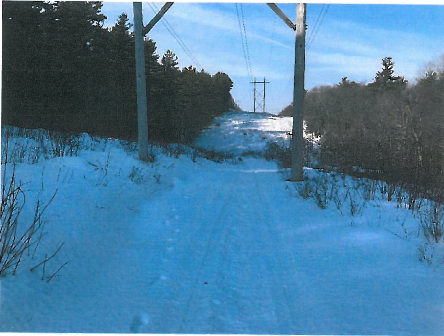
Photograph No. 3: Looking southeasterly at proposed access and work pad at Structure 304 to be replaced.
