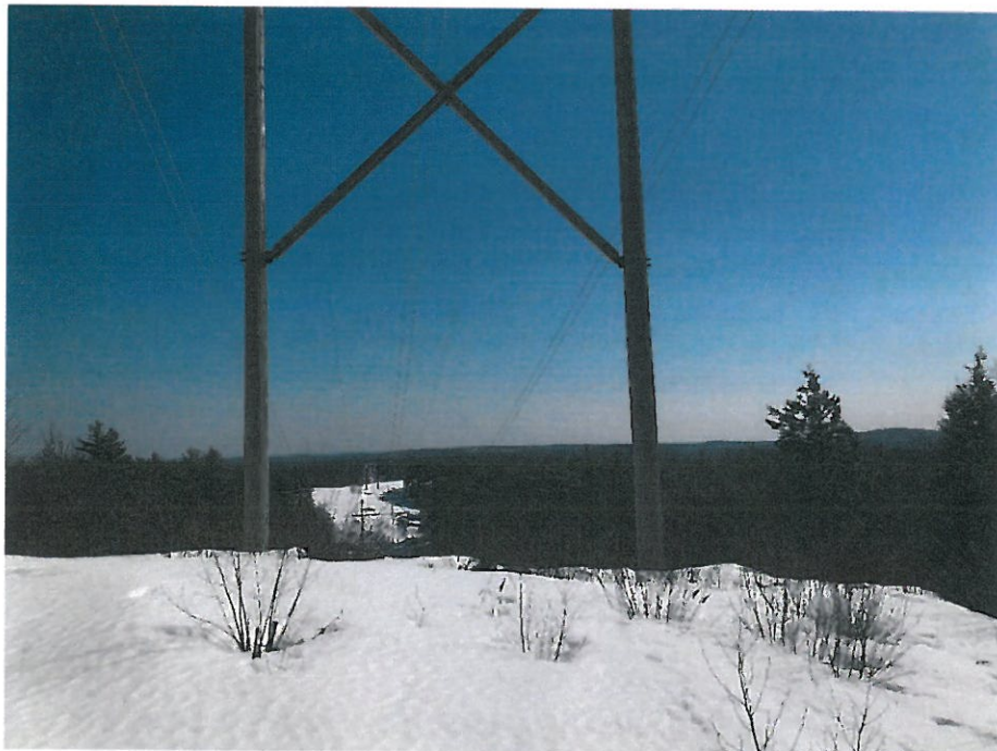
Photograph No. 14: Looking easterly at proposed work pad for Structure 288 to be replaced.
