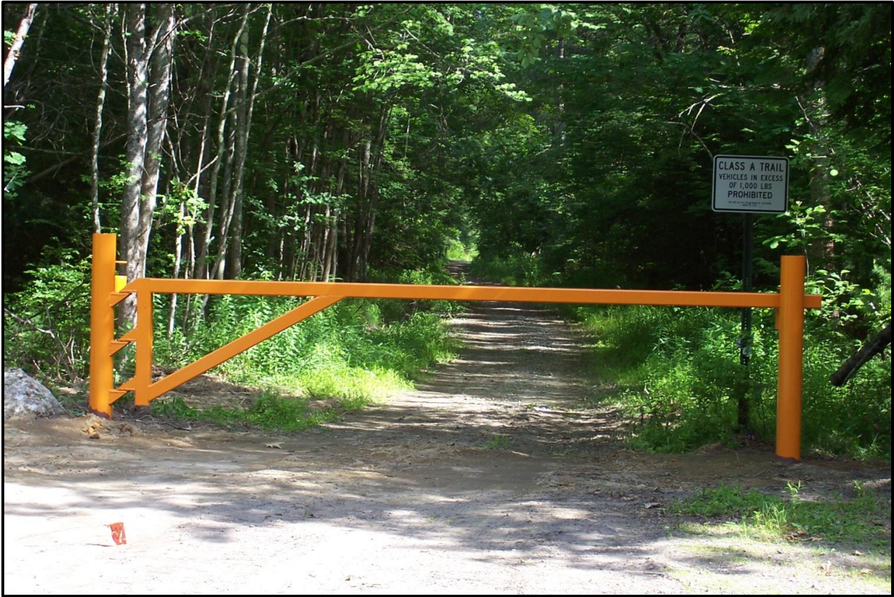
Proposed Southern Connector Trail – West Side Road Gate - Sample gate picture without pass-thru
