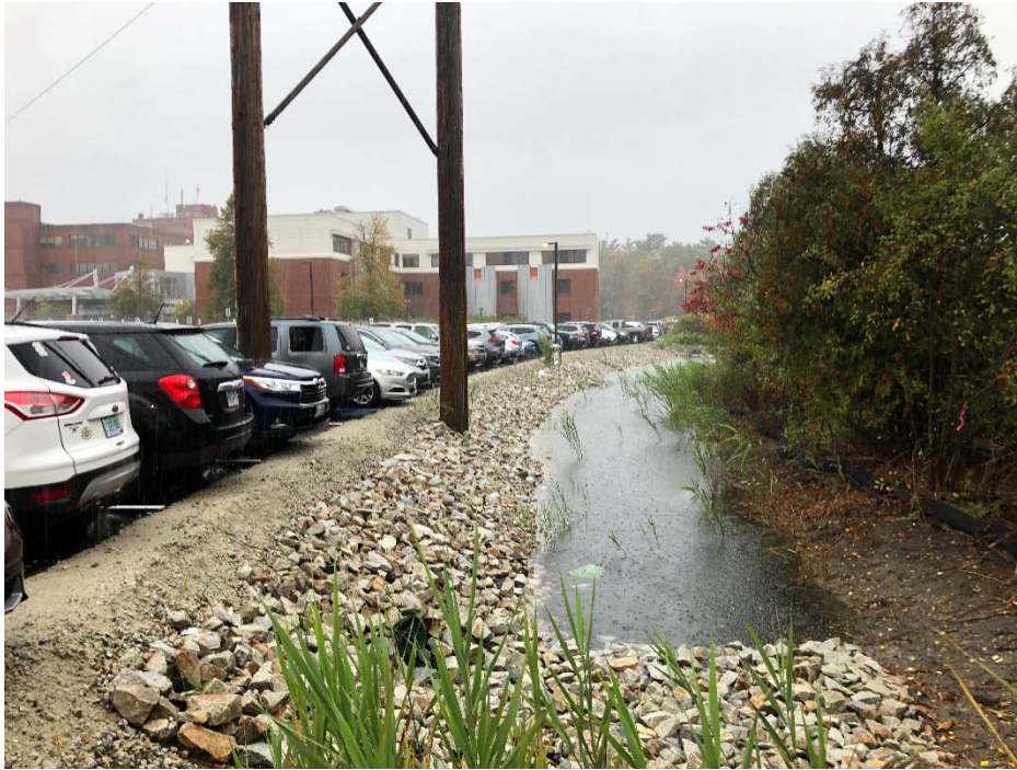
Photograph No. 9: Westerly view of Wetland PW-11 (right) and E194 Structure 36 to be replaced.
