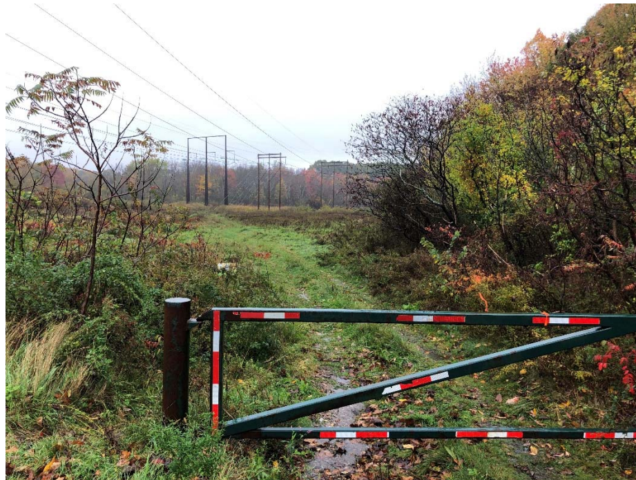
Photograph No. 10: Southeasterly view of proposed access from Greenland Road for 3135 Structure 105 and 106 to be replaced.
