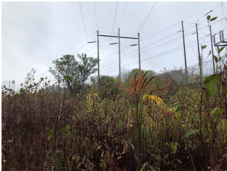
Photograph No. 4: Northeasterly view of E194 Structure 34 to be replaced within Wetland PW-11.
