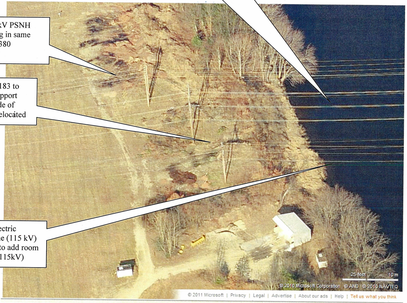
Figure 1. Closer View of Merrimack River Crossing (west side), Merrimack, NH. Note storage building is not on PSNH property and is just south of PSNH owned parcel (See Figure 3). A new substation will be built northerly of the parcel named Eagle Substation.
