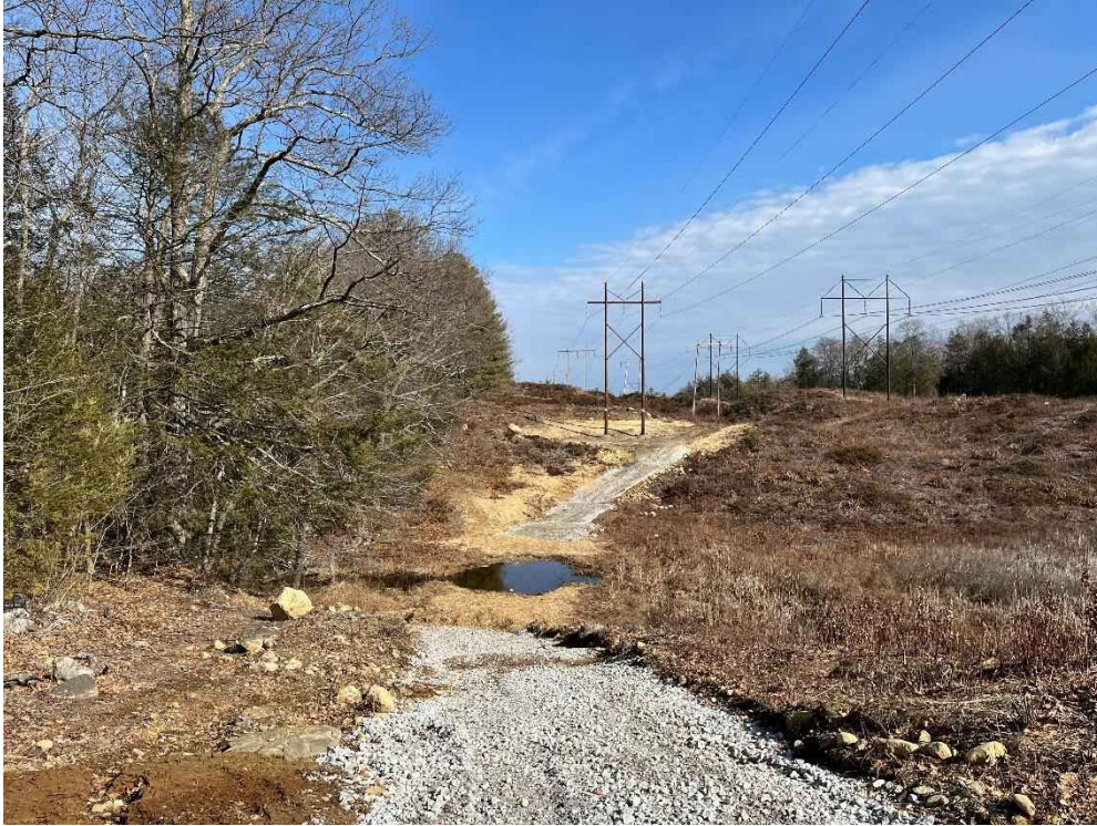
Photograph No. 11: Looking at proposed access to H141 Structure 307.
