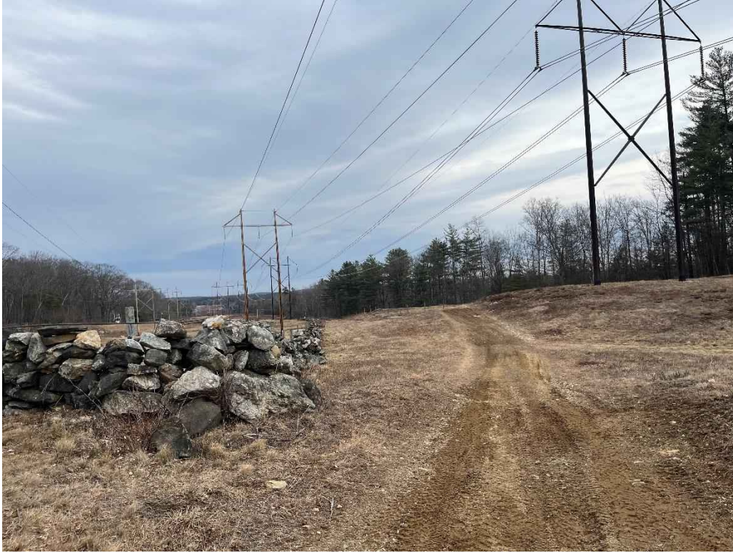
Photograph No. 7: Looking at proposed access and work pad location for H141 Structure 312 (left).
