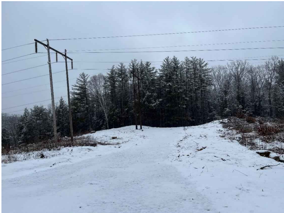
Photograph No. 24: Looking at proposed access and work pad location for H141 Structure 287.
