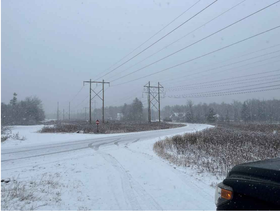
Photograph No. 13: Looking at proposed access and work pad location for H141 Structure 299 (right), from Pheasant Run Drive.
