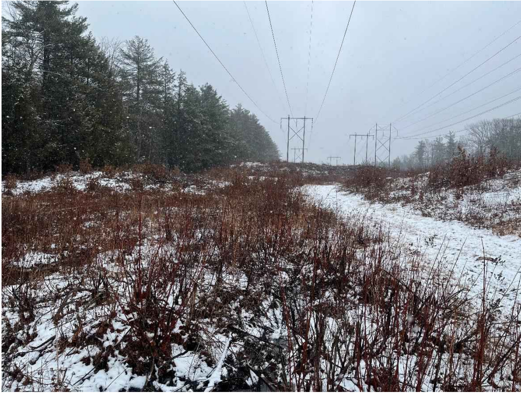
Photograph No. 29: Looking at proposed access to H141 Structure 282.
