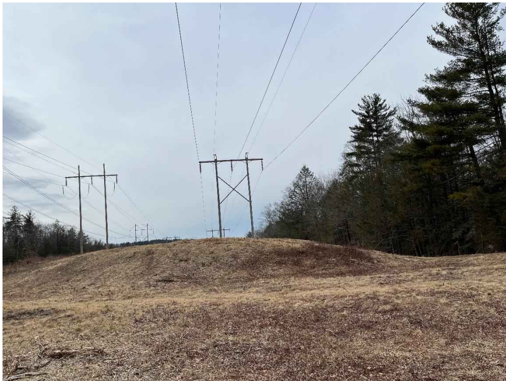
Photograph No. 6: Looking at proposed access and work pad location for R193 Structure 348 (right).
