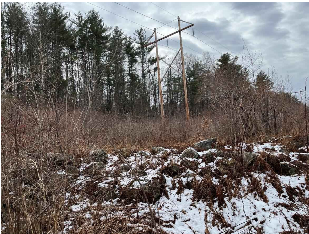
Photograph No. 40: Looking at proposed access and work pad for H141 Structure 262, facing south from the base of R193 Structure 291.
