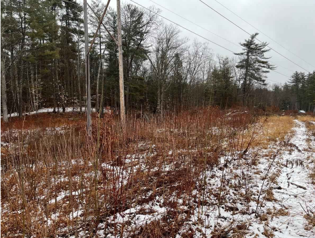
Photograph No. 35: Looking at proposed access and work pad locations for R193 Structure 306 (left) and H141 Structure 274 (right).
