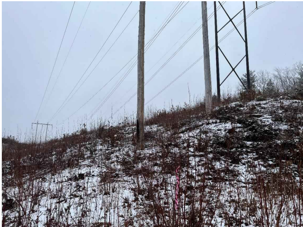
Photograph No. 26: Looking at proposed access and work pad location for H141 Structure 285.
