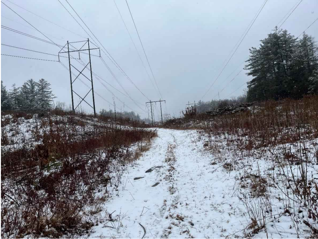
Photograph No. 27: Looking at proposed access to H141 Structure 284, facing west towards 363 Structure 154.
