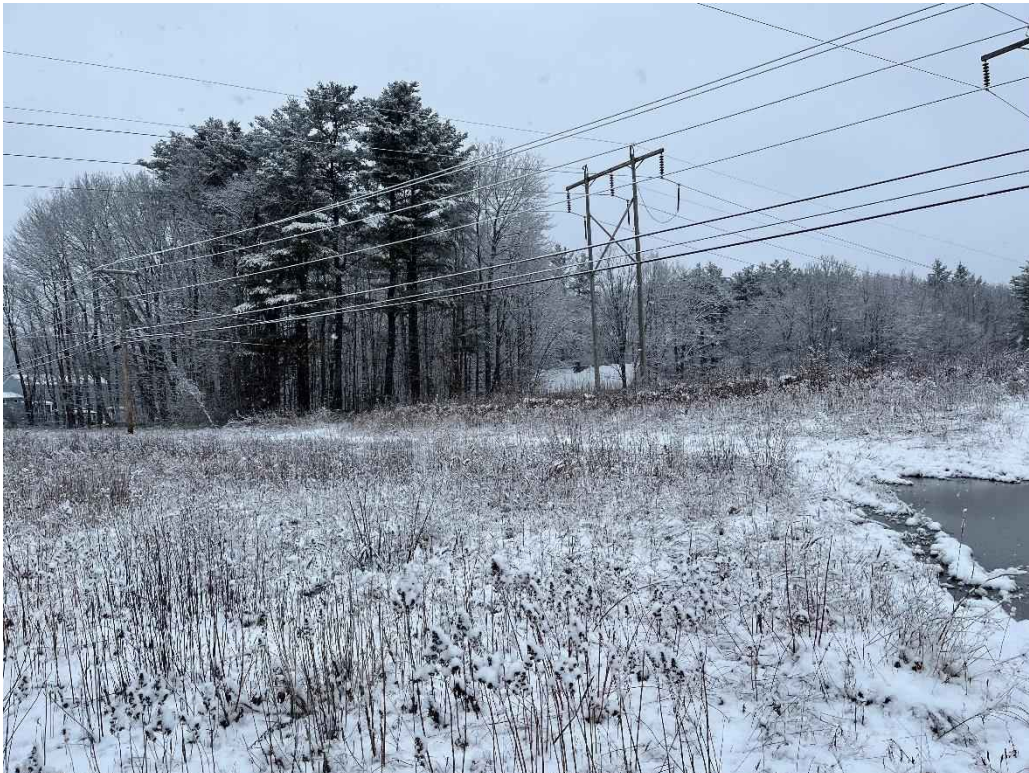
Photograph No. 20: Looking at proposed access and work pad location for R193 Structure 325.
