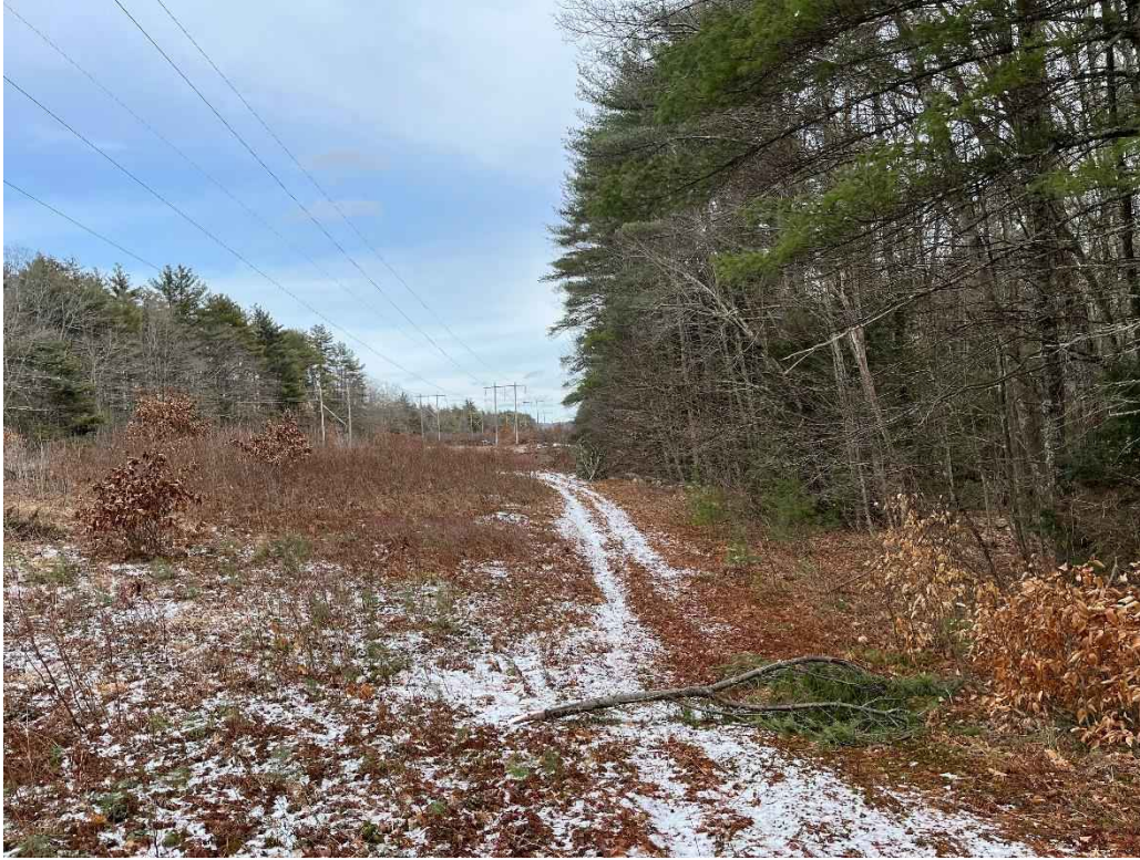
Photograph No. 41: Looking at proposed access adjacent to H141 Structure 261 (left).
