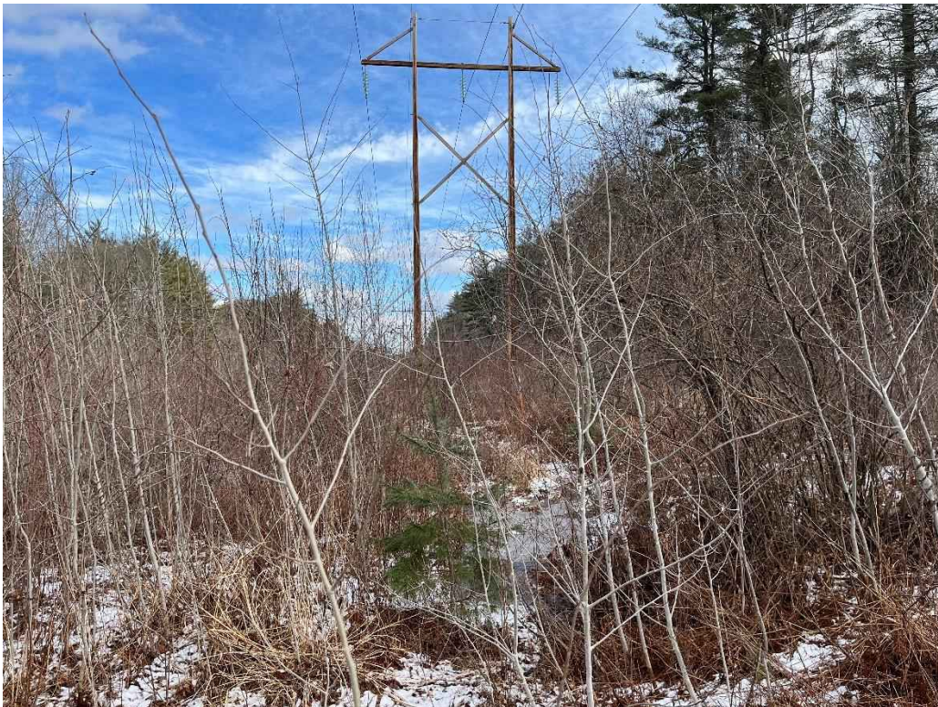
Photograph No. 38: Looking at proposed access to H141 Structure 263.
