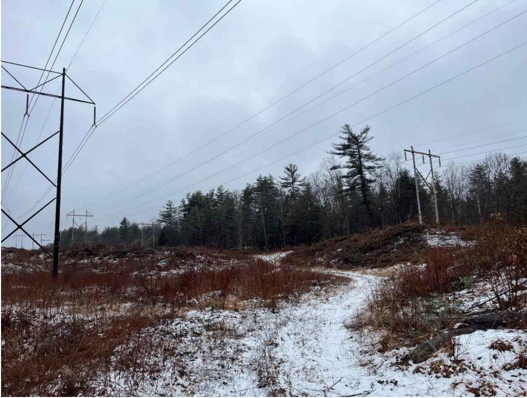
Photograph No. 33: Looking at proposed access and work pad location for R193 Structure 305 (right).
