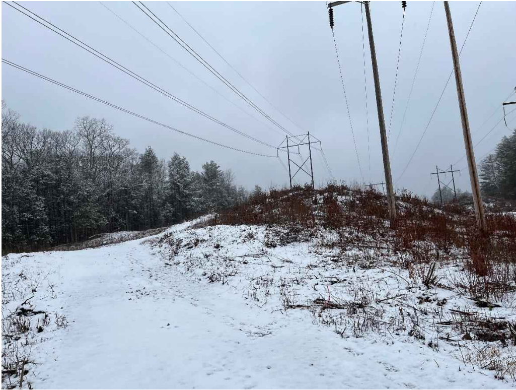
Photograph No. 25: Looking at proposed access and work pad location for H141 Structure 286.
