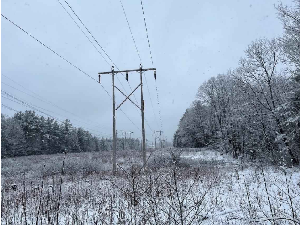
Photograph No. 17: Looking at proposed access and work pad location for R193 Structure 326.
