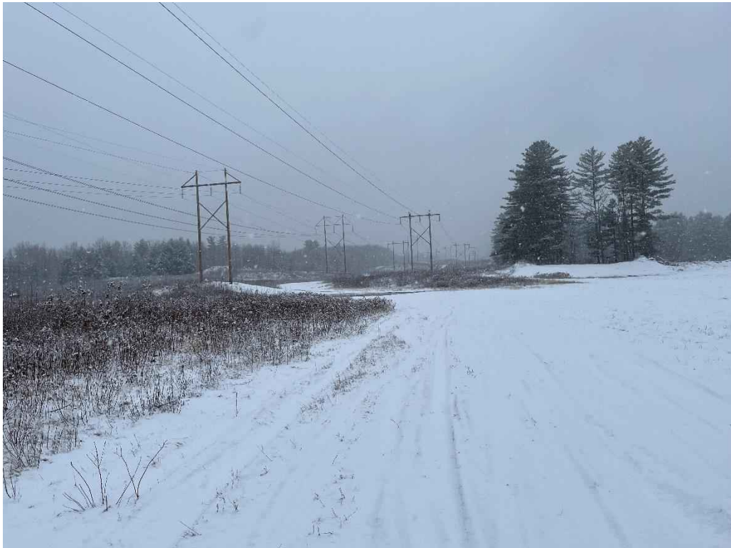
Photograph No. 14: Looking at proposed access and work pad location for H141 Structure 300 (left).
