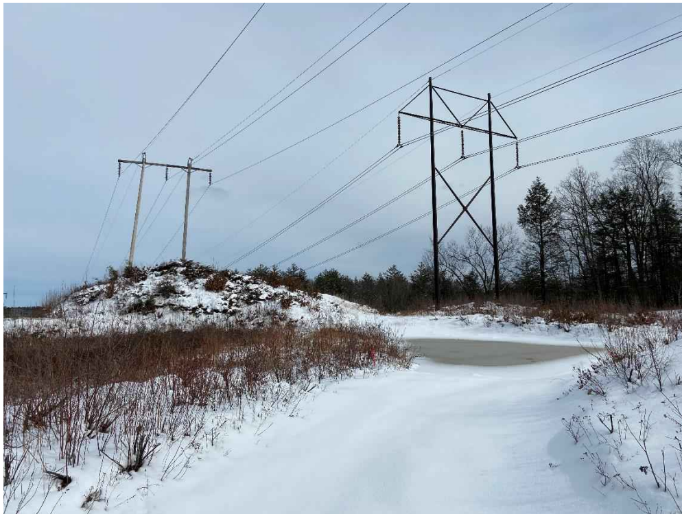
Photograph No. 12: Looking at proposed access for H141 Structure 306.
