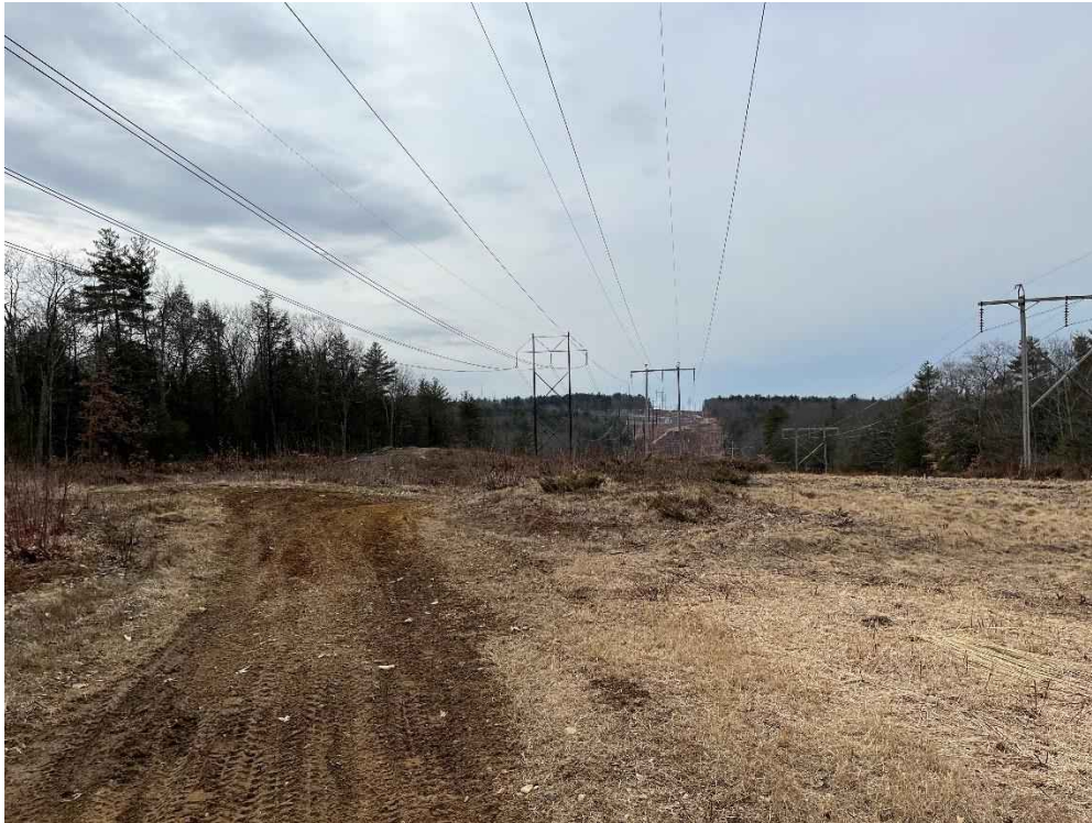
Photograph No. 5: Looking at proposed access and work pad location for R193 Structure 349 (right), adjacent to H141 Structure 314.
