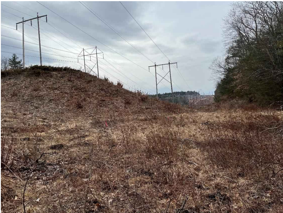
Photograph No. 4: Looking at proposed access and work pad location for R193 Structure 349, facing south-southwest towards H141 Structure 315.
