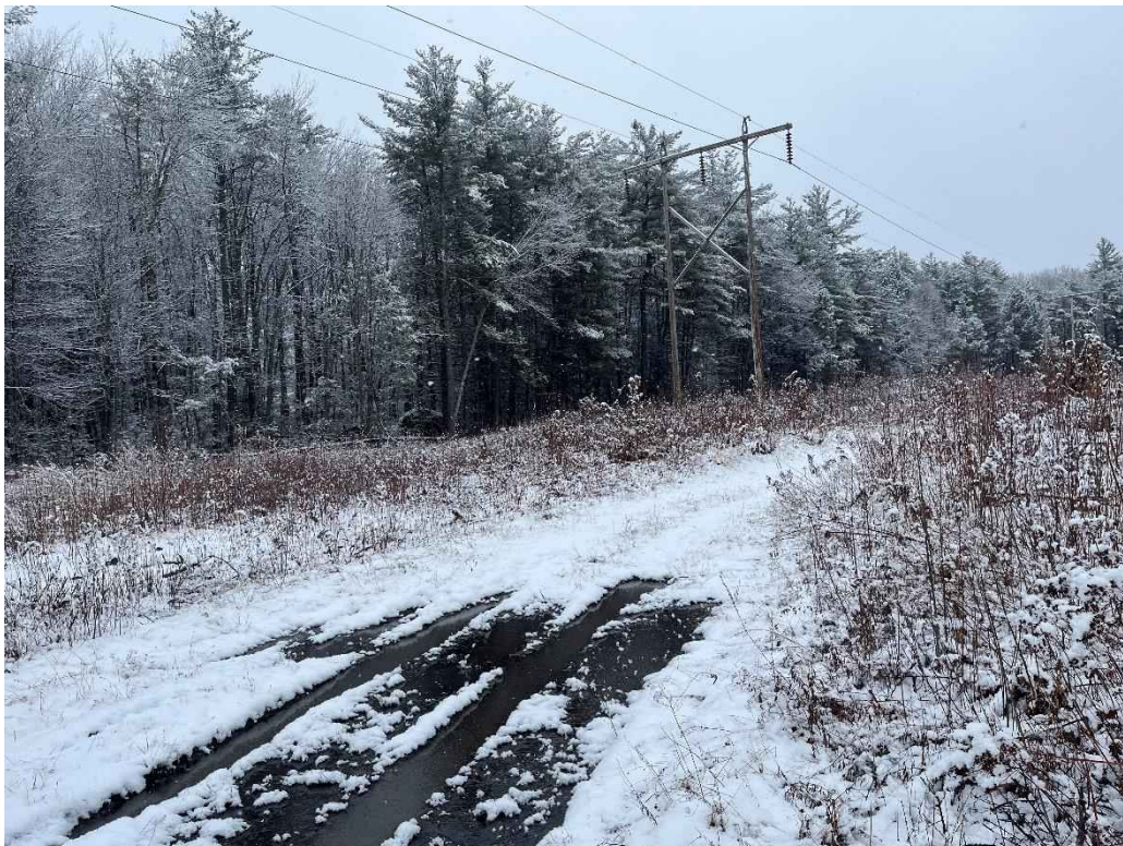
Photograph No. 22: Looking at proposed access and work pad location for R193 Structure 324.
