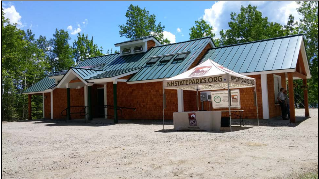
Broad view of the new accessible facilities prior to the grand opening ceremonies. Dishwashing station to left; toilets, shower, laundry in center; concessions to right
