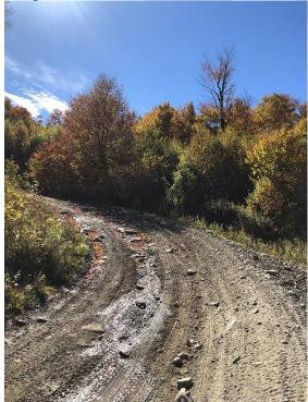
Figure 9- Shows berm on corner of trail
