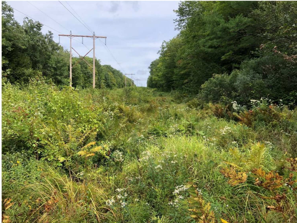
Photograph No. 9: Looking at proposed access and work pad at Structure 174.
