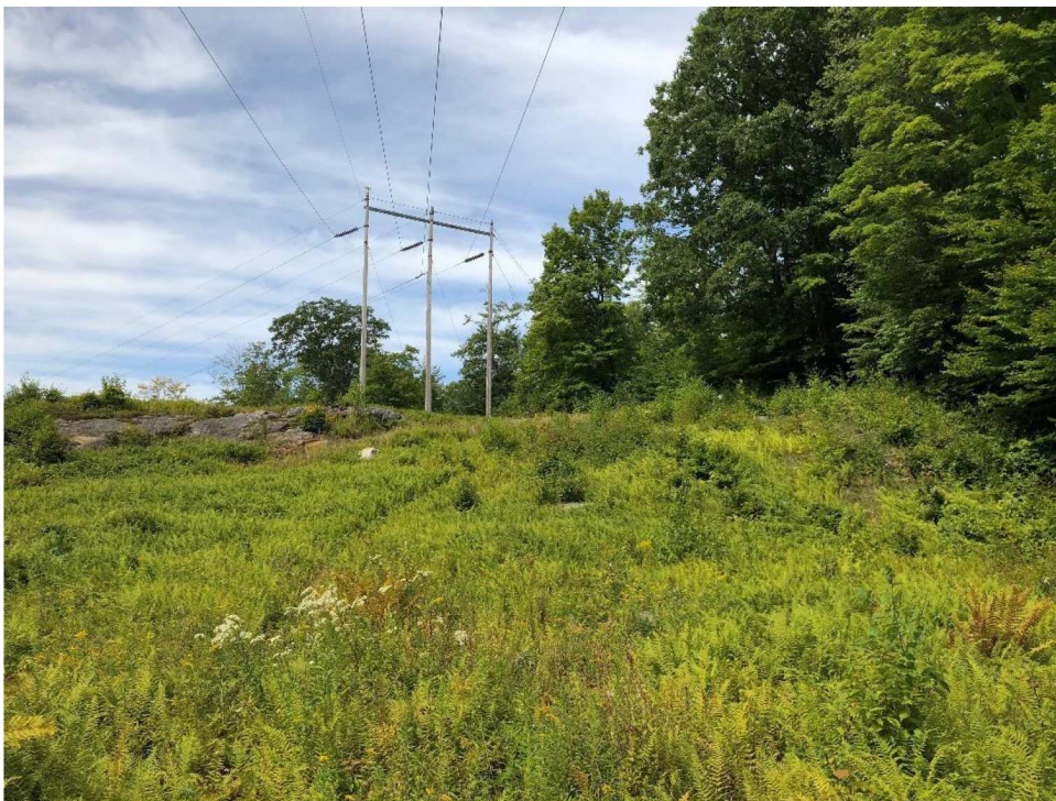
Photograph No. 28: Looking at proposed work pad and access at Structure 180.
