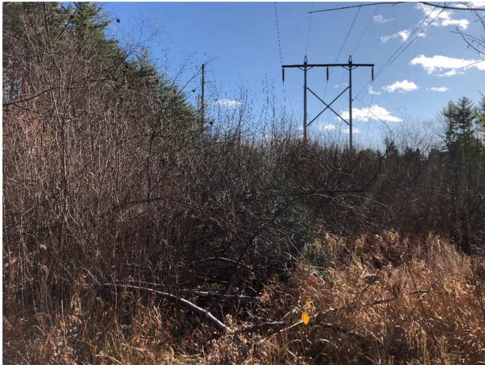
Photograph No. 6: Looking at proposed access and proposed structure replacement structure 208.
