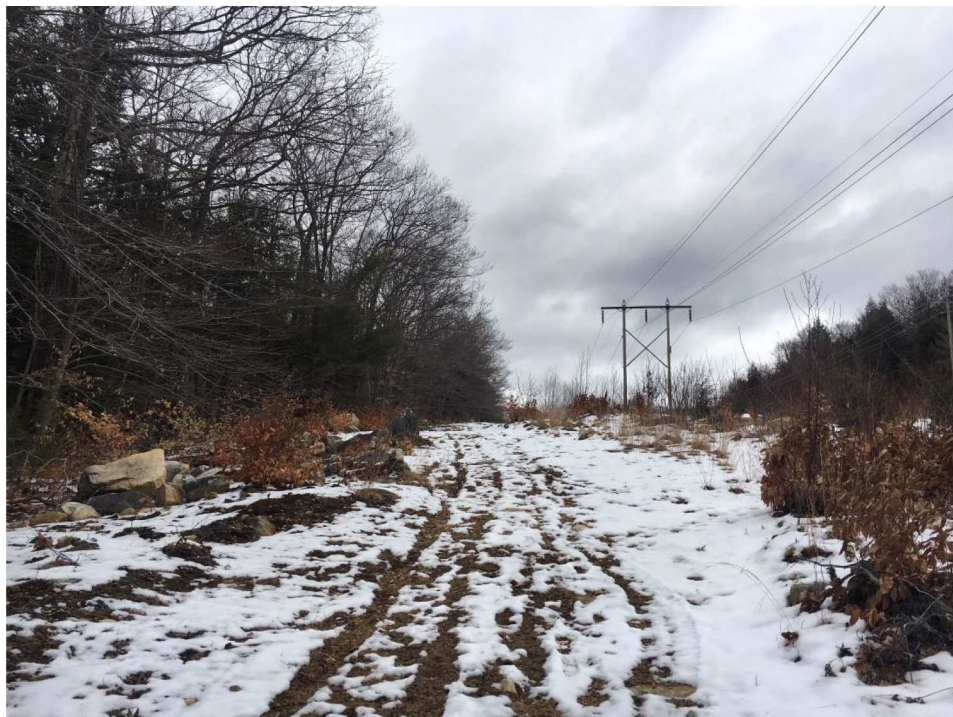
Photograph No. 20: Looking at proposed access toward Structure 188 off Old Gilsum Road.
