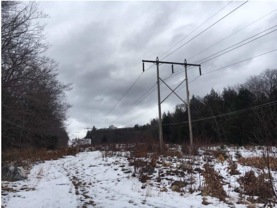
Photograph No. 21: Looking at proposed access and work pad at Structure 188.
