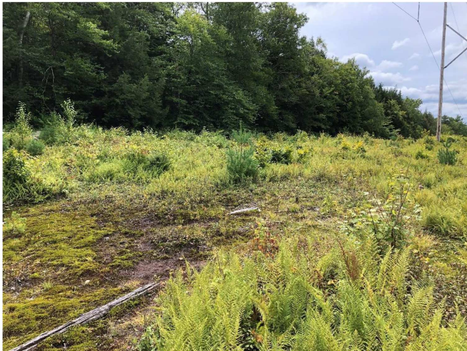
Photograph No. 18: Looking at proposed work pad at Structure 169.
