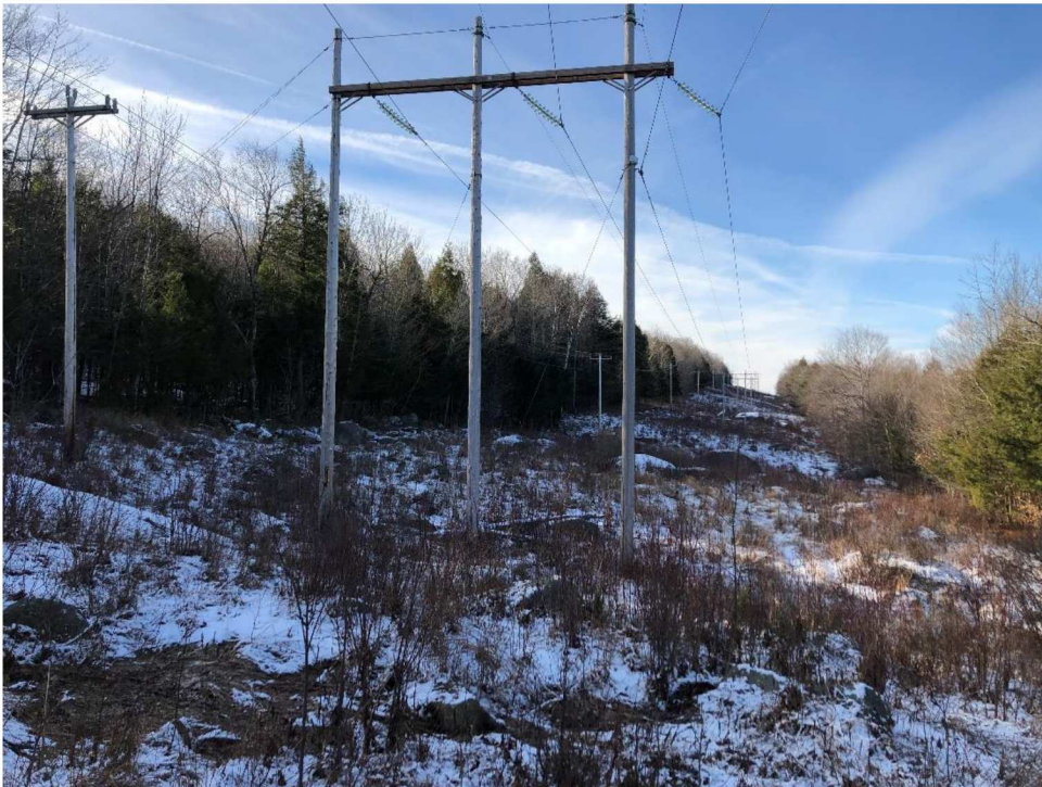
Photograph No. 38: Looking at proposed work pad and access at Structure 9.
