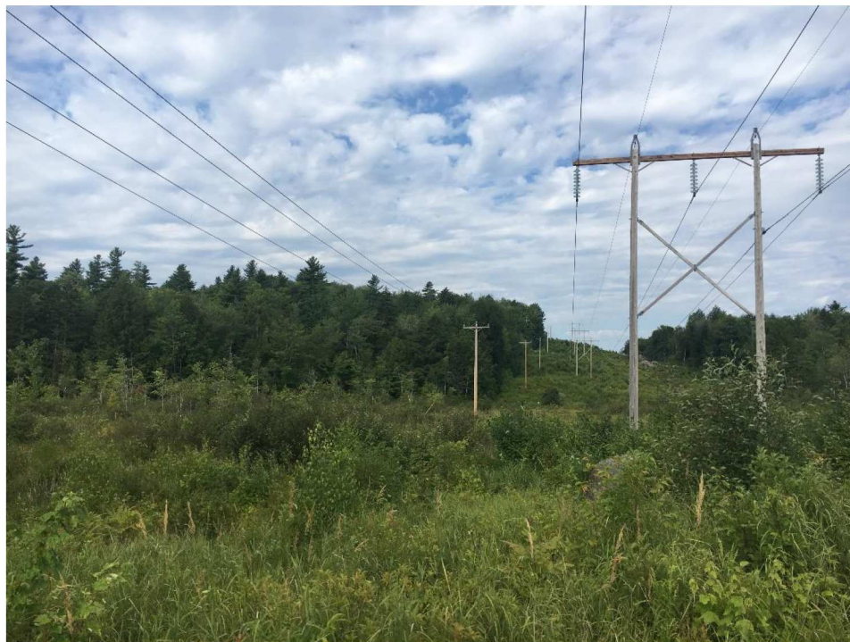
Photograph No. 30: Looking at proposed access adjacent to Structure 24.
