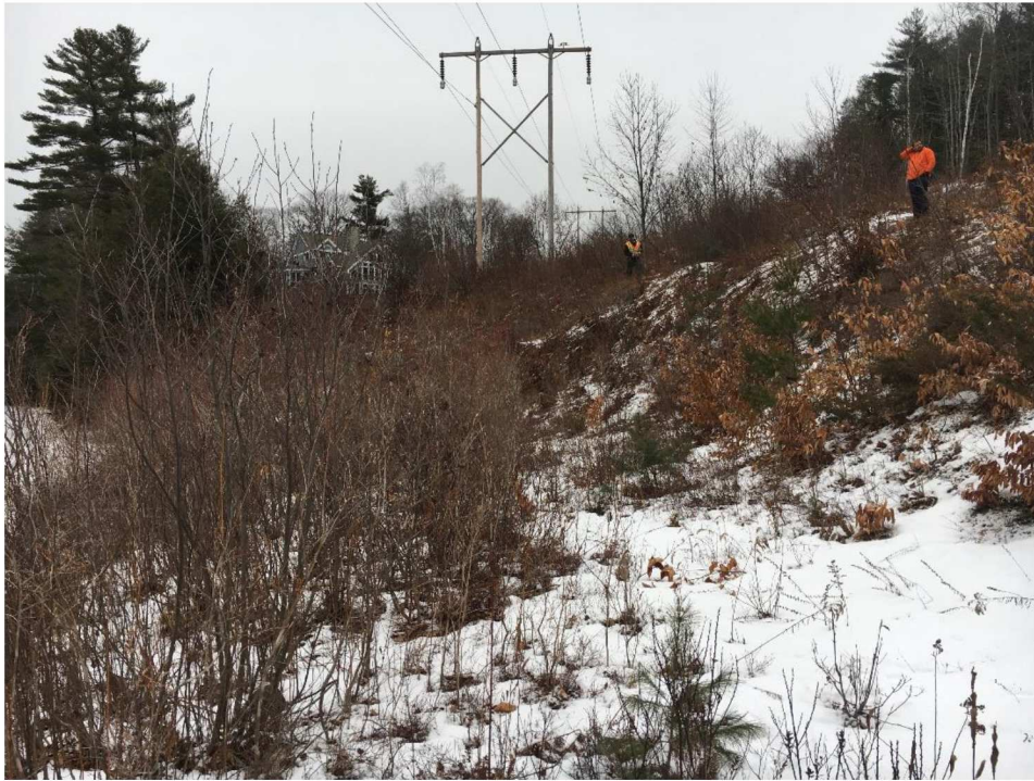
Photograph No. 43: Looking at proposed work pad and access to Structure 44 (X104 Line).
