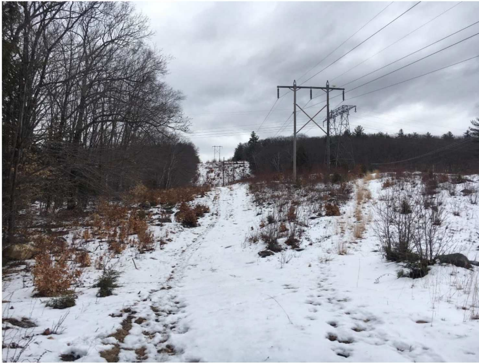
Photograph No. 23: Looking at proposed access and work pad at Structure 187.
