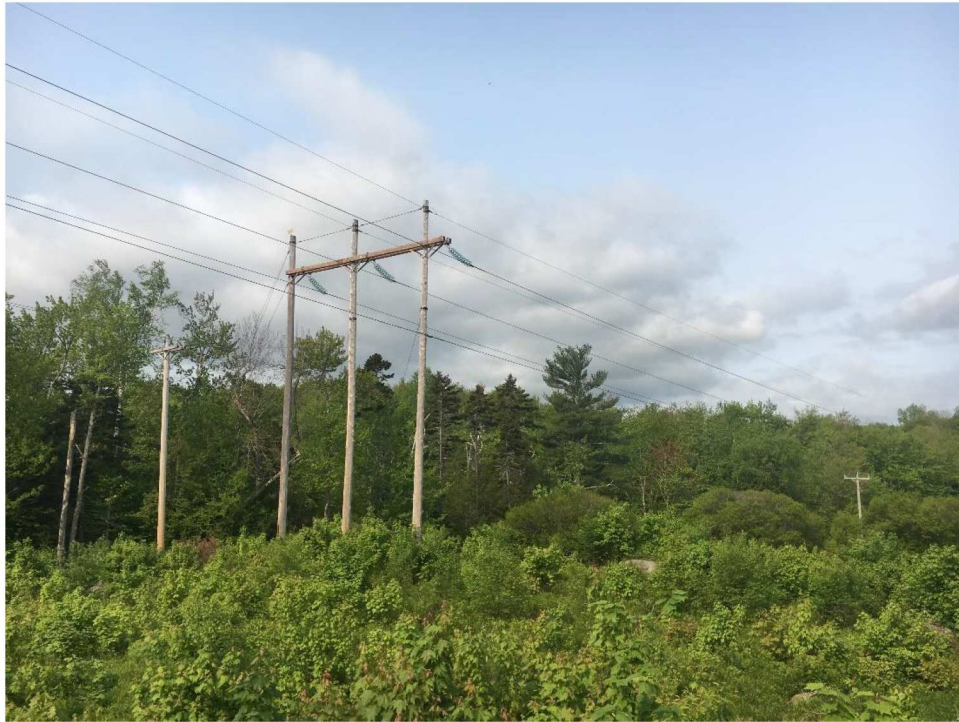
Photograph No. 29: Looking at proposed work pad at Structure 30.
