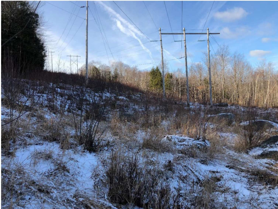
Photograph No. 40: Looking at proposed access and work pad between Structure 3 and 4.
