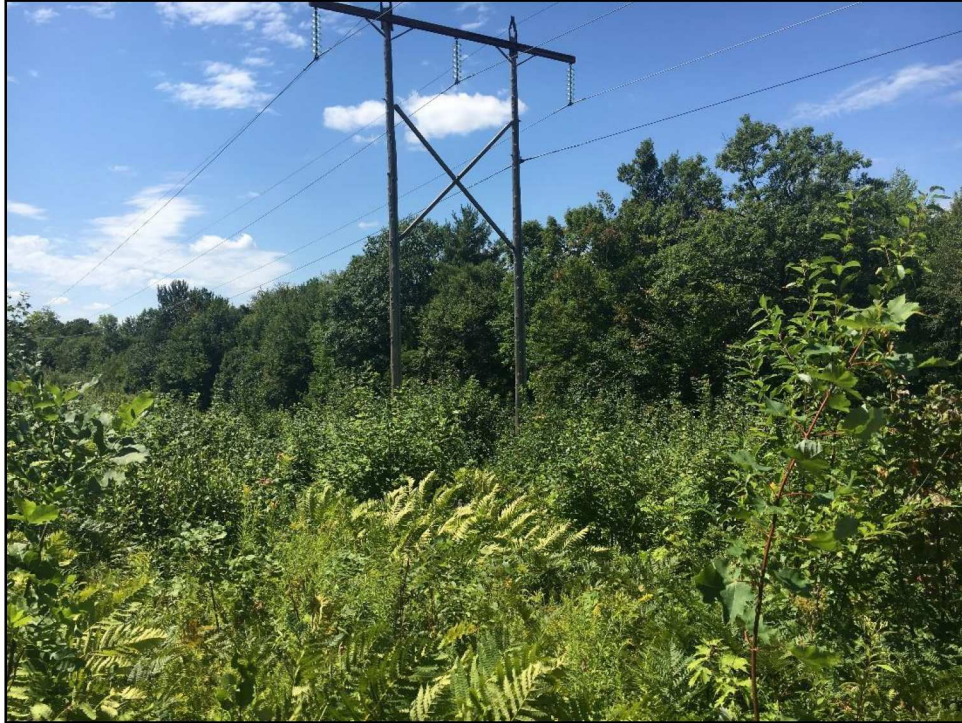
Photograph No. 39: Looking at proposed access adjacent to Structure 7.
