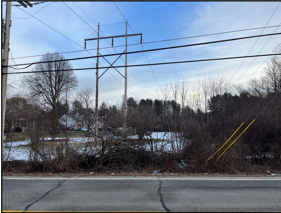
Photo 1: View northeast at proposed access location along Garrison Road adjacent to Structure 44.
