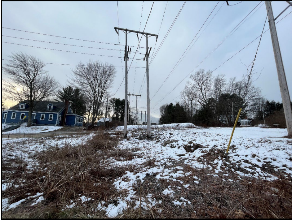
Photo 5: View north along transmission line ROW from Dover Point Road to Old Dover Point Road at Structure 57, which is proposed to be replaced as part of the Project.
