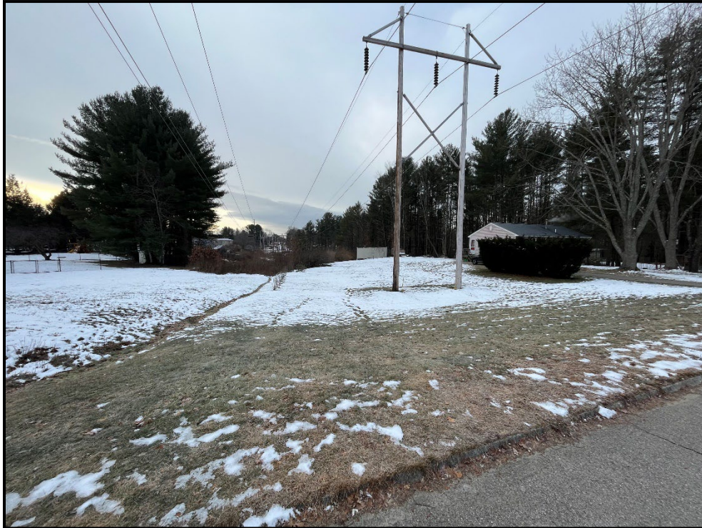
Photo 7: View south of proposed matting location off Toftree Lane at Structure 59 which is proposed to be replaced as part of the Project.
