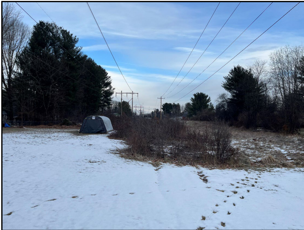
Photo 8: View north along transmission line ROW off Toftree Lane toward Structure 60.
