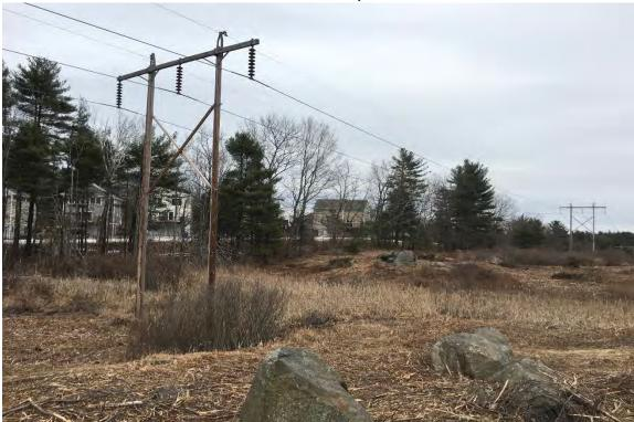
Photo 1. View northeast at Structure 176 (A126 Line) to be replaced within Wetland EW-16 located adjacent to Watson Road.
