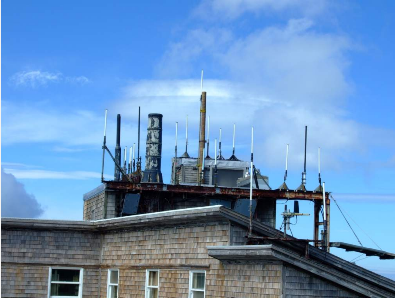
Penthouse Roof Antennas
