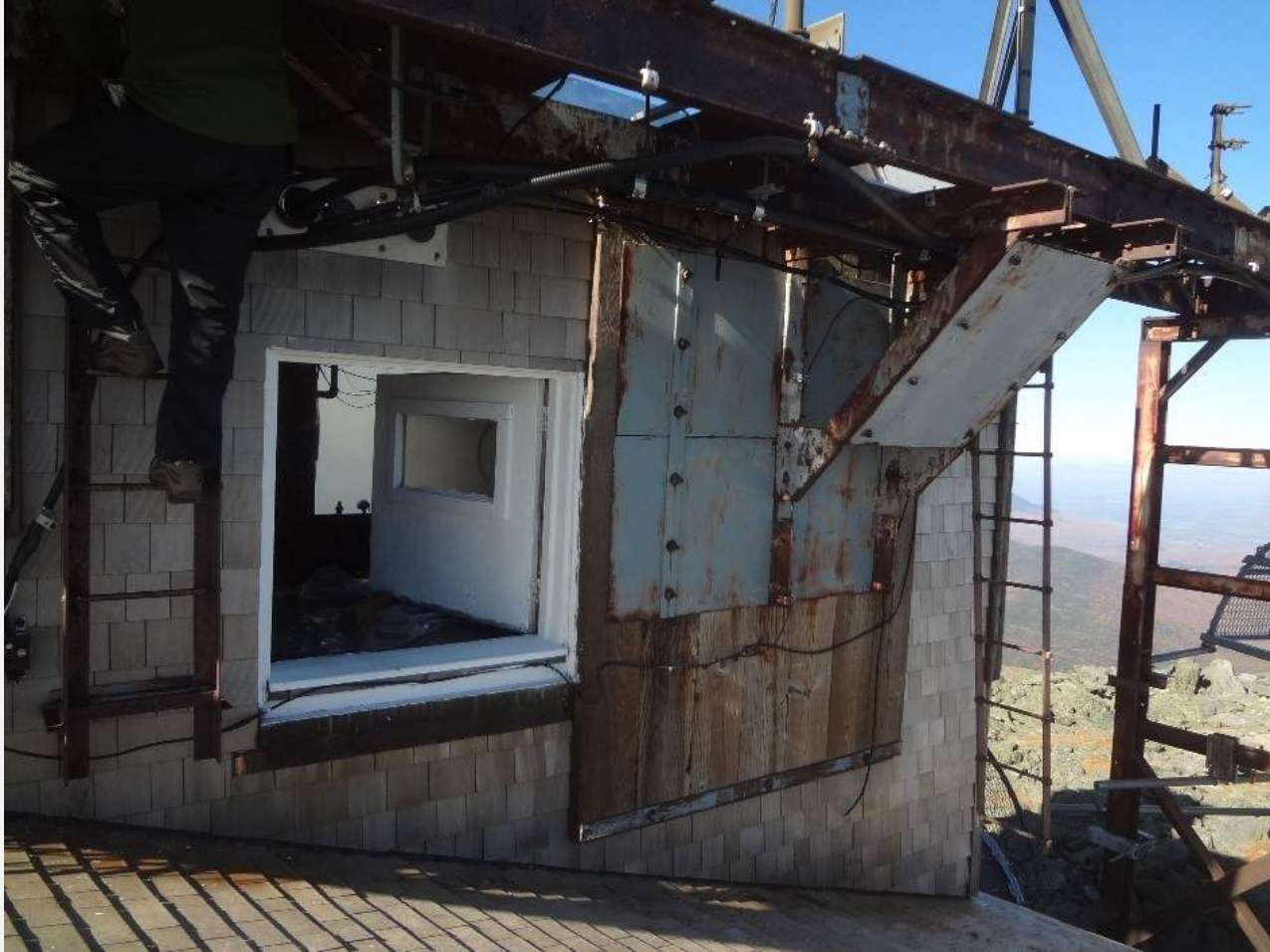
Access To Penthouse
