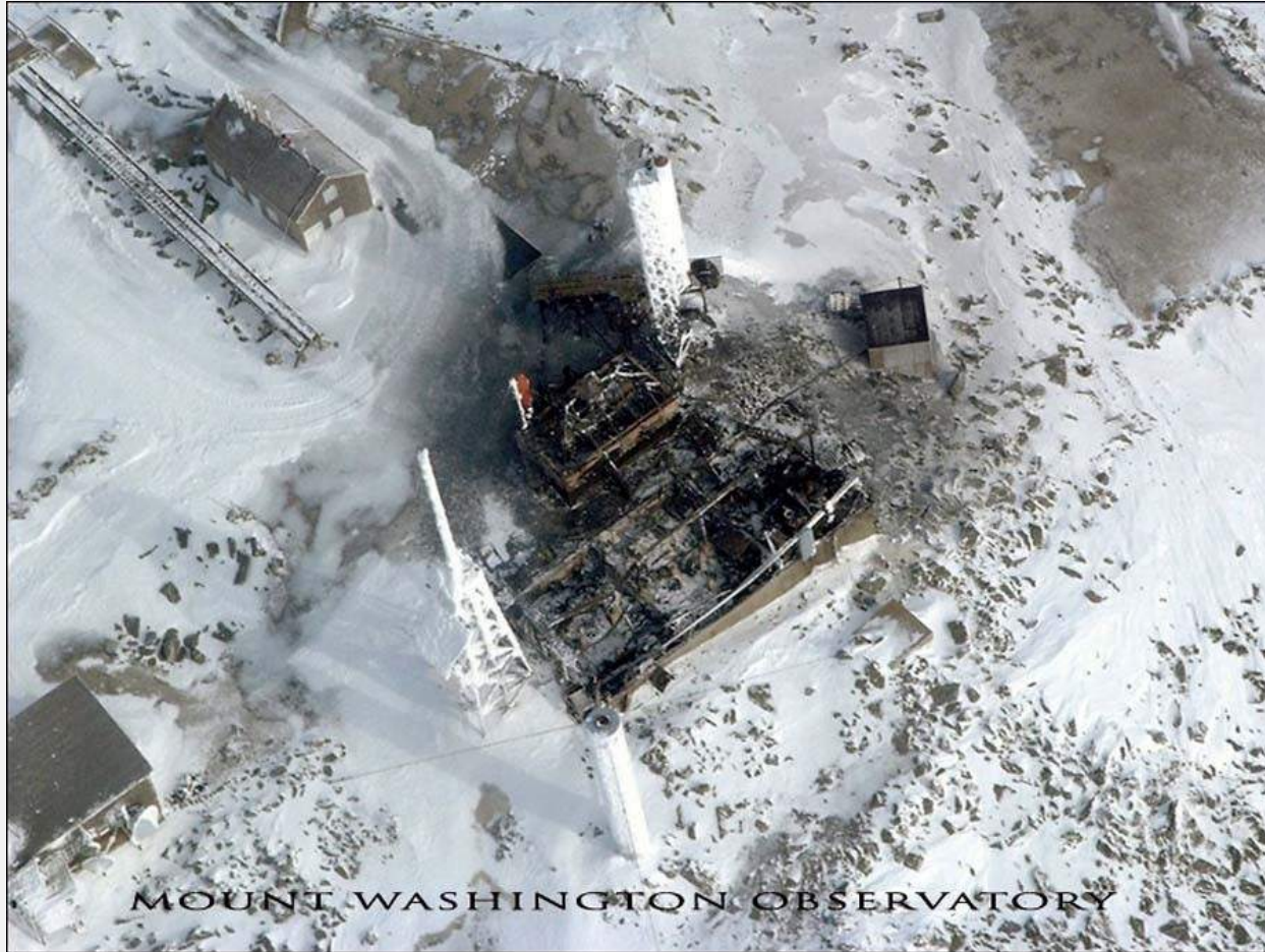
Old Generator Building Fire 2003
