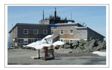
The Yankee Building supports many systems of State and national importance. However, the building is currently in a State of disrepair. {In recent times, the Yankee Building has suffered from leaking roofs, poor insulation, disjointed work areas, and a general condition that is far below acceptable levels for public buildings.} The Commission shall conduct further studies to determine how to properly provide an up-to-date communications and maintenance
