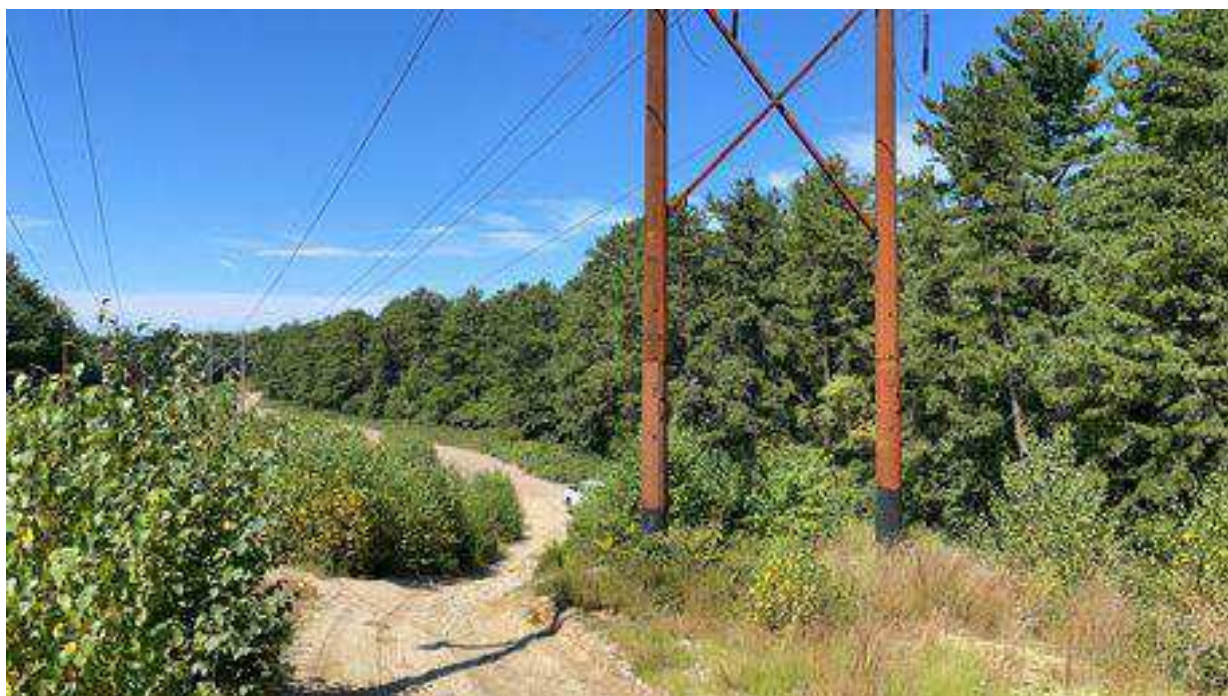
Photo 13. Str. 54 future work area, viewing northwest.
