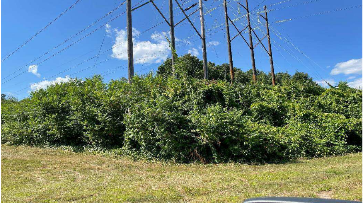
Photo 37. Str. 70 future work area, viewing from highway.
