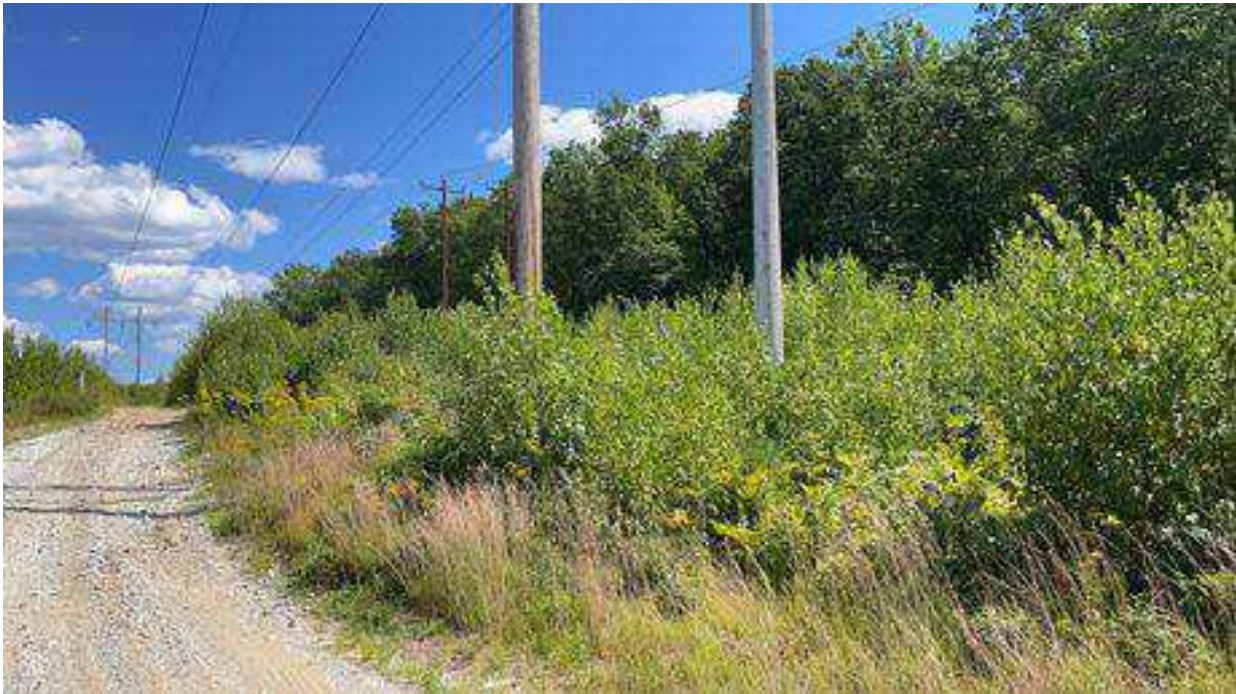
Photo 24. Str. 61 future work area, viewing southeast.
