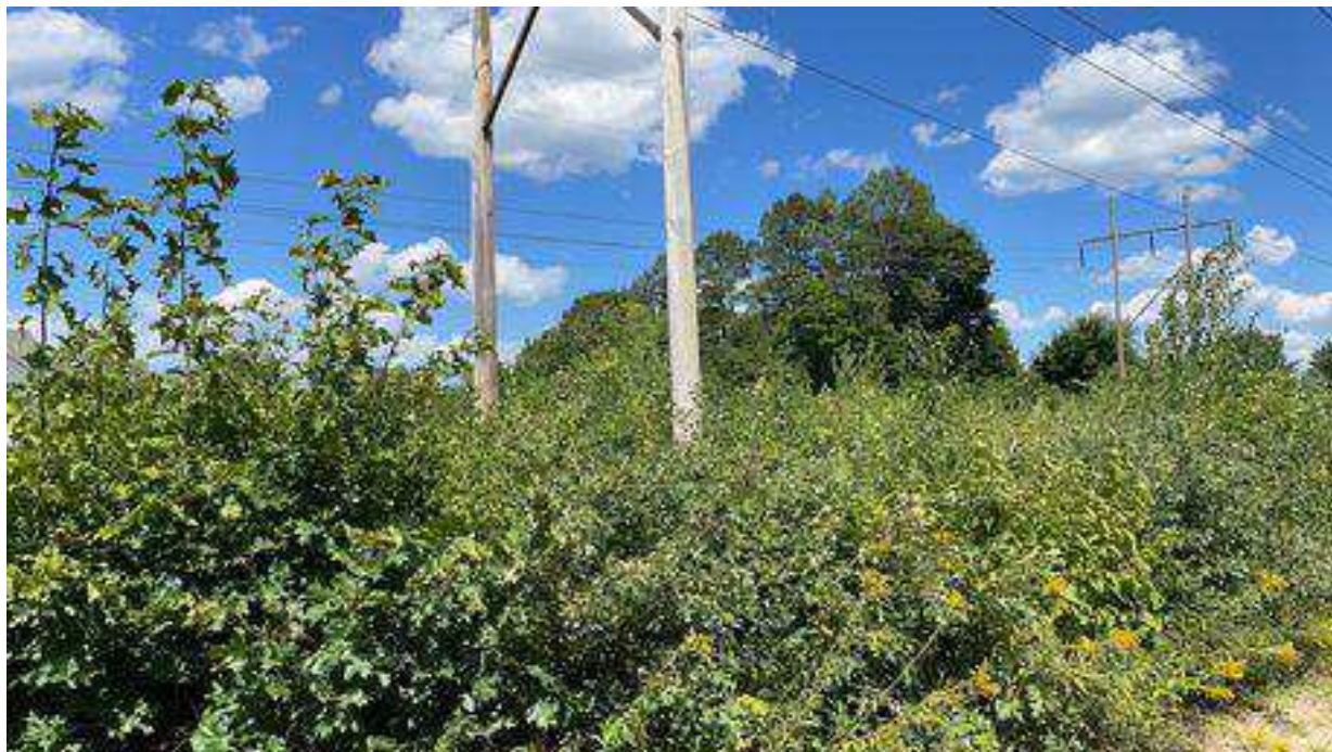
Photo 27. Str. 63 future work area, viewing northeast.
