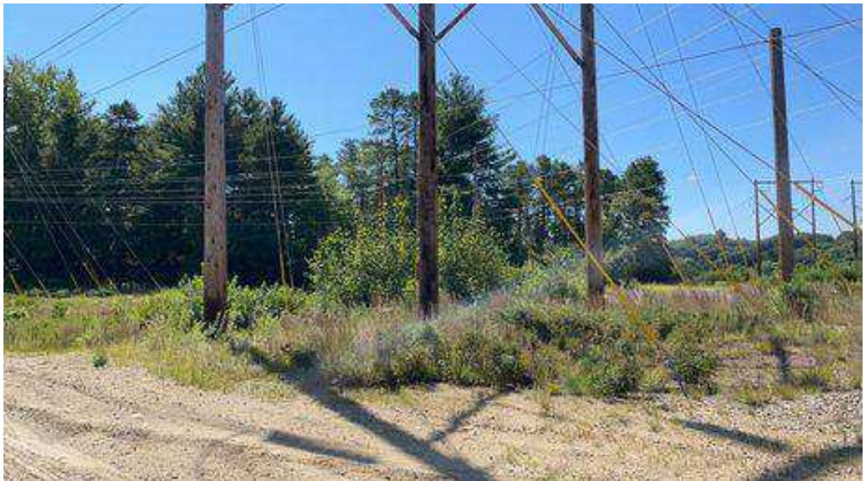
Photo 7. Str. 51.3 future work area, viewing south.
