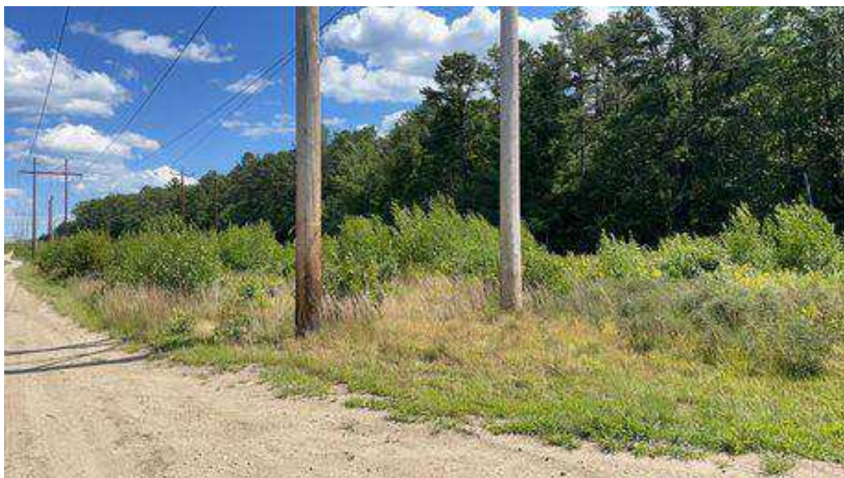
Photo 22. Str. 59 future work area, viewing southeast.
