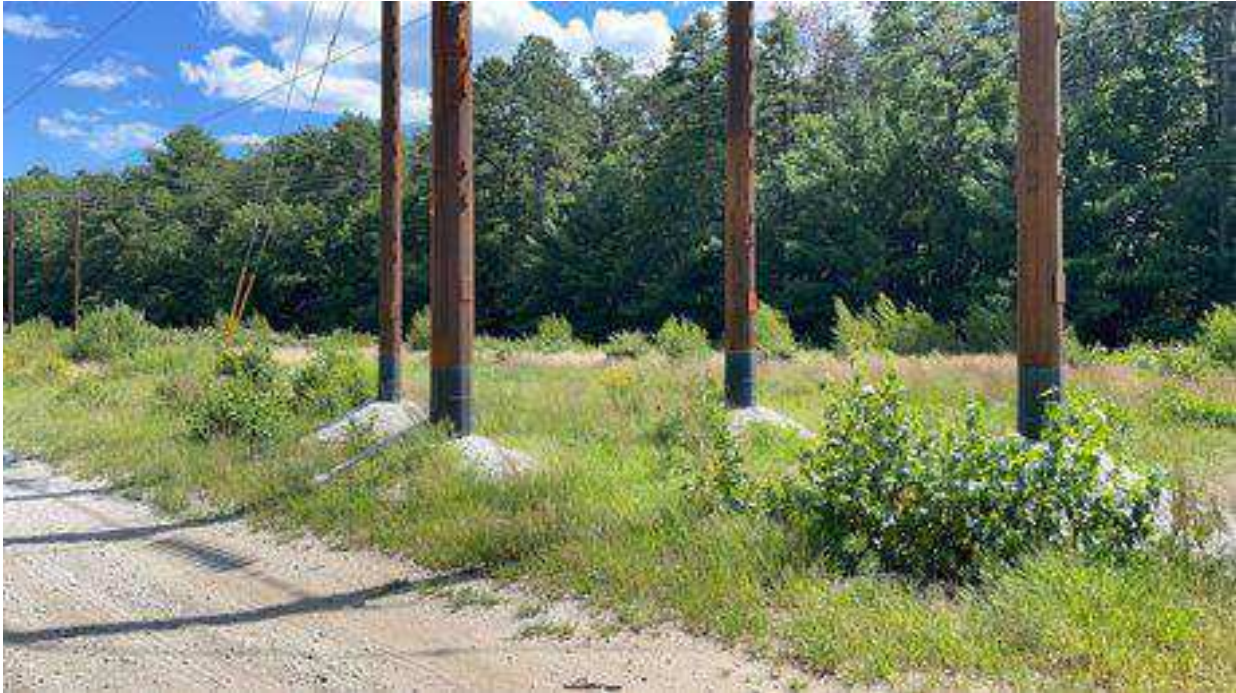
Photo 23. Str. 60 future work area, viewing southeast.
