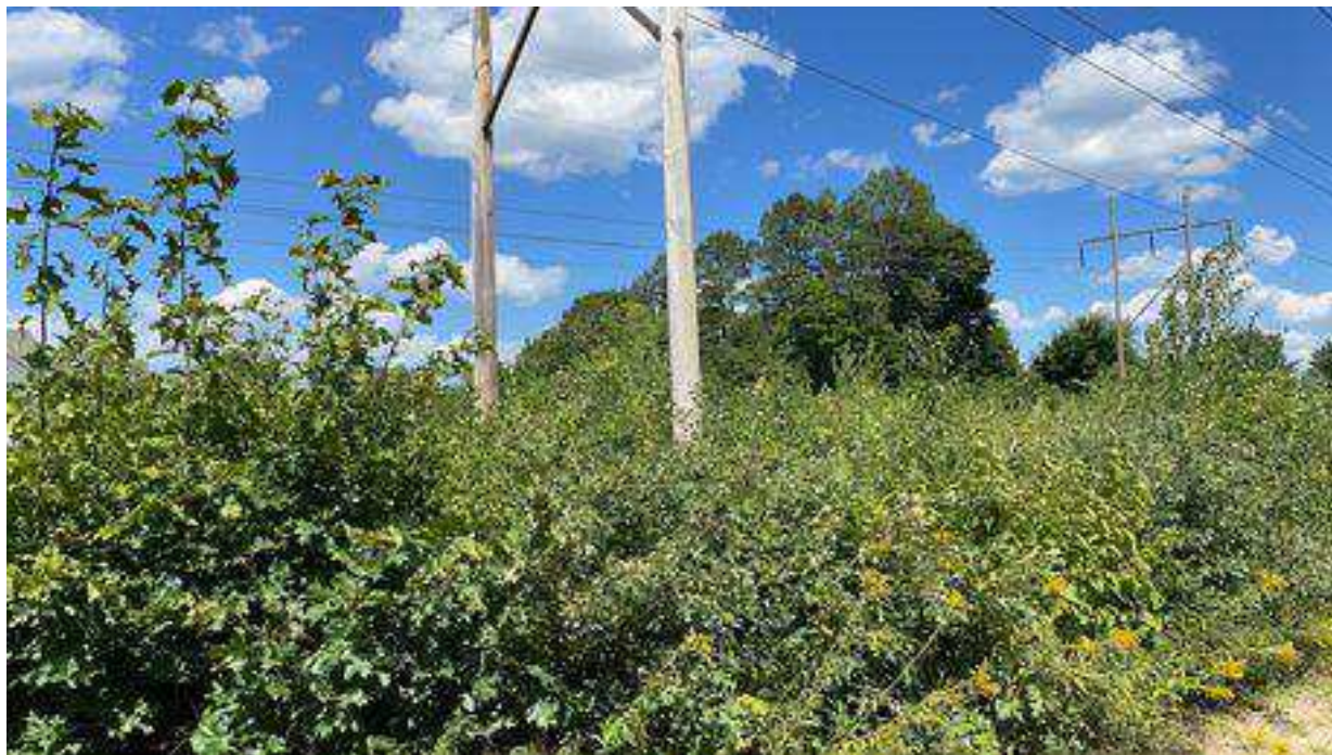
Photo 27. Str. 63 future work area, viewing northeast.
