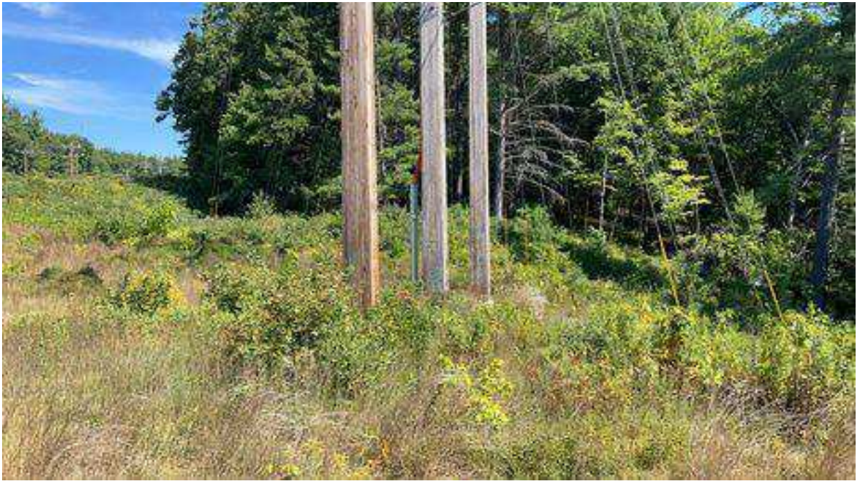
Photo 1. Str. 50 future work area, viewing northeast.
