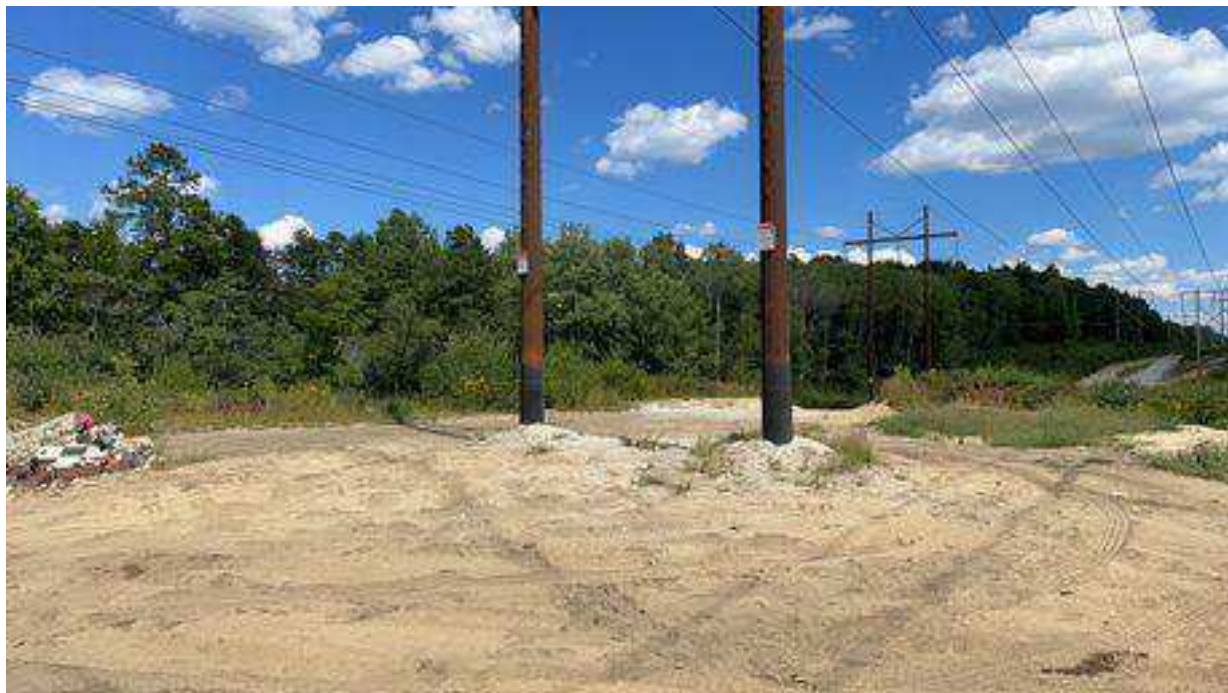
Photo 19. Str. 57 future work area, viewing east.
