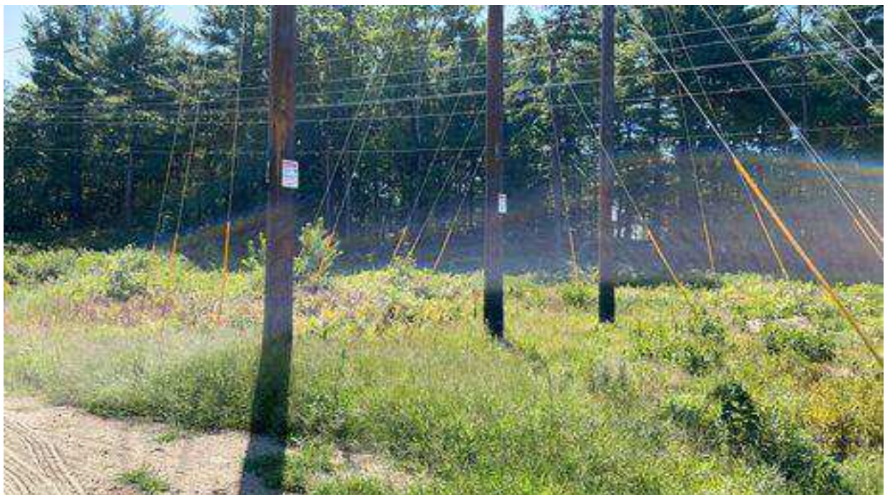
Photo 9. Str. 52 future work area, viewing south.
