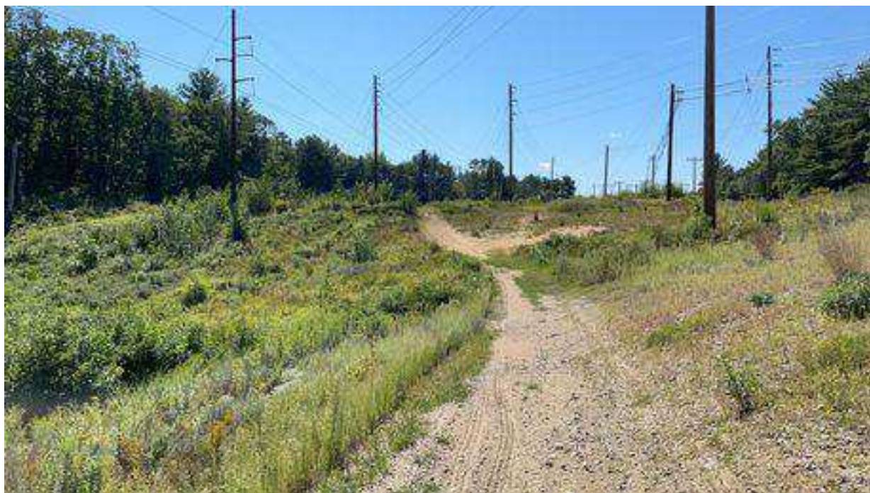
Photo 3. Proposed access road between Strs. 50 and 51.3, viewing south.
