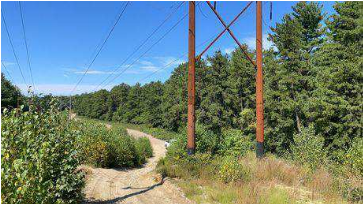
Photo 13. Str. 54 future work area, viewing northwest.
