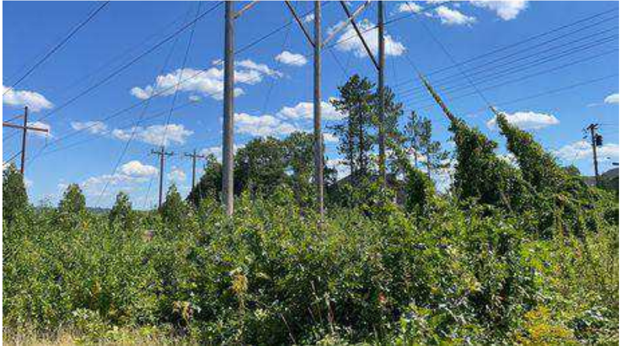
Photo 35. Str. 68 future work area, viewing southeast.
