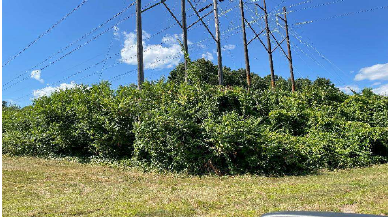
Photo 37. Str. 70 future work area, viewing from highway.
