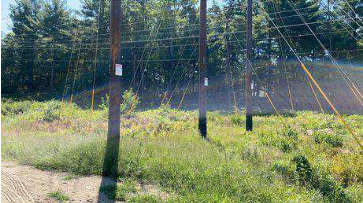
Photo 9. Str. 52 future work area, viewing south.
