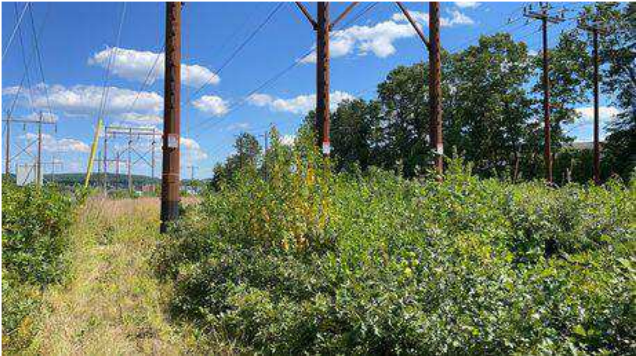
Photo 34. Str. 67 future work area, viewing southeast.
