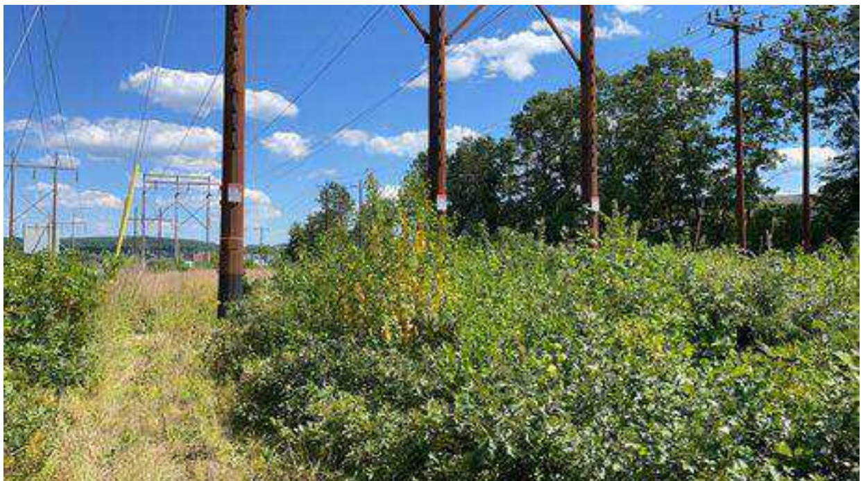
Photo 34. Str. 67 future work area, viewing southeast.
