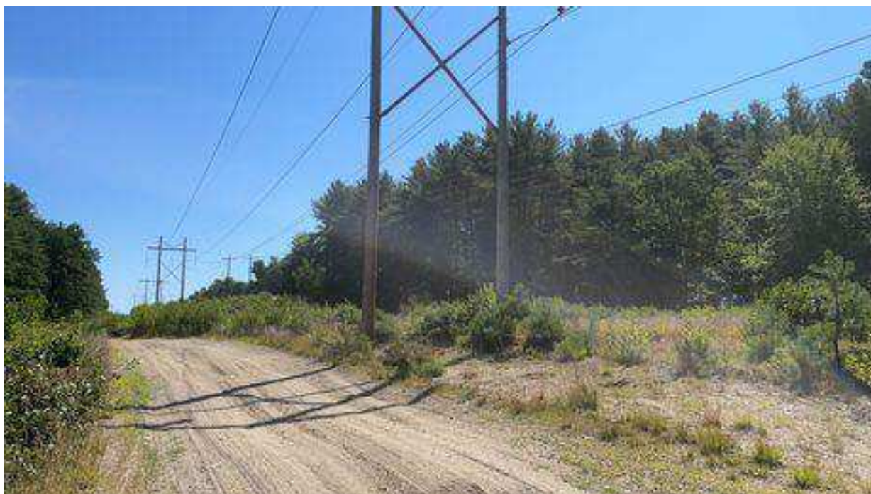
Photo 11. Str. 53 work area, viewing southeast.
