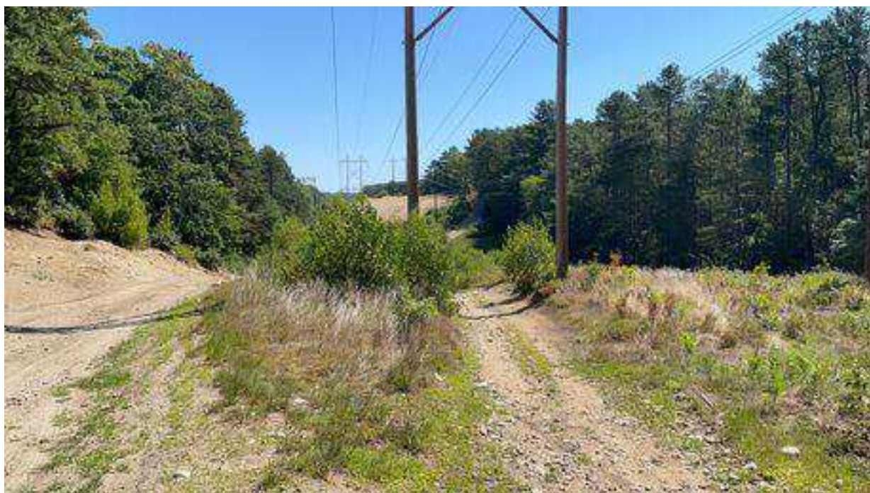
Photo 15. Str. 55 future work area, viewing east. Note ATV path immediately below structure.
