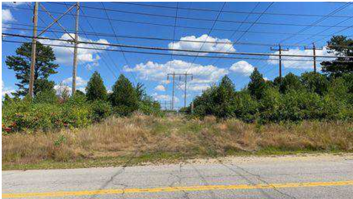
Photo 31. Montgomery Street crossing, viewing east. Str. 66 visible in distance.
