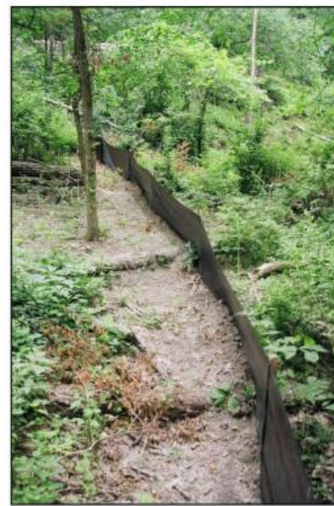
Best Management Practice 5: Silt Fence
