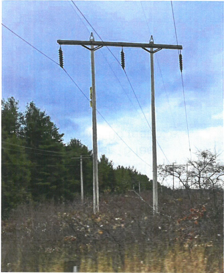
Example of existing structure to be removed
