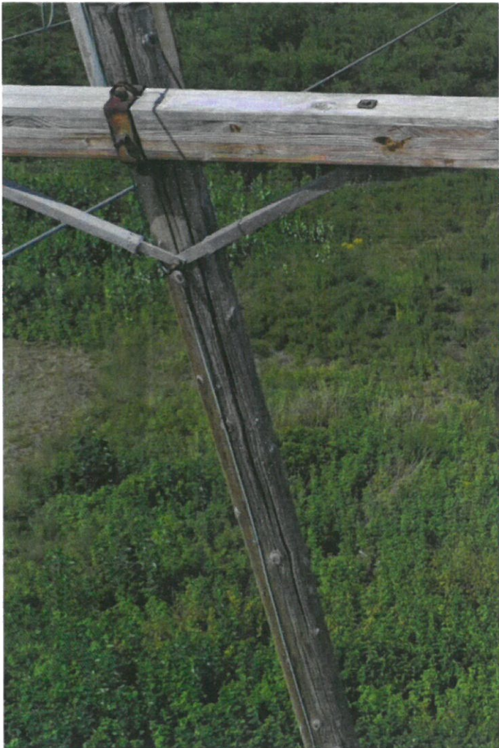
Cracked Pole
